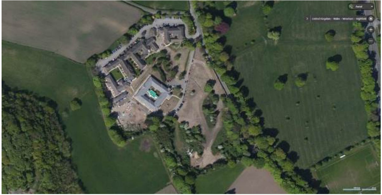
Site aerial (pre-laundry block construction)
