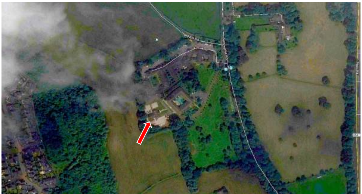
Site Aerial (with laundry block constructed - arrowed)
