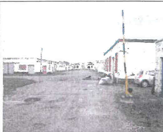
26. View looking northwards across site
