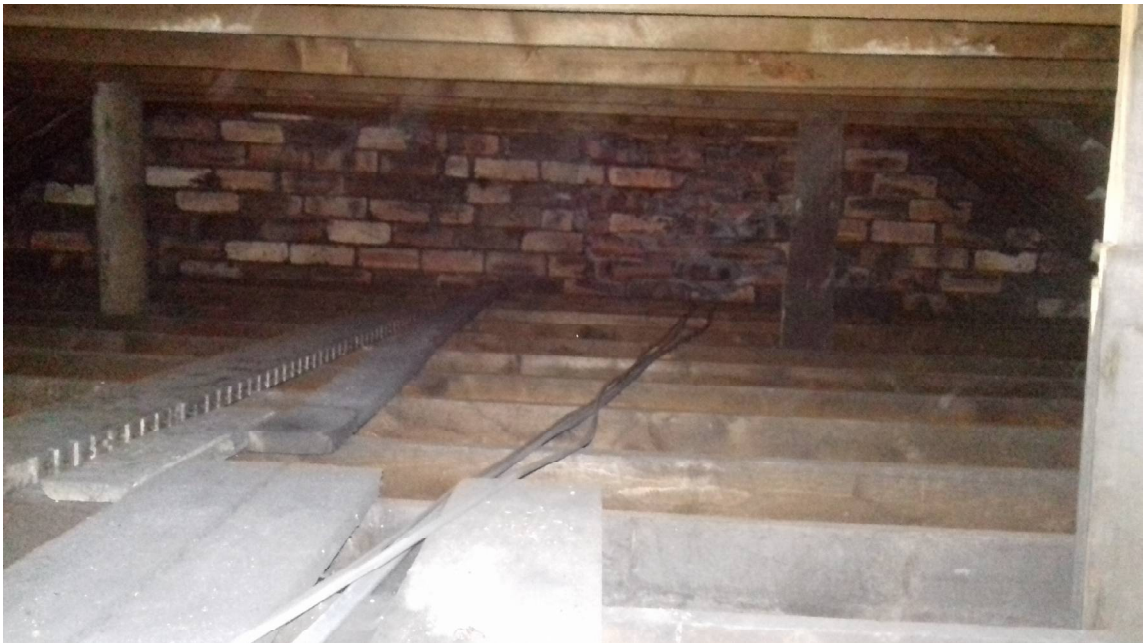
Truss roof construct of B1
