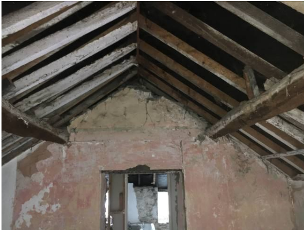
Photo 7: Internal view of house - upper room.
