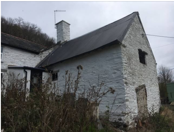
Photo 3: Hay Barn viewed from the west.
