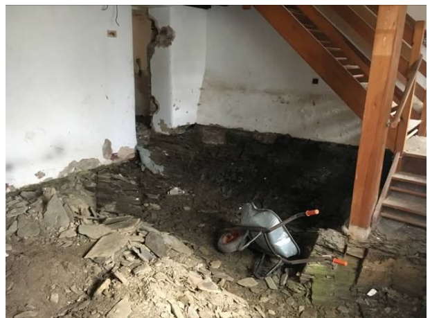
Photo 6: Internal view of house - ground floor.
