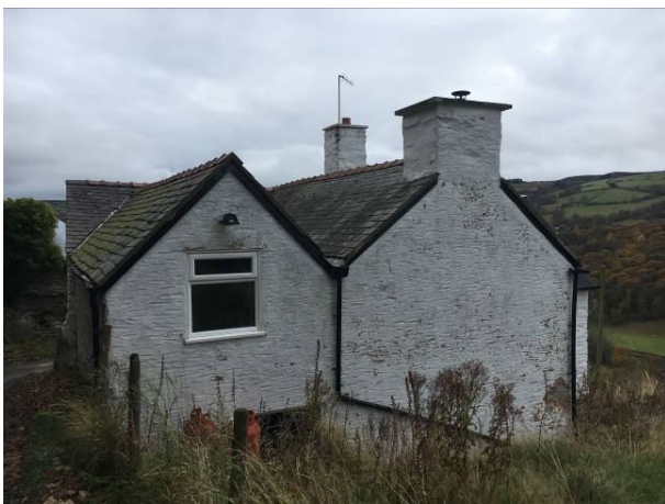
Photo 5: House viewed from the north.
