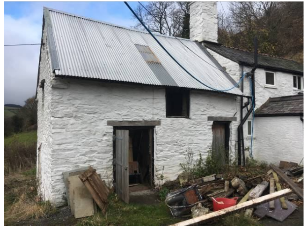
Photo 2: Hay barn viewed from the south east..
