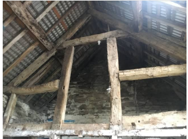
Photo 8: Internal view of hay barn.
