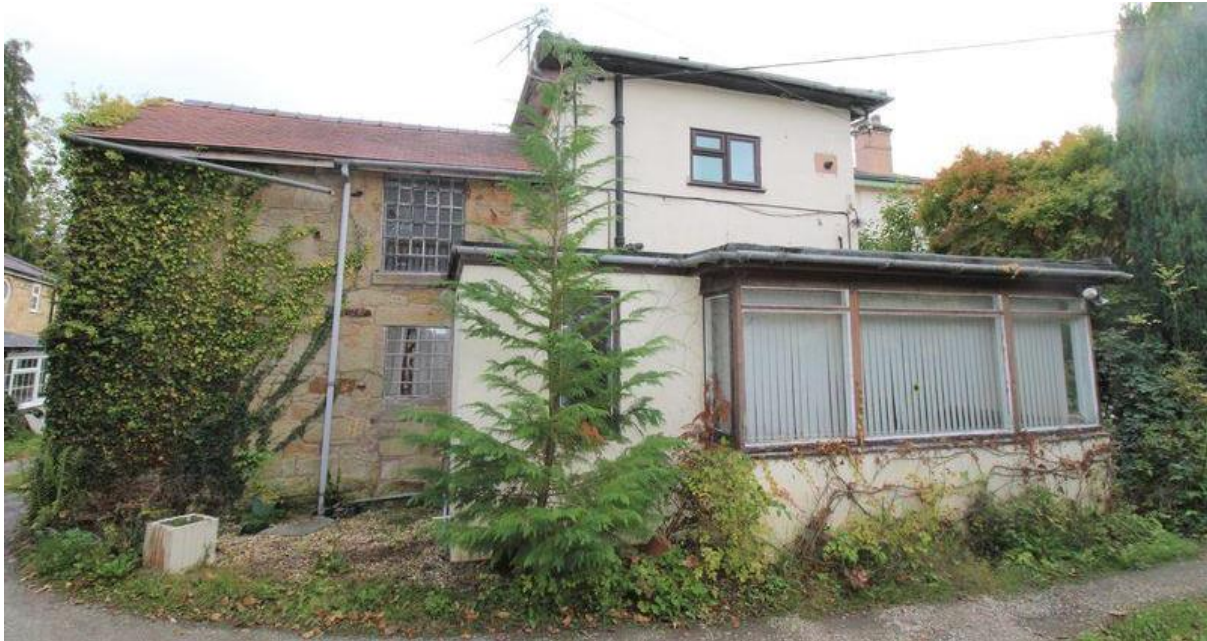
Image of rear elevation illustrating the original rendered service wing, adjoining stone extension and rear conservatory (21.01.2019)
