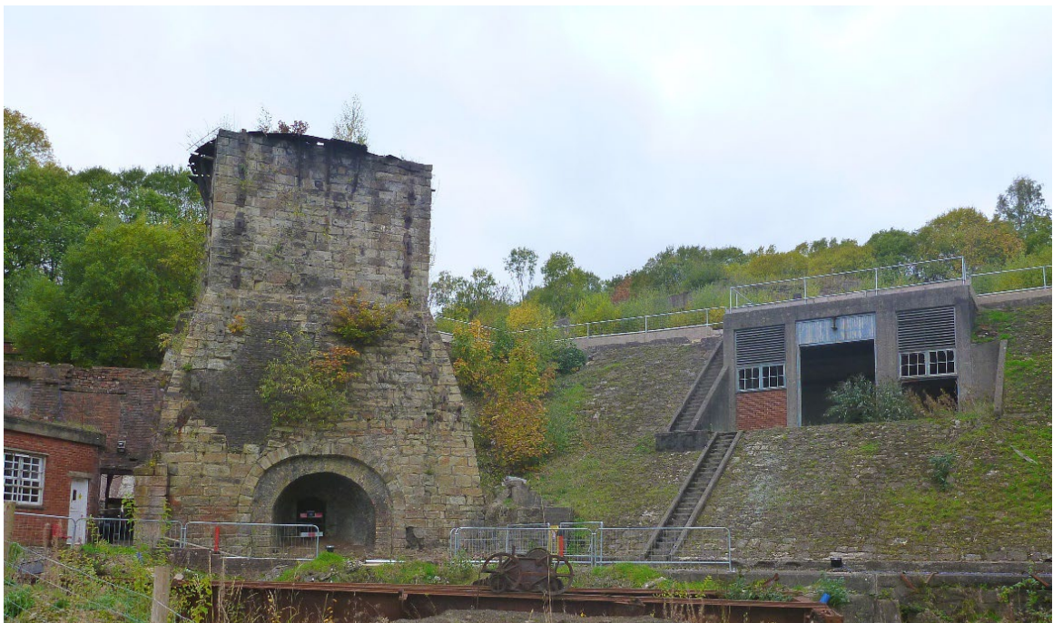
Figure 2: View west towards No.1 Furnace as it stands today
