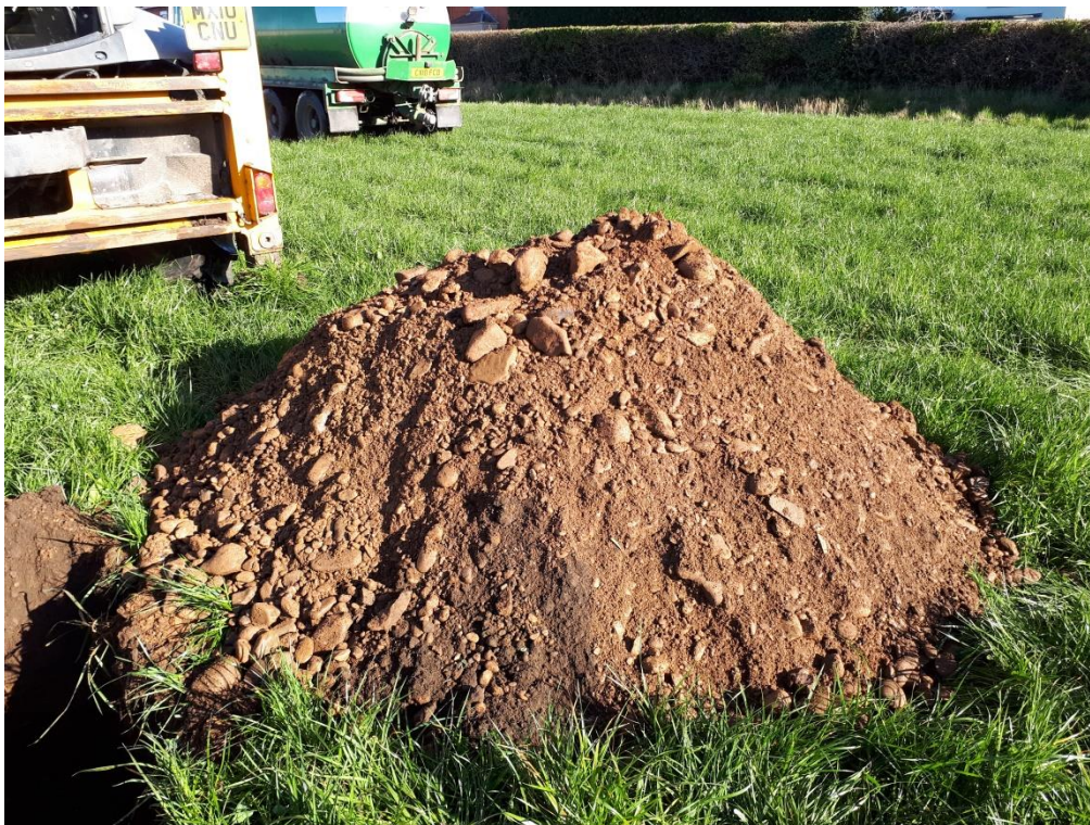
Trial Pit 01 - Arisings
