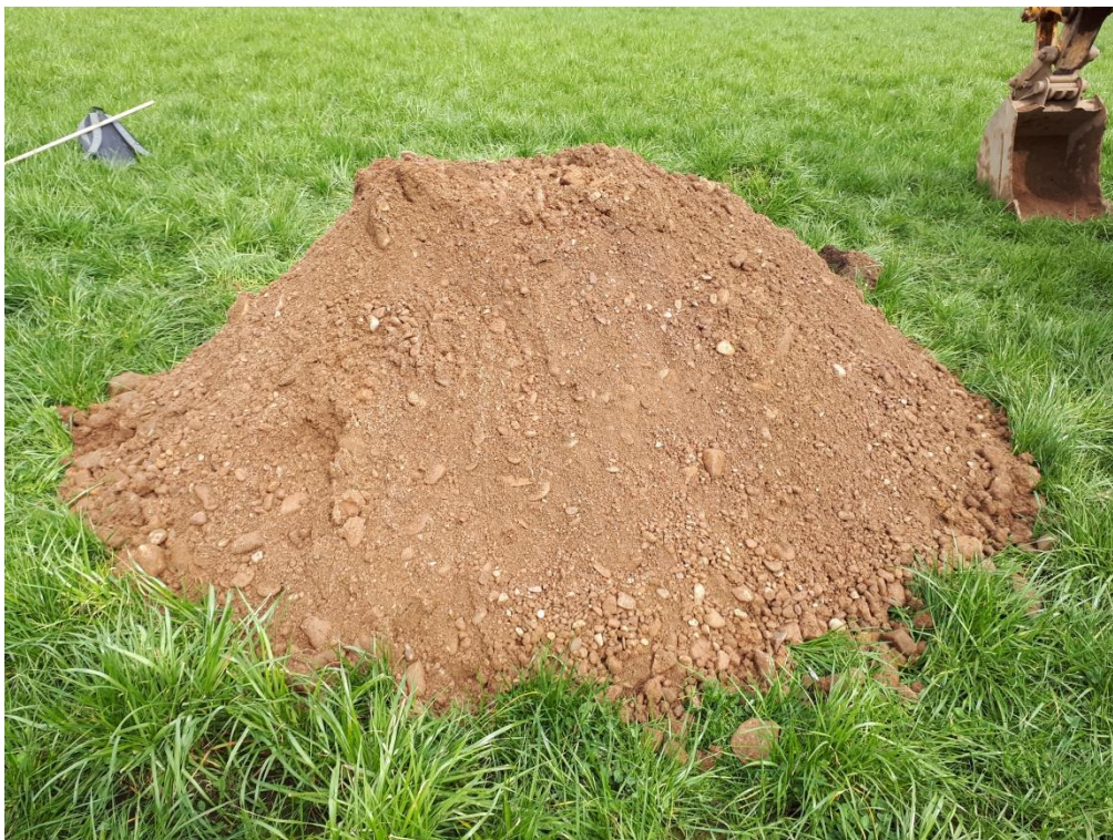
Trial Pit 10 – Arisings
