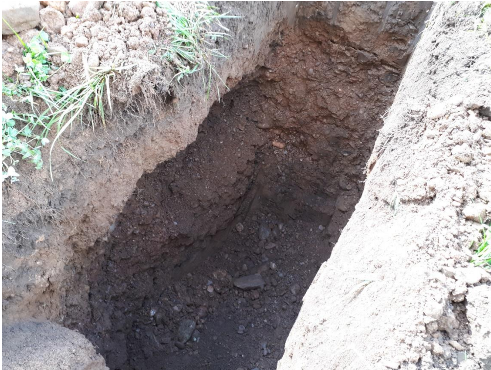
Trial Pit 11 – Pit Walls
