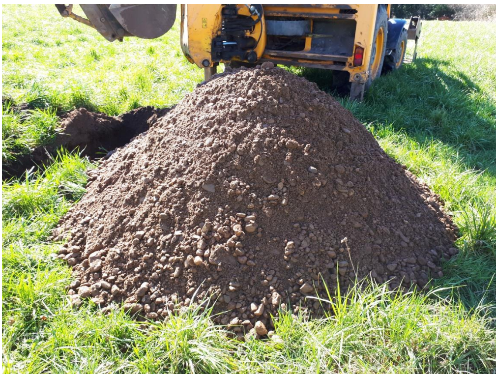
Trial Pit 02 - Arisings
