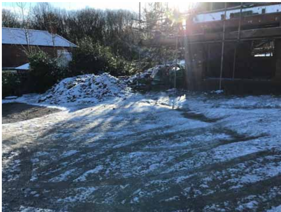
Stockpiles of excavated soil and construction materials at eastern boundary of the site
