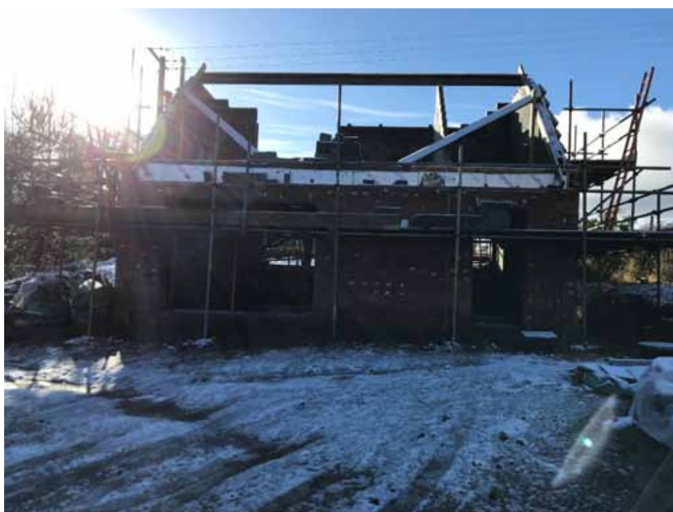
Existing structure on site (looking south-west towards read of site)
