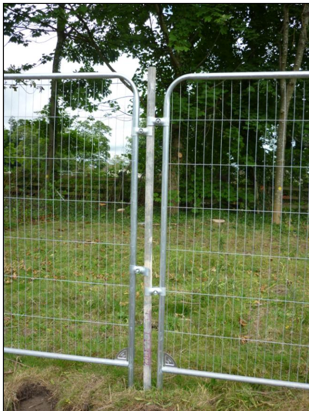
Tree Protective Fencing Specification
