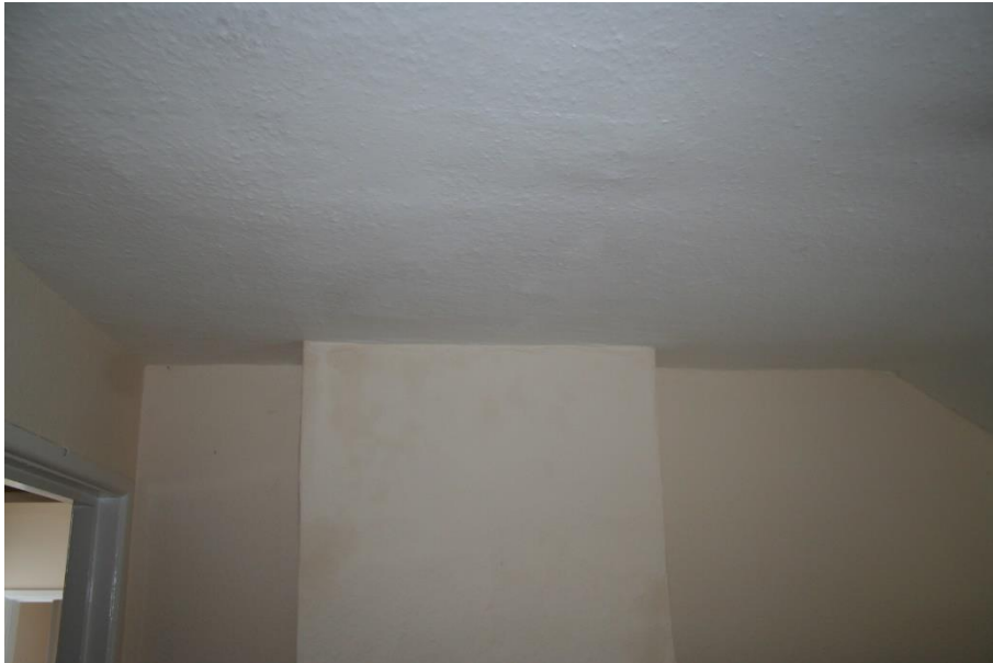
Figure 4.6: Internal assessment of the flat to the first floor
