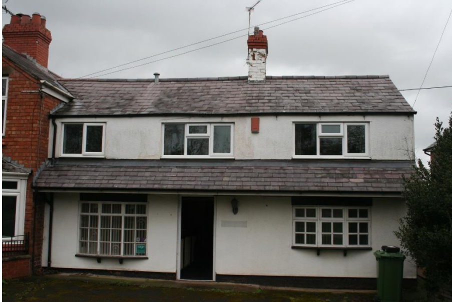
Figure 4.2: Photo of the front of the main building, showing sealed brickwork and slate tile roof and canopy.
