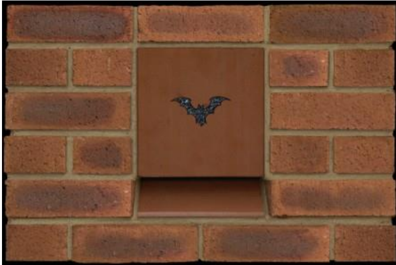
Figure 6.1. Integral bat box
