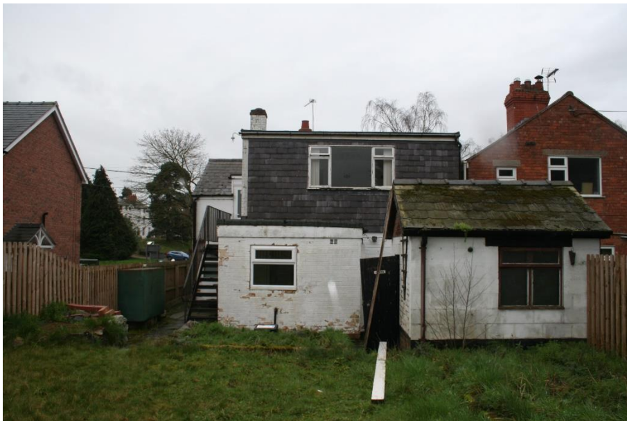
Figure 4.9: Photo of the north facing side of the outbuilding and main building, showing hanging tiles
