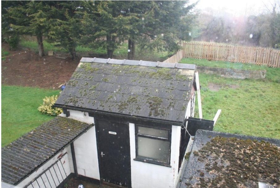
Figure 4.8: Aerial photo of the outbuilding used as an external toilet
