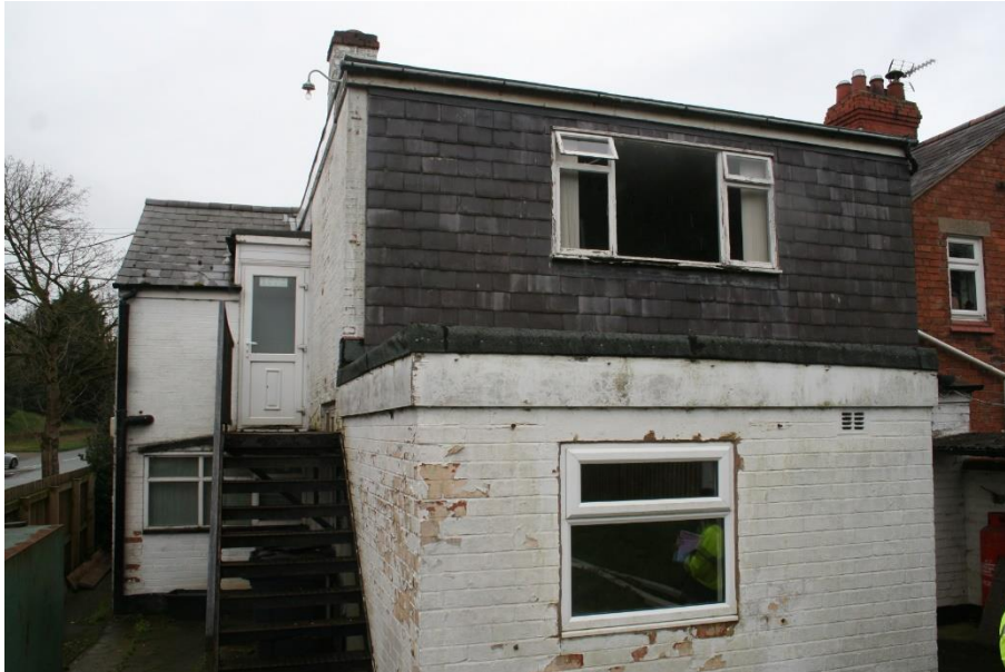
Figure 4.3: Photo of the rear of the main building, showing hanging tiles and slate tile roof and well mortared brickwork
