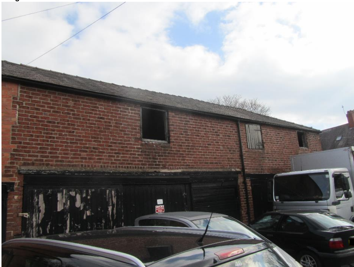
Image 3.26 Northern elevation of B3
