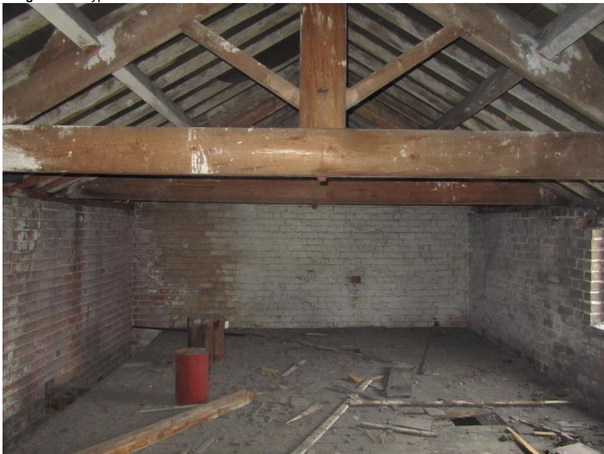
Image 3.27 A typical view within the first-floor level of B3
