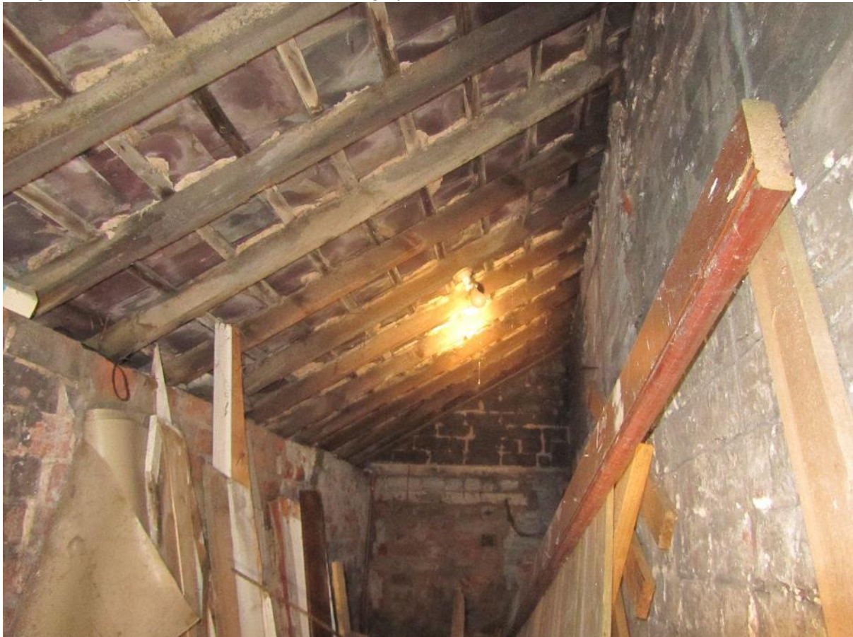
Image 3.24 A typical view inside B2, showing open/ unlined roof
