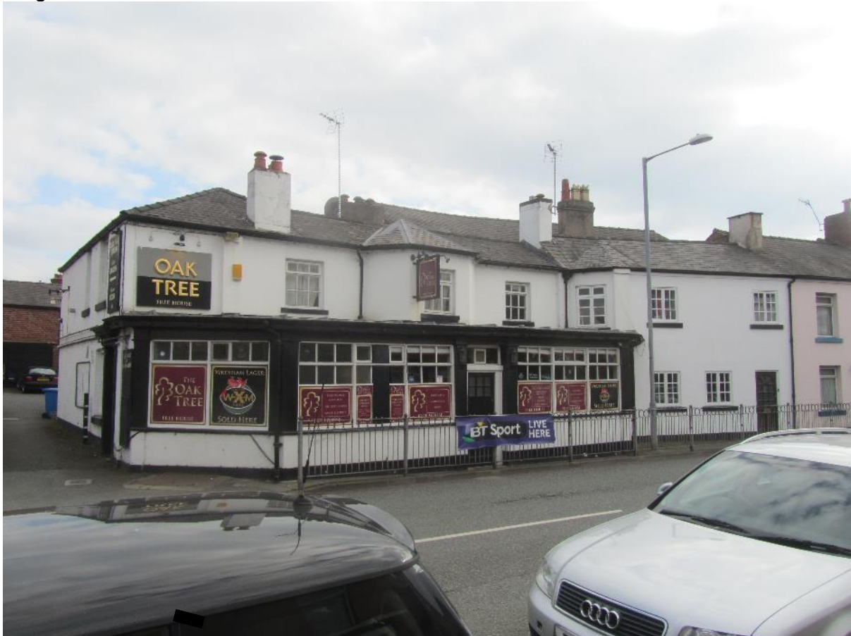
Image 3.4 Northern elevation of B1
