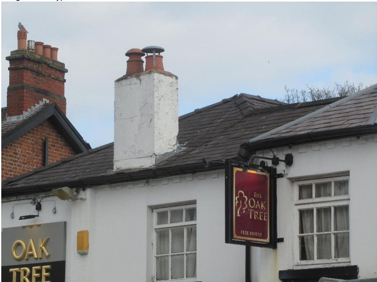
Image 3.17 A typical view of the roof of B1
