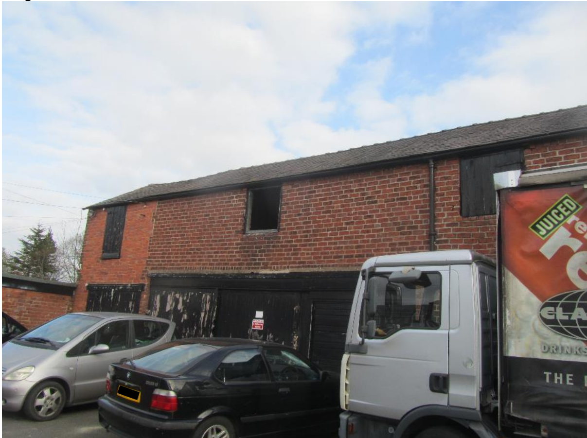
Image 3.7 Northern elevation of B3
