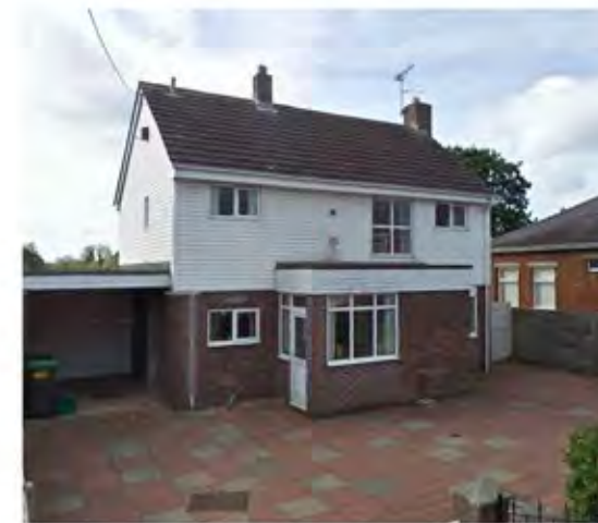
projecting porches / cladding / flat roofing
