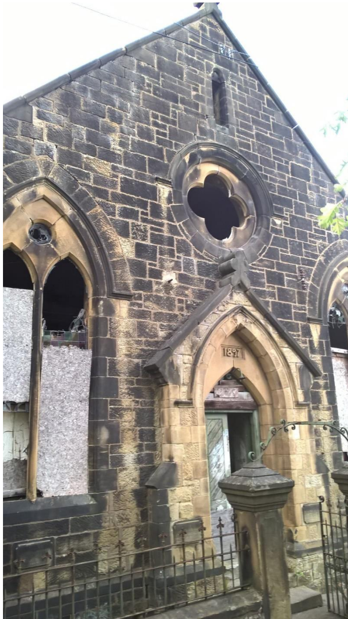
Figure 3 – south side of the chapel
