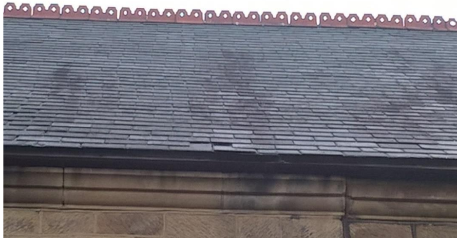
Figure 7 – The roof from the east side
