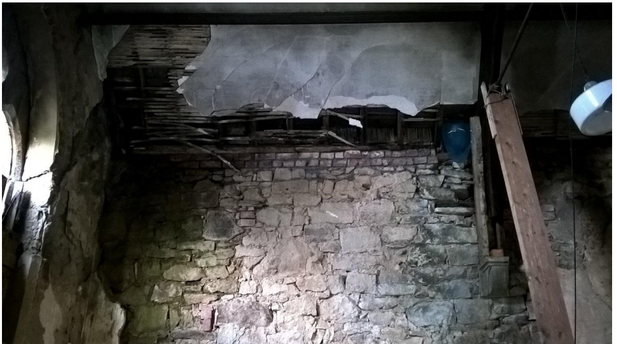
Figure 11 – Lathe and plaster construction of the ceiling
