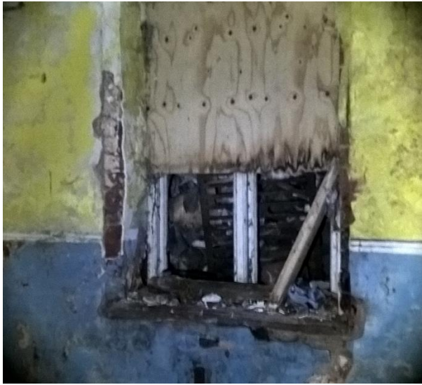
Figure 12 – Window to the north of the basement
