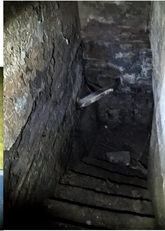
Figure 13 – Stairs to the coal store/heating room
