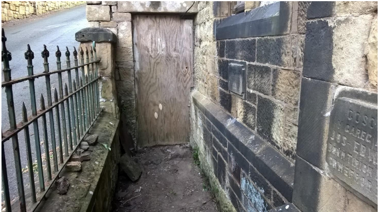
Figure 4 – door to the west of the main entrance
