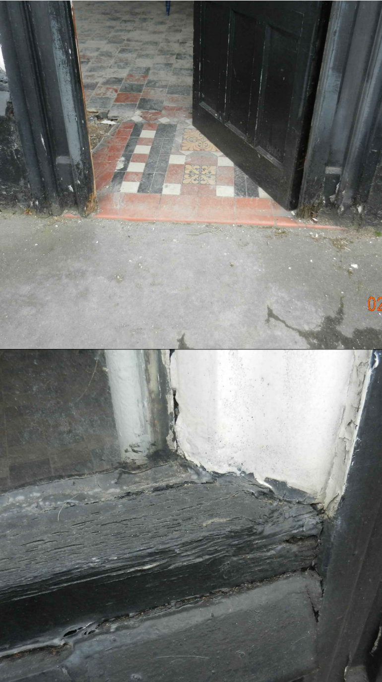
Images showing existing condition of shop front
