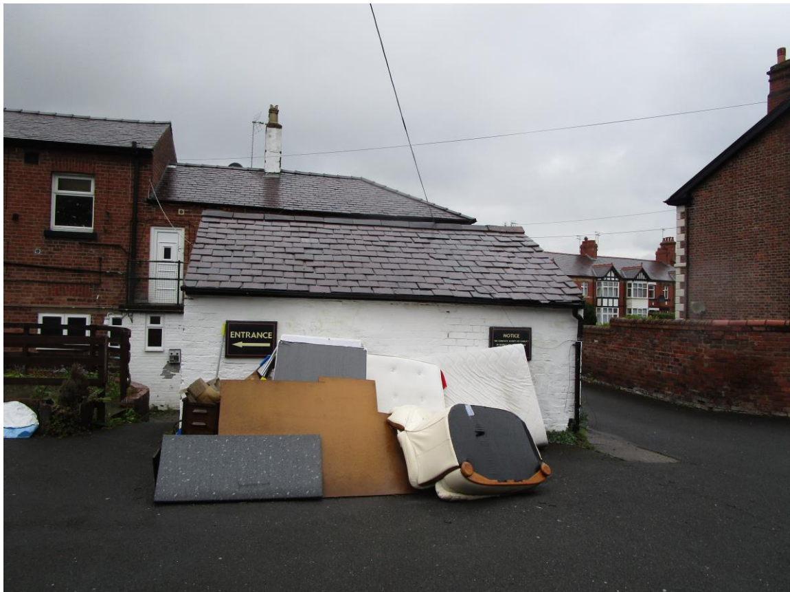
Photograph 11 – detached out building adjacent to public house
