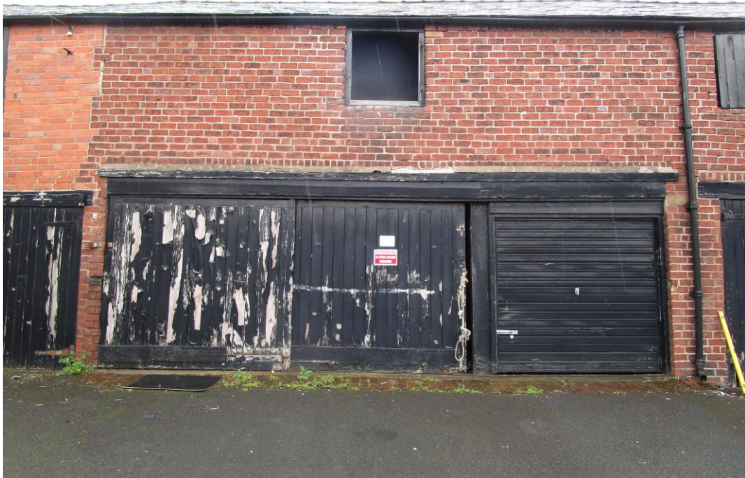
Photograph 5 – showing dominant opening to front elevation with non-original supporting column
