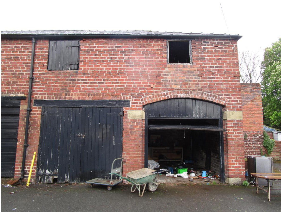
Photograph 6 – showing brick arch to right-hand opening
