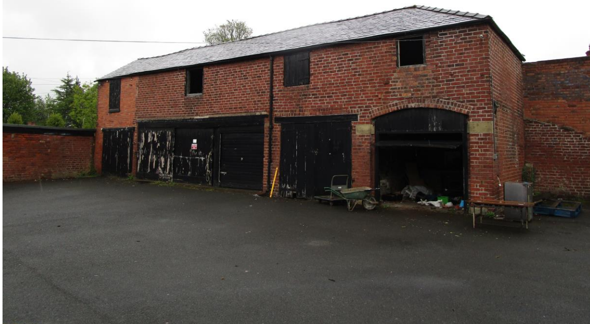
Photograph 1 – front elevation of former stable block
