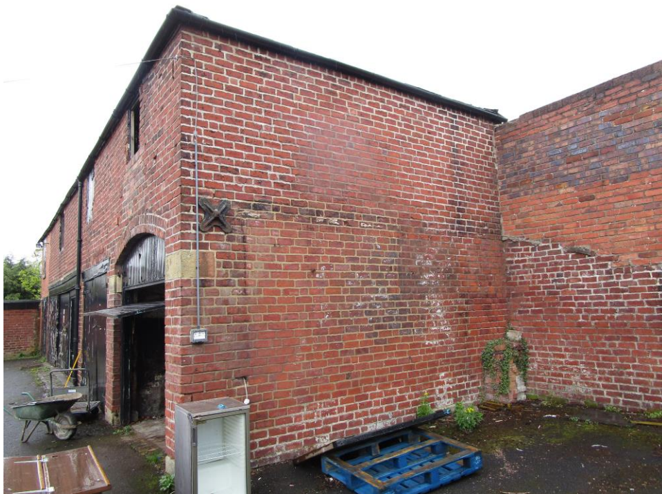
Photograph 8 – showing right-hand elevation
