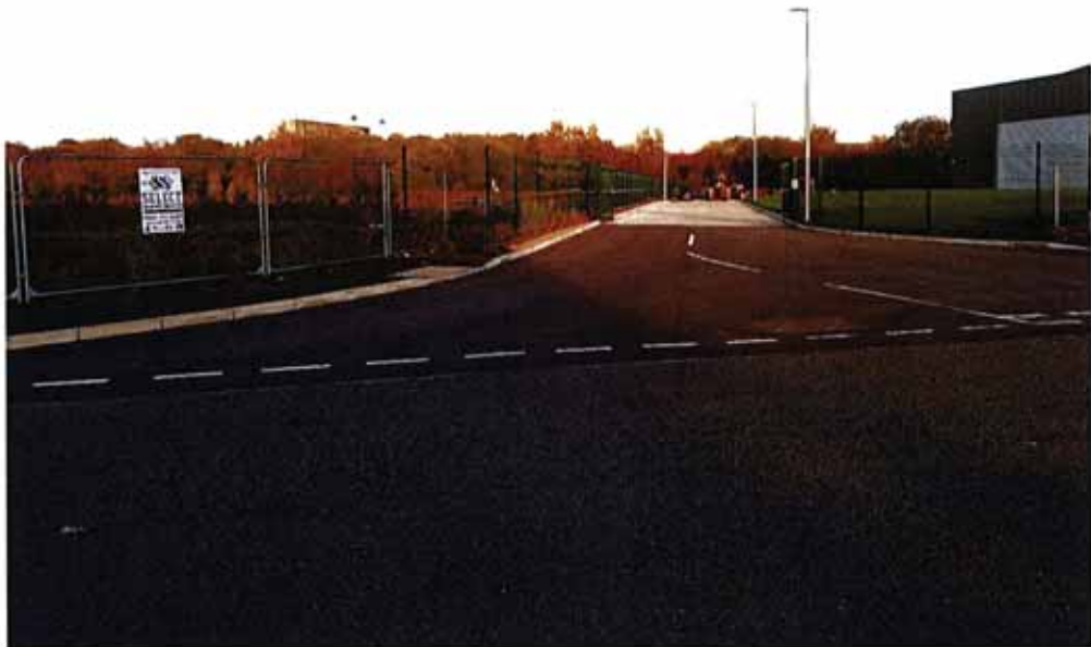
Photograph 12 Access road on southern site boundary
