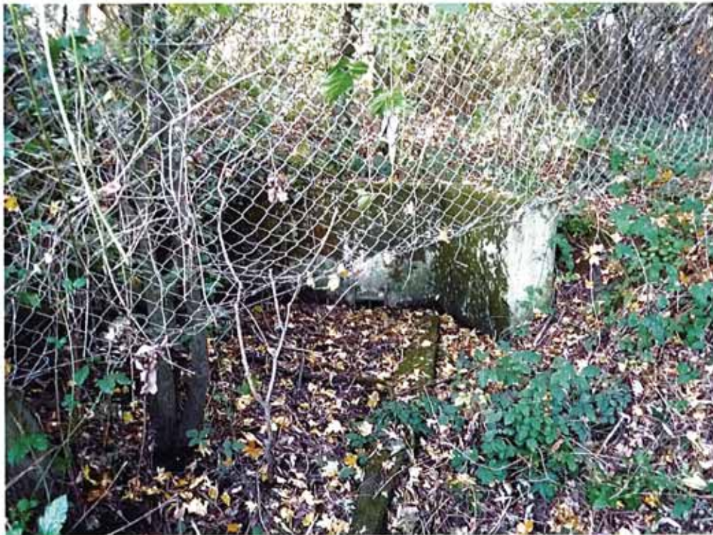
Photograph 14 Concrete headwall in northern corner of site
