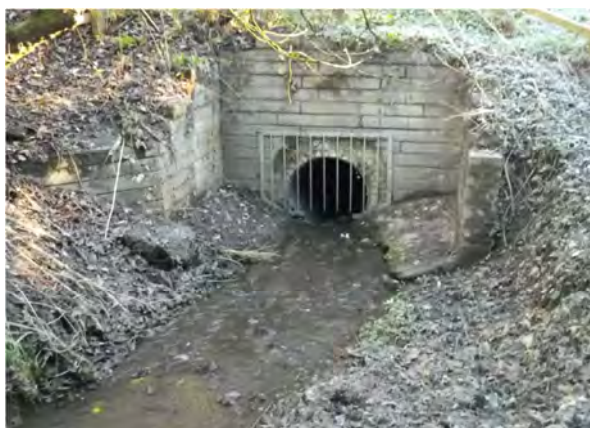
3. Culvert Inlet – Rhos_0362 ESTRY Unit: Circular Culvert
