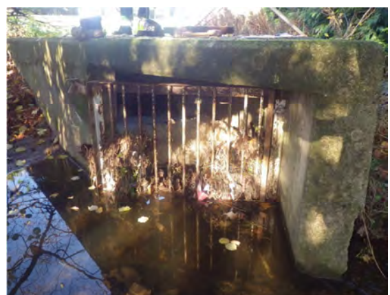
2. Culvert Inlet – Rhos_1059 ESTRY Unit: Circular Culvert
