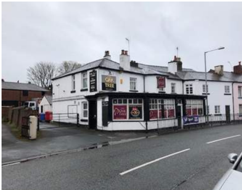
Fig 1 Oak Tree, Ruabon Road, Wrexham
