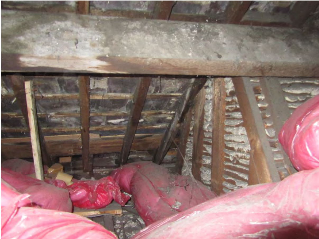
Image 3.20 A typical view within a loft void inside B1, showing unlined roof
