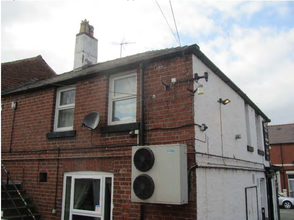
Image 3.16 Southeast corner of B1, showing general construction
