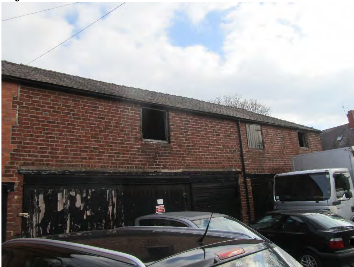
Image 3.26 Northern elevation of B3
