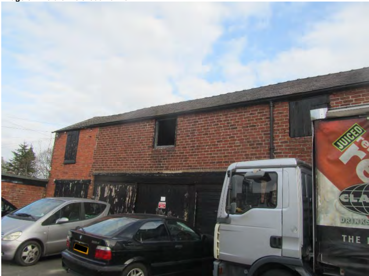
Image 3.7 Northern elevation of B3
