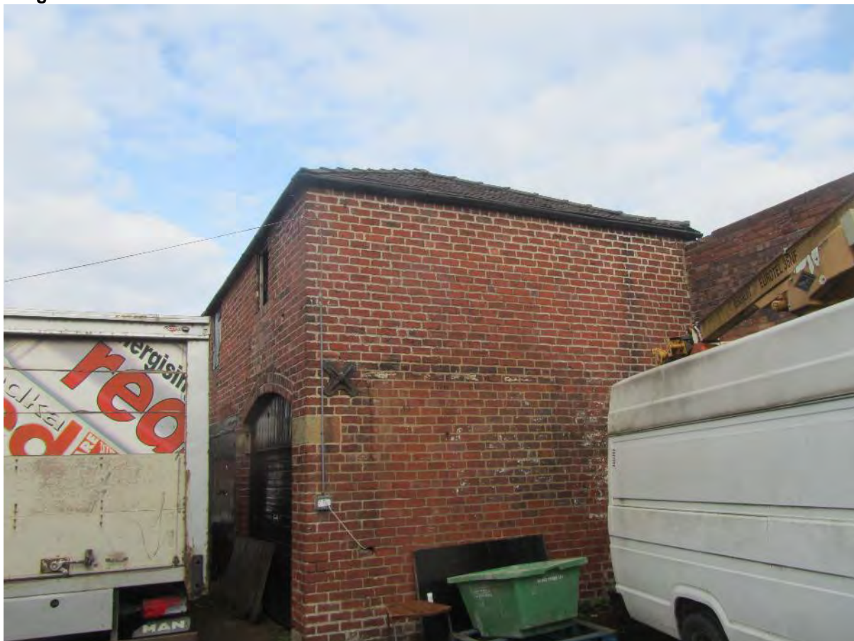
Image 3.25 Western elevation of B3
