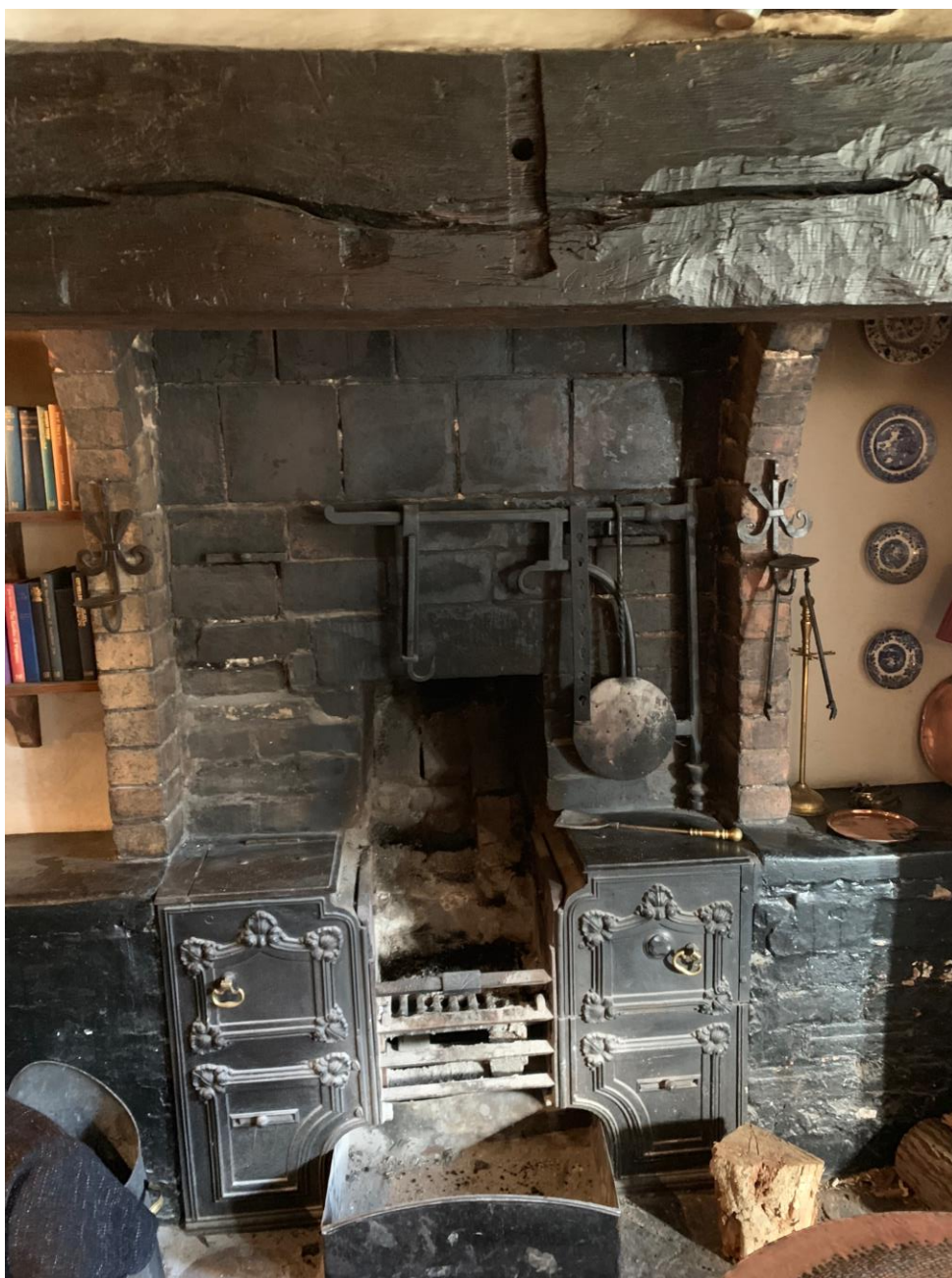
Figure 4- range and bressumer. Post-1870 range with slow combustion grate set low on the hearth, and long and narrow opening.
