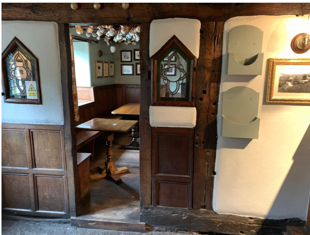
Figure 5- dividing wall, east building
