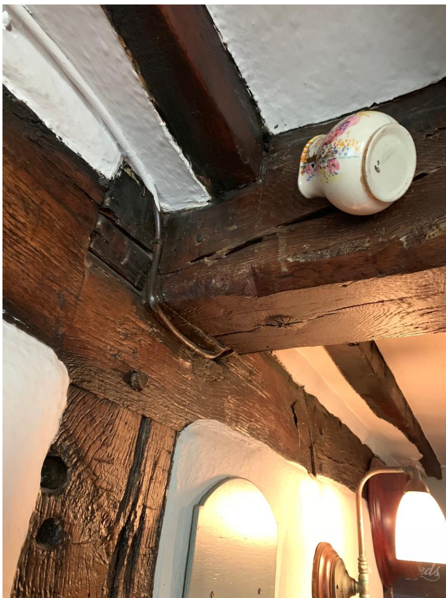
Figure 8- ceiling beam with simple chamfered stops. Timber packing to the lateral tie-beam illustrates re-use and re-positioned timbers.
