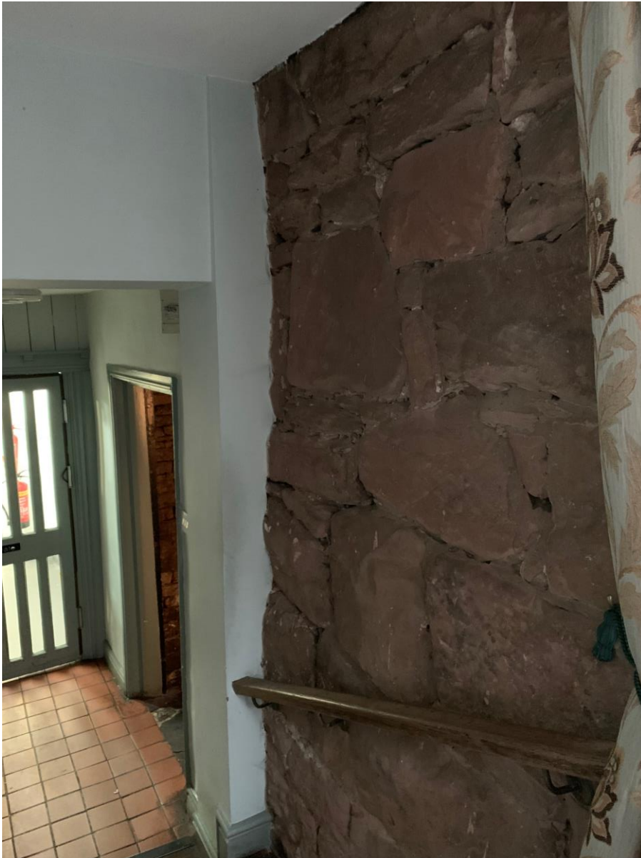
Figure 17- part of northern return wall of north exterior wall, in western building, now internalised.
