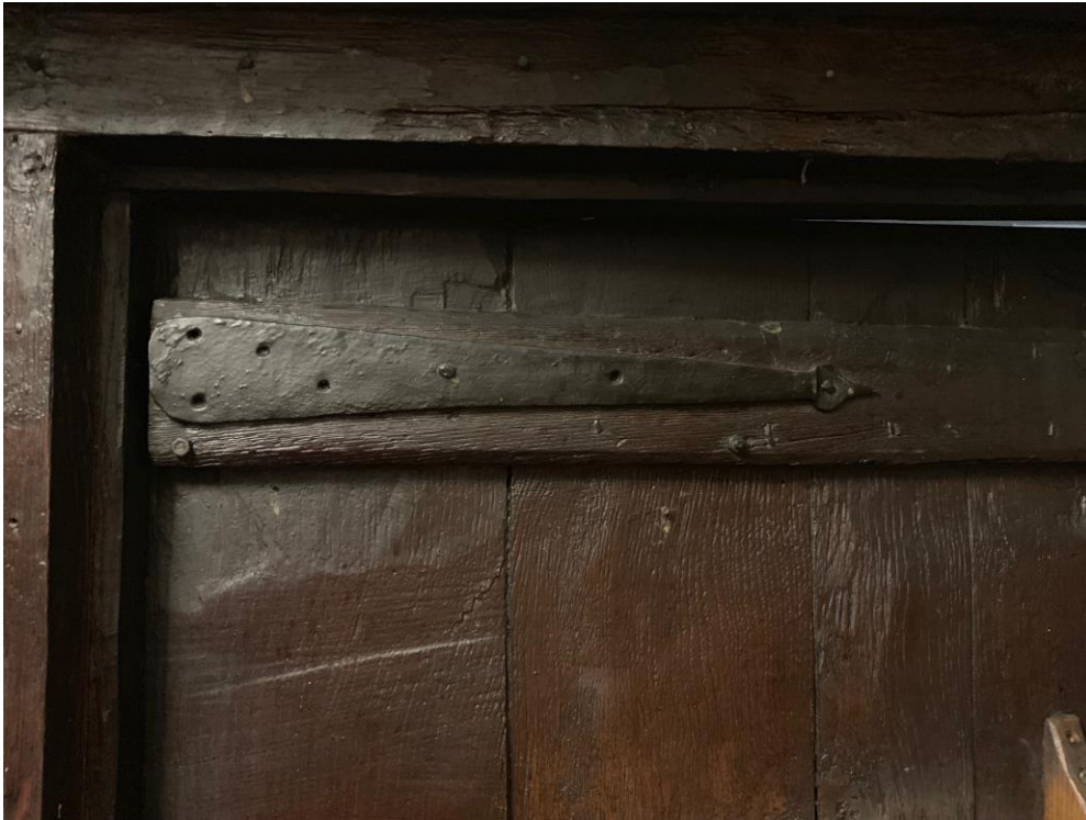
Figure 3- door showing detail of strap hinge
