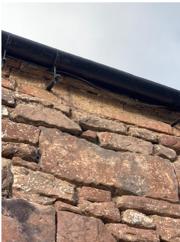
Figure 23- brick coursing at eaves level, west building.
