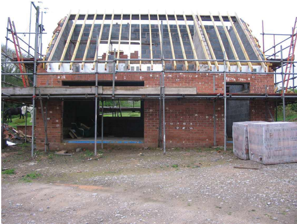
7) The New Garage Building
