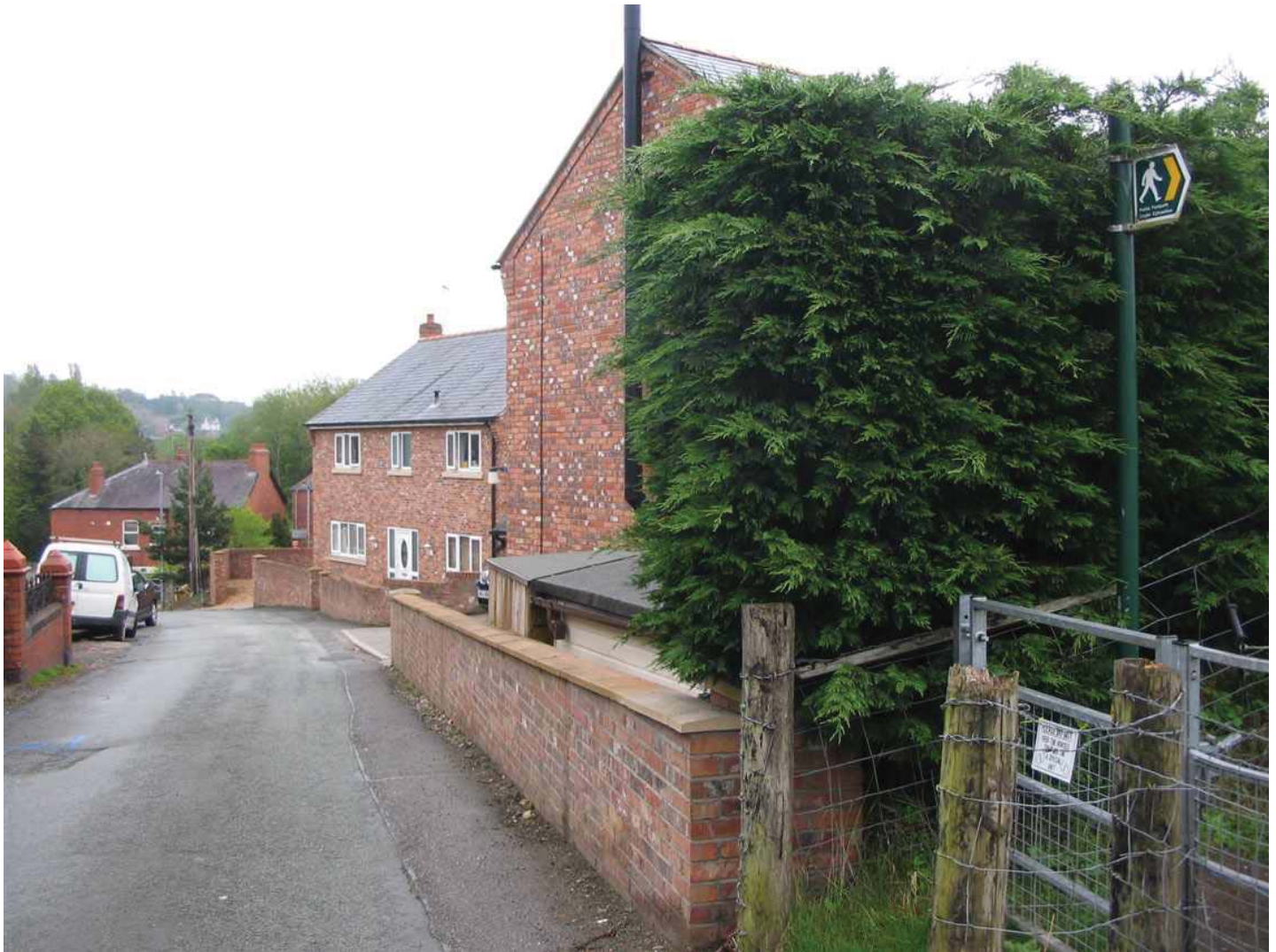
2) View down Tower Hill from the site of a Former Rock Cutting - 1st May 2019
