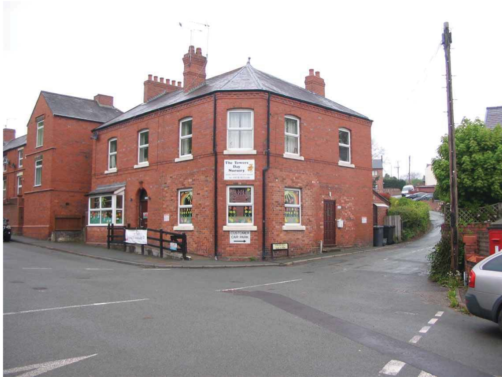
1) The Towers Day Nursery off Llangollen Road
