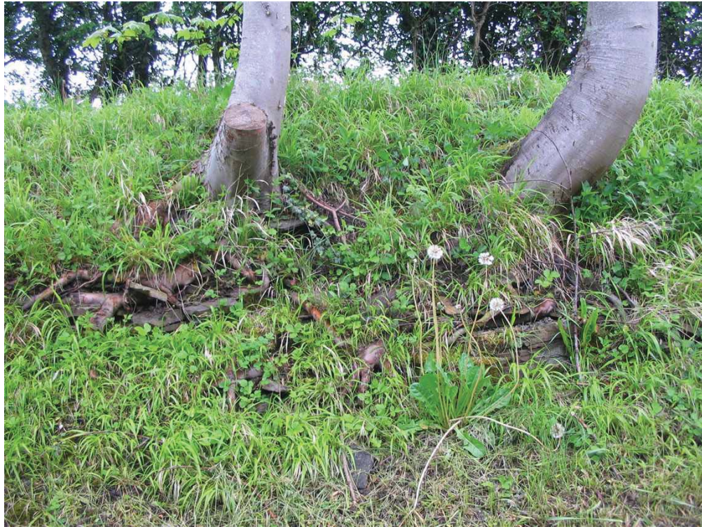
7) Rock Outcrop below Trees along Llangollen Road
