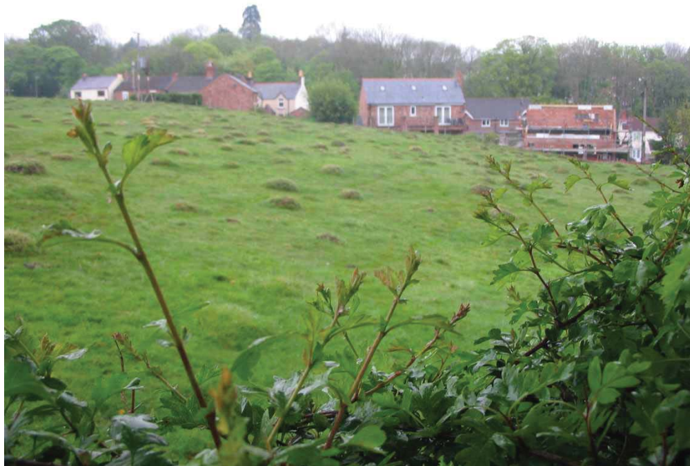
12) Hafan, Sara and the New Building at the Site viewed from Llangollen Road
