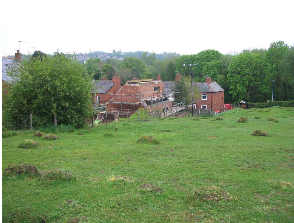
13) New Building at the Site viewed from the North-west
