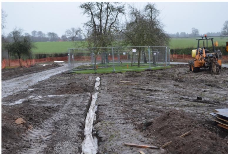
Photo 5. T56 drainage trench
