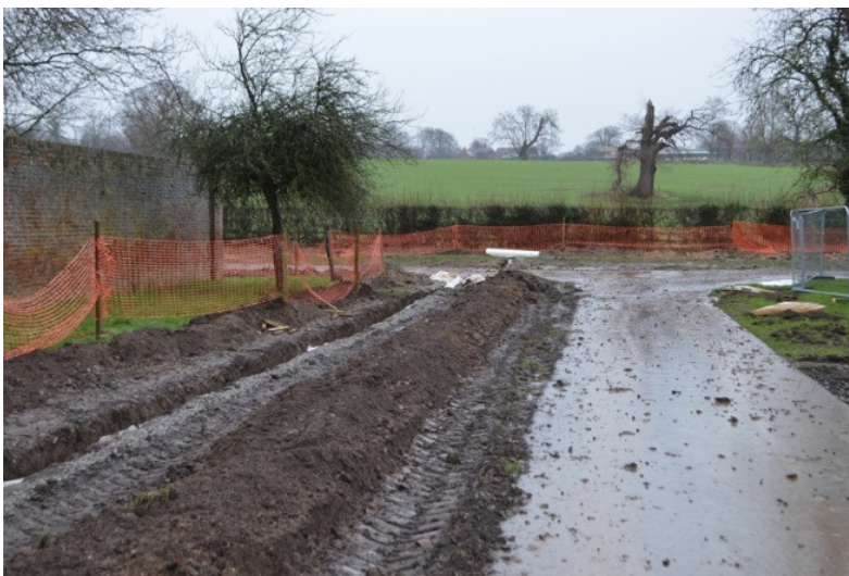
Photo 3. T13 drainage trench
