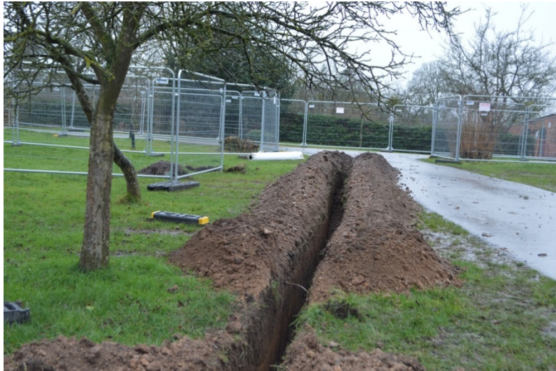
Photo 4. T28 drainage trench
