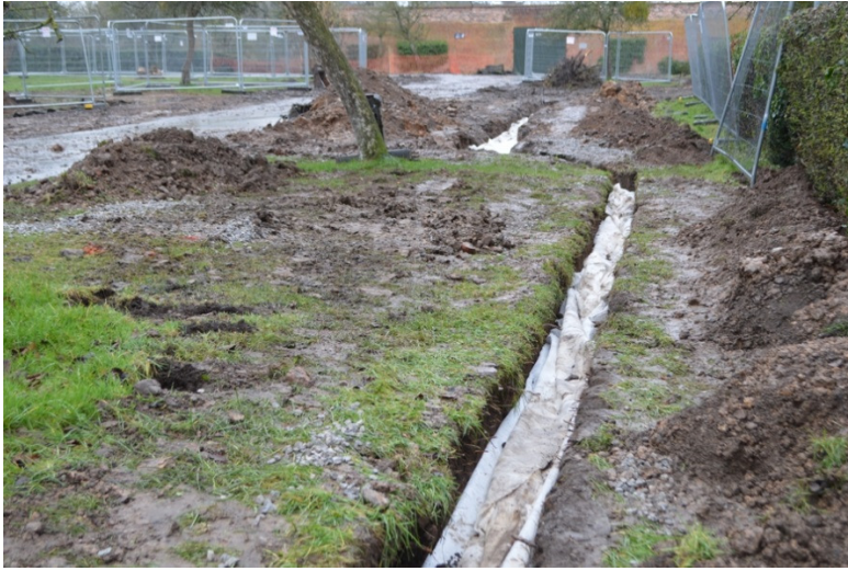
Photo 1. T114 drainage trench
