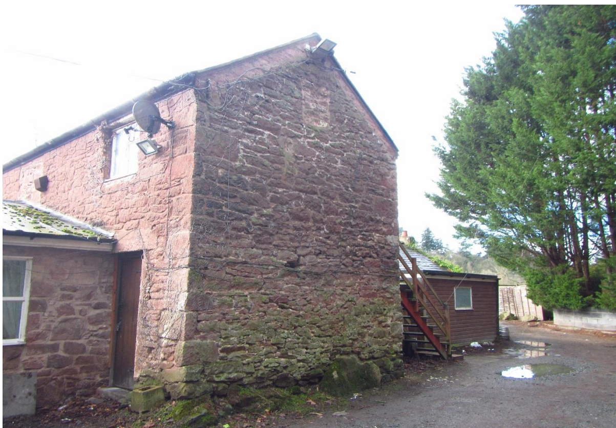
Photo 7. Rear (north) gable end of Building B.
