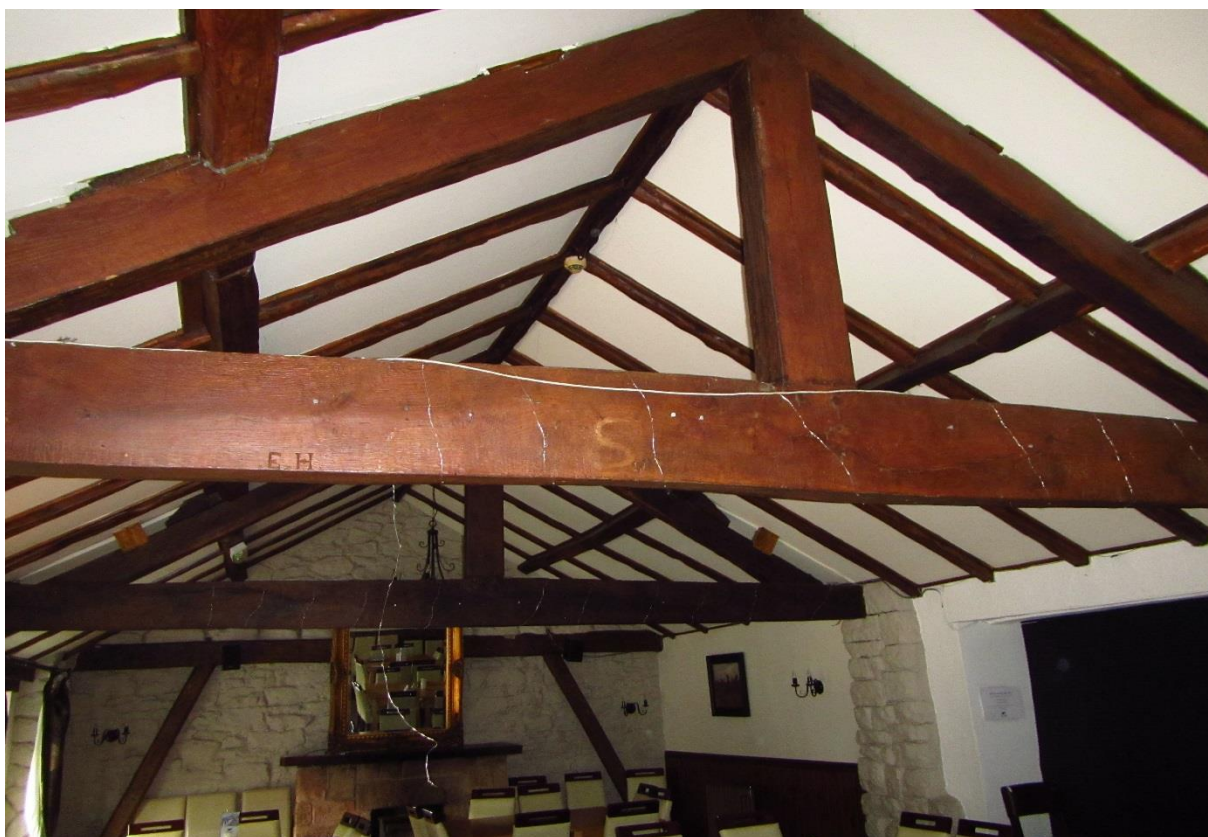
Photo 12. Interior of Building C.
