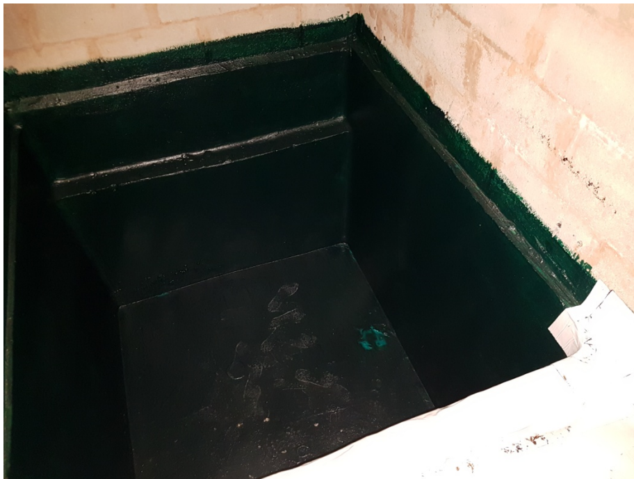
Photograph 4: Liquid Corden EPS Liquid Gas Barrier within the lift pit.
