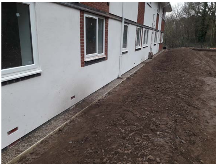
Photograph 2: Replaced sub floor air vents and newly installed air vents within cavity wall.
