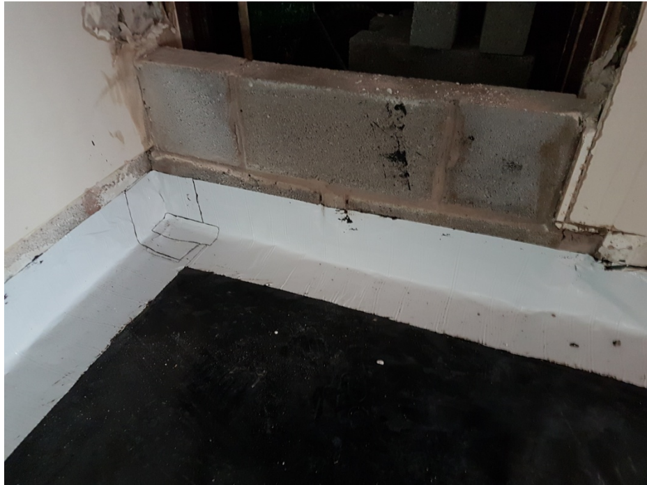
Photograph 3: Corner detail with self adhesive membrane.
