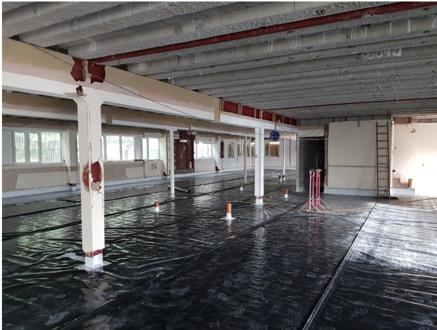
Photograph 2: General photograph of the Evolution VOC membrane across the existing ground floor.
