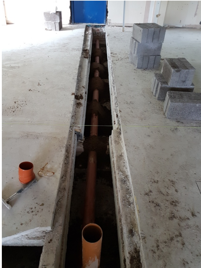
Photograph 1: Trench to install new drainage, showing the existing suspended floor slab and subfloor void.
