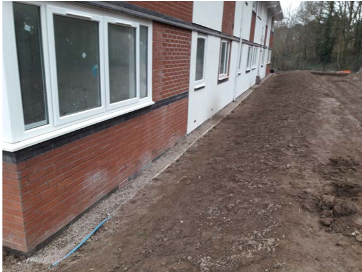
Photograph 1: Replaced sub floor air vents and newly installed air vents within cavity wall.
