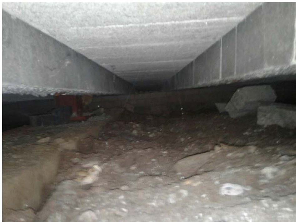
Photograph 3: Subfloor void (minimum 400mm) to allow subfloor ventilation (25.07.18).
