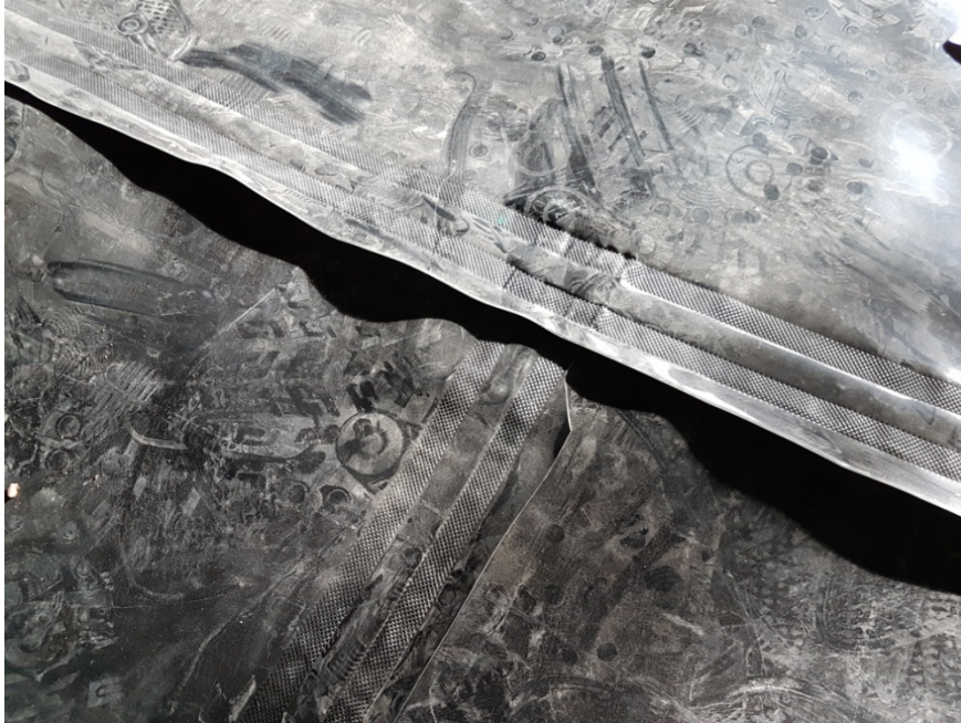
Photograph 1: Detail of welded joints and cut-out tab.
