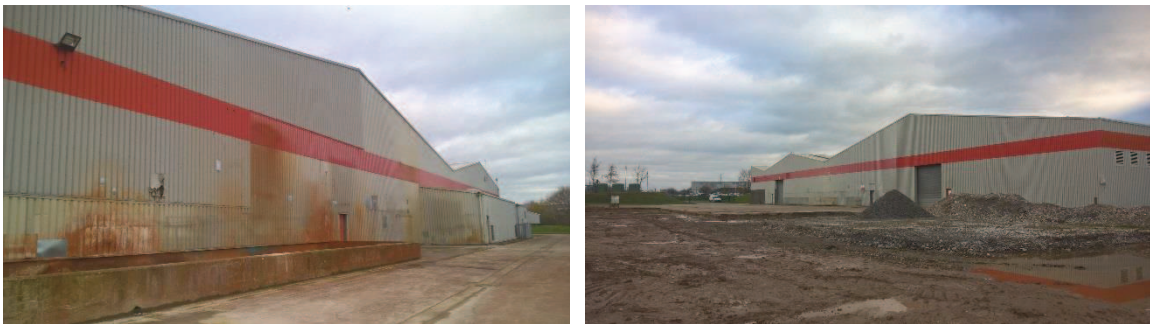
PHOTO 4.1 & 4.2. EASTERN AND WESTERN SIDES OF THE FACTORY BUILDING
