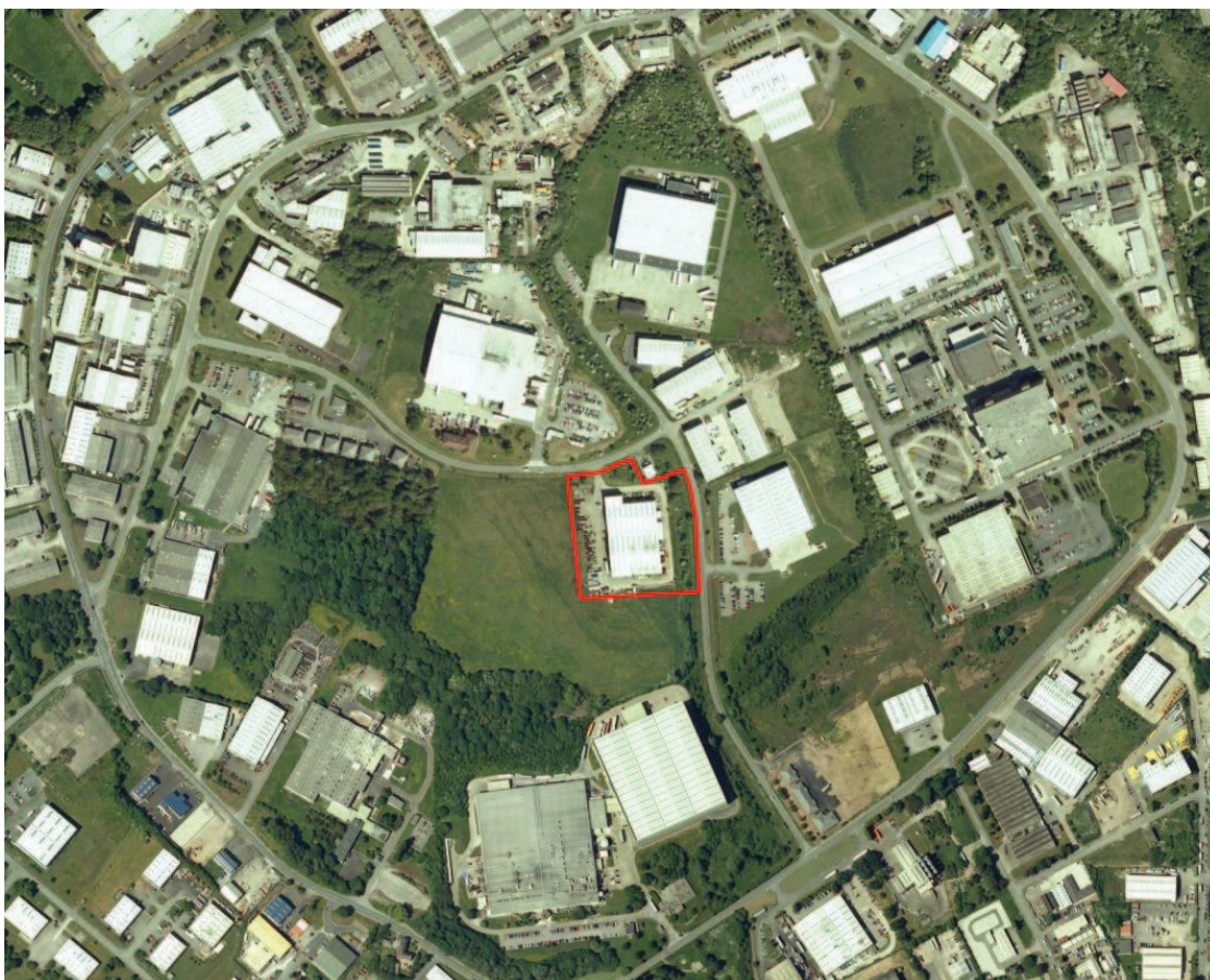
FIGURE 2.1. SITE BOUNDARY AND SURVEY AREA SHOWN IN RED. (THIS IMAGE WAS TAKEN PRIOR TO 2017 AND DOES NOT ACCURATELY REPRESENT WHAT IS ON THE GROUND AT PRESENT) © GOOGLE 2017.
