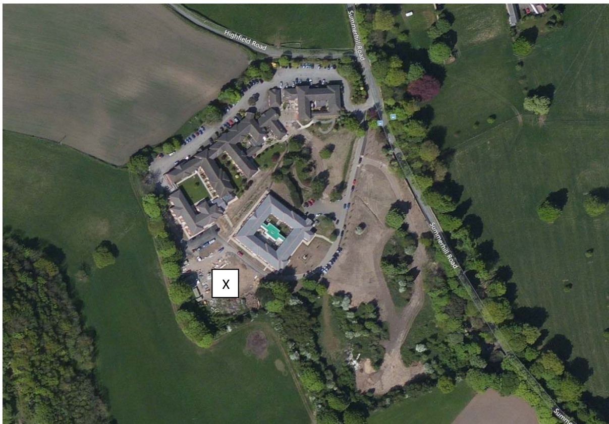
Aerial of site before construction of the laundry block at 'X'
