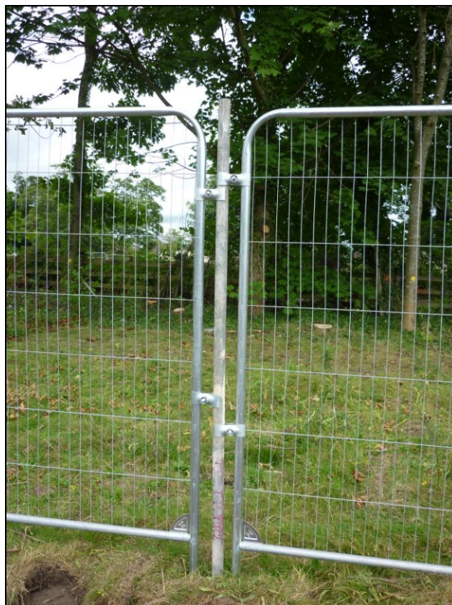
Tree Protective Fencing Specification
