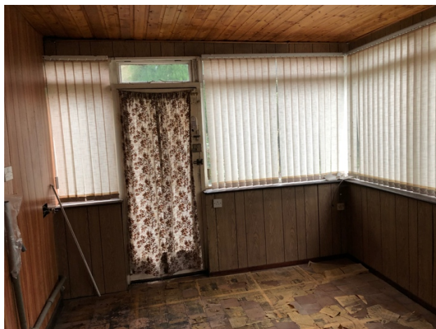
Internal image of existing flat roof conservatory:
