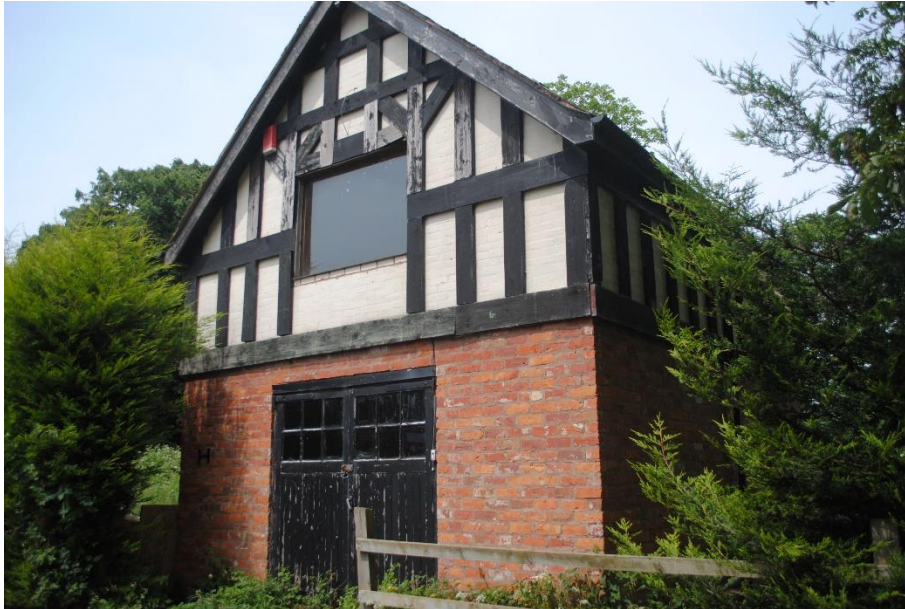
Figure 2: Building from the drive
