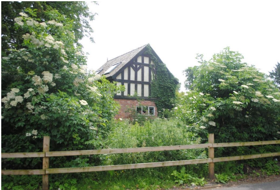
Figure 5: Site from the road
