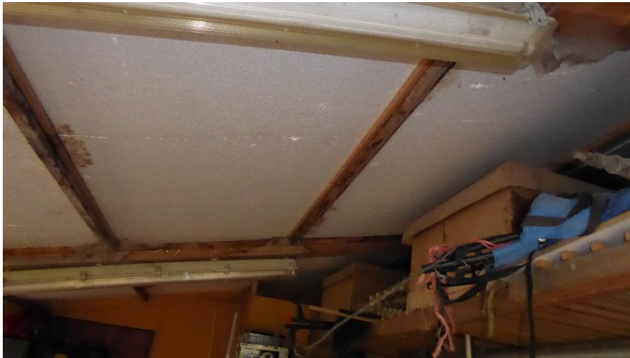
Figure 9. Inside the lean-to
