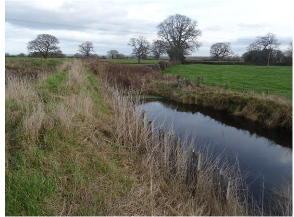
P19: Attenuation pond and bunds, looking NE
