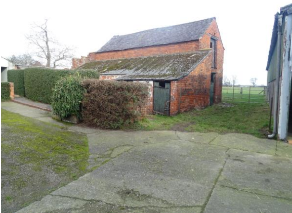
P14: NW yard area, looking N
