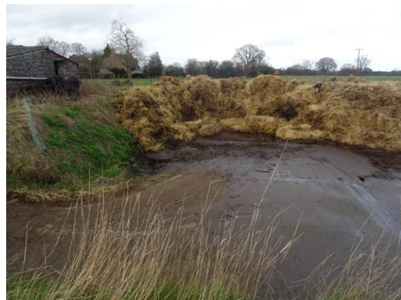
P3: Slurry lagoon adjacent to Pond 1, looking NW
