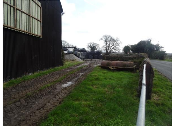
P7: SW yard area, looking E
