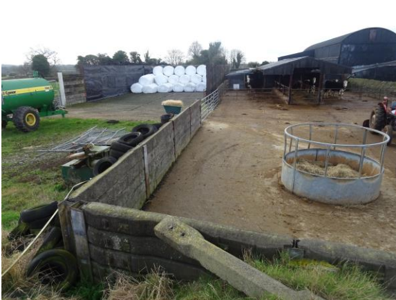
P10: NE yard area, looking SSW
