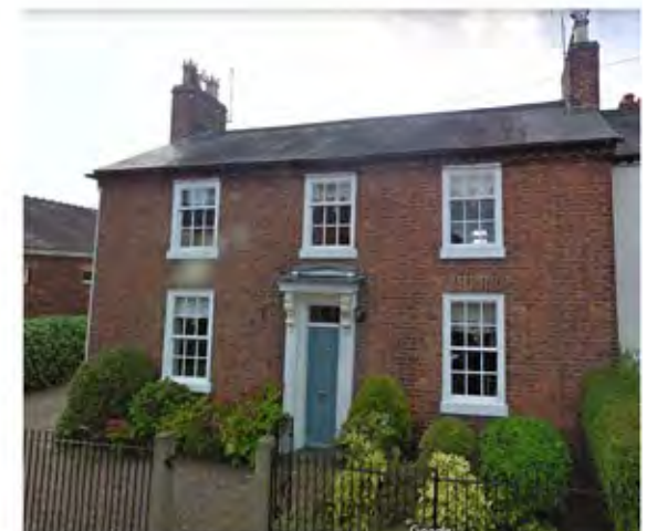
brick window heads / timber sash / shallow roof pitch / Georgian Architecture
