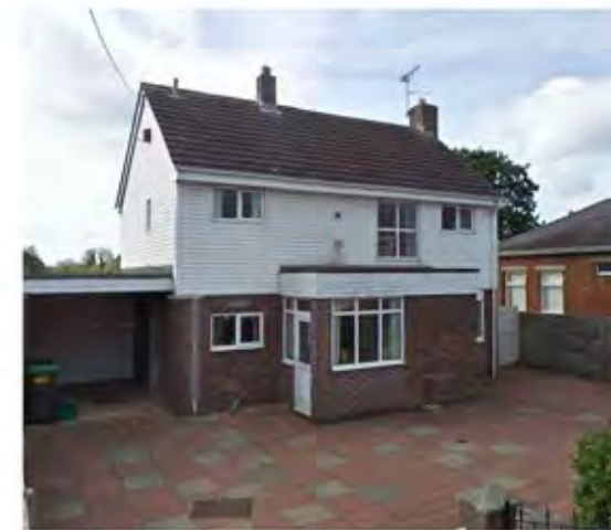
projecting porches / cladding / flat roofing
