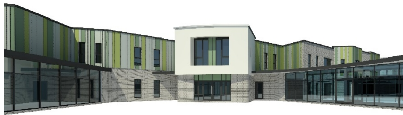
Fig 24: Materials study, viewed across central landscaped courtyard, illustrating:
