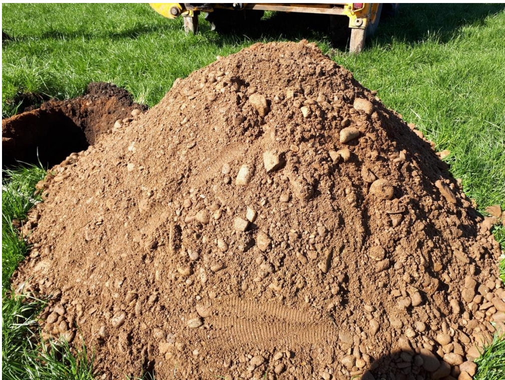
Trial Pit 03 - Arisings
