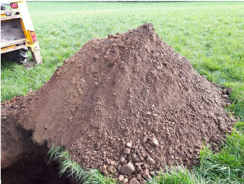
Trial Pit 07 – Arisings
