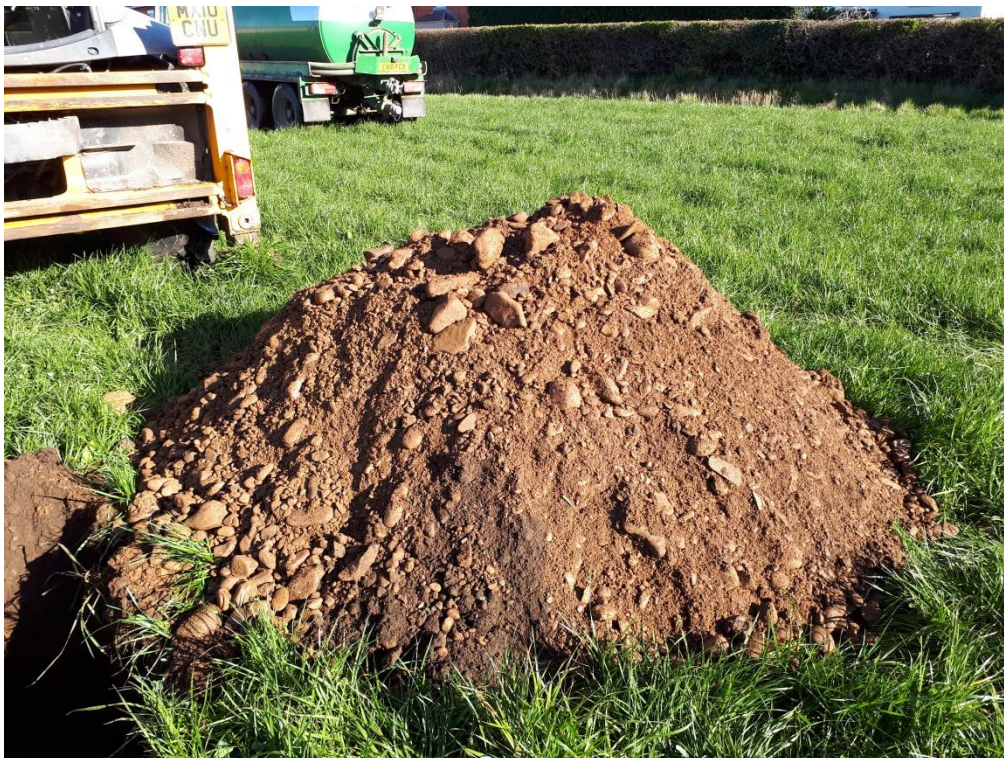
Trial Pit 01 - Arisings
