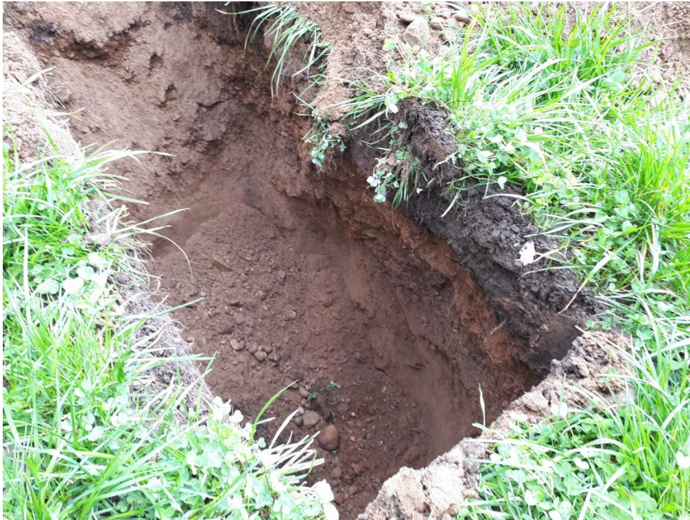
Trial Pit 12 – Pit Walls
