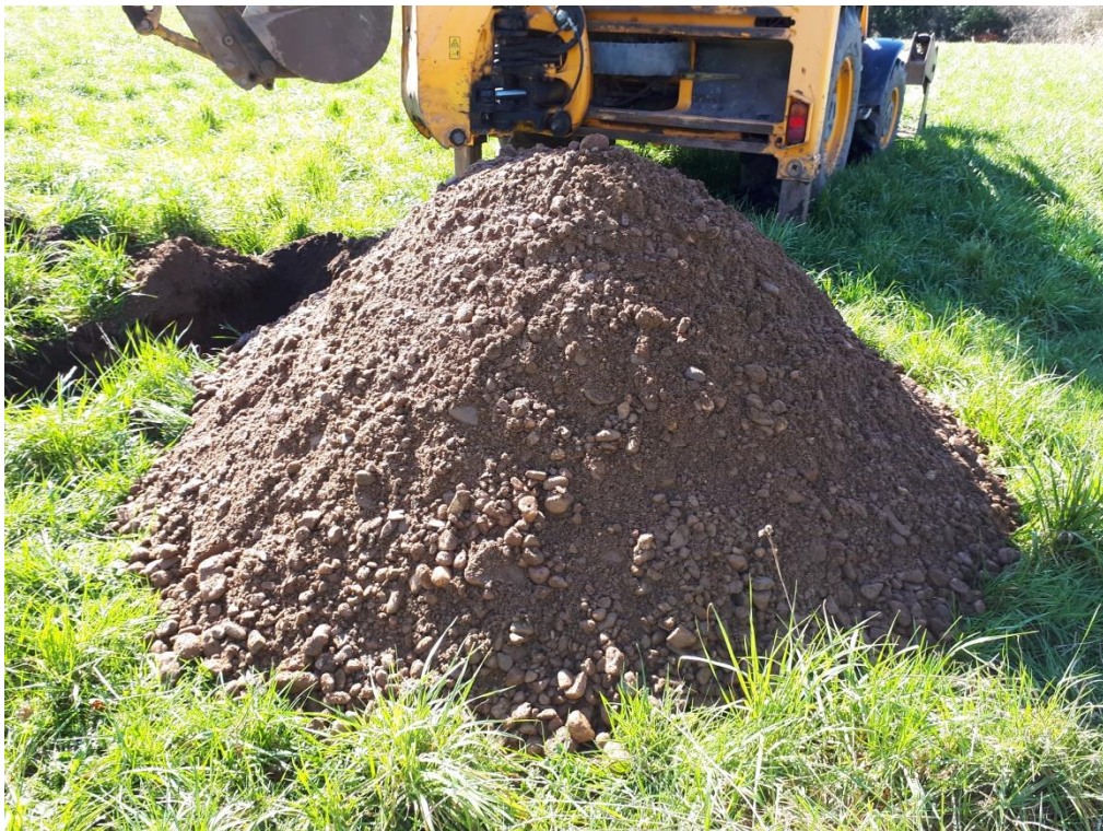
Trial Pit 02 - Arisings
