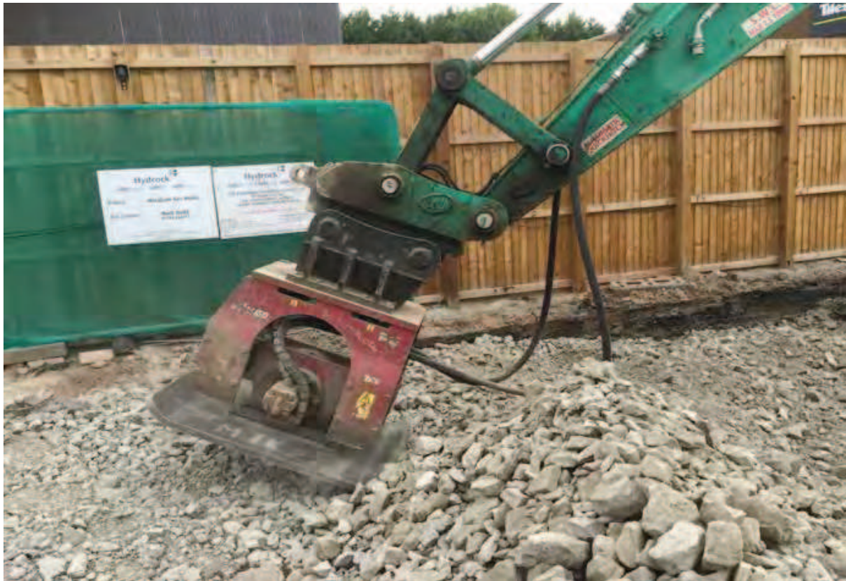
Photo (57): Backfilling and compaction of imported 6F5 to Excavation Area 12
