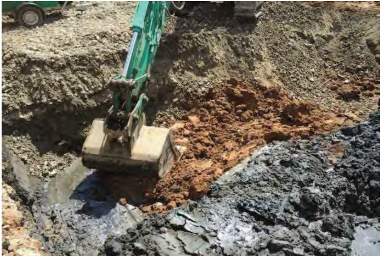
Photo (49): Imported clay being placed in base of Excavation Area 12 to act as a barrier above sands and gravels
