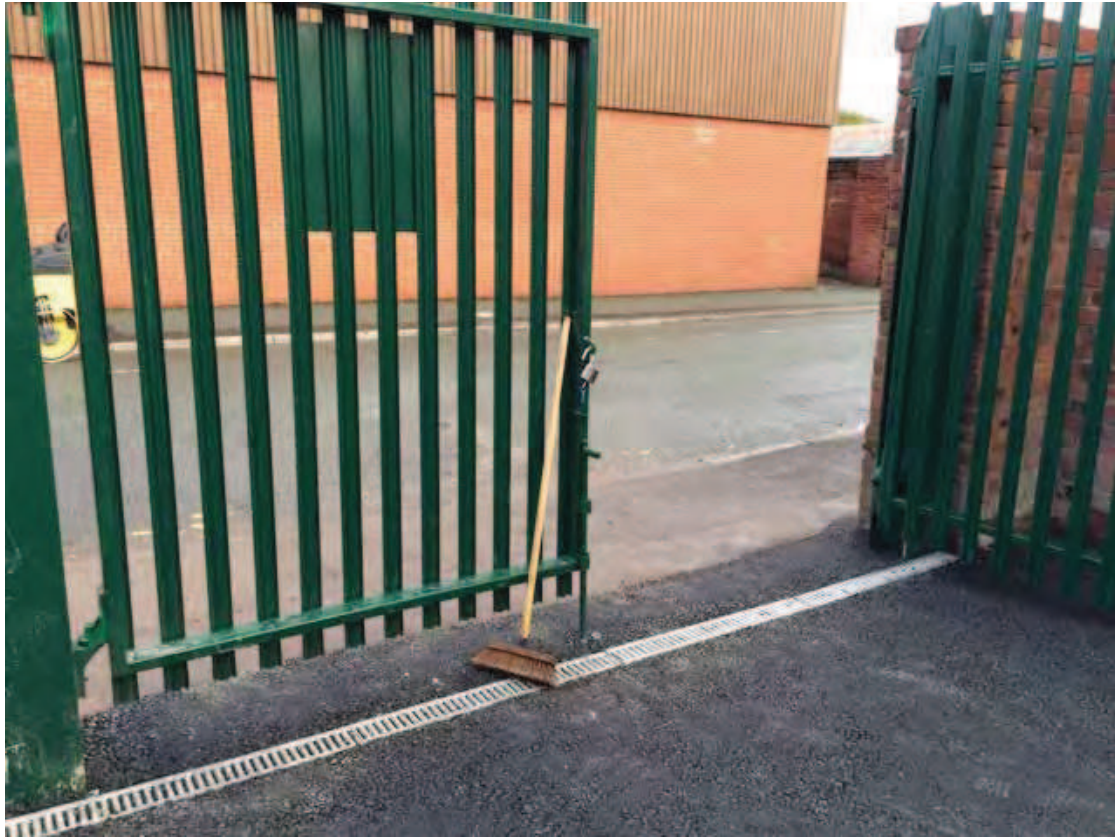
Photo (79): PRI compound newly installed palisade gate, tarmac ramp and aco drainage channel
