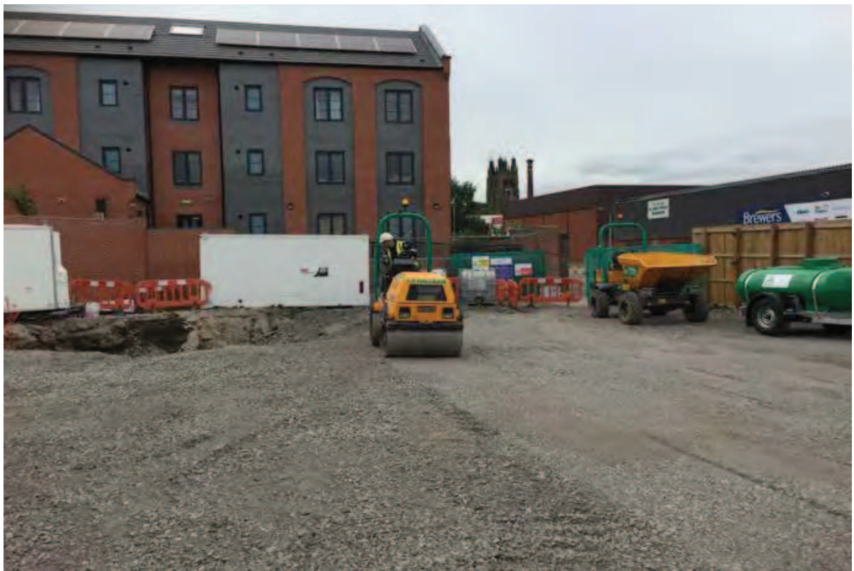
Photo (66): Compaction of 300mm Type 1 capping layer across entire site
