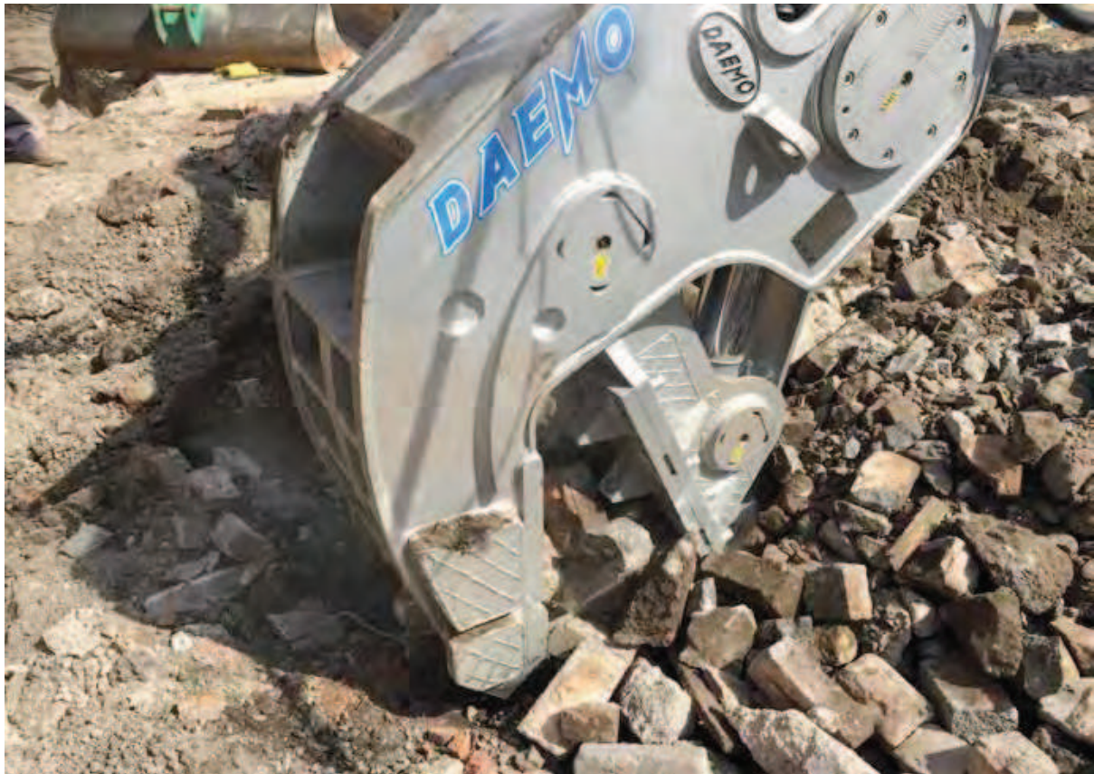
Photo (5): Crushing for site-won bricks to produce reusable aggregate for backfill
