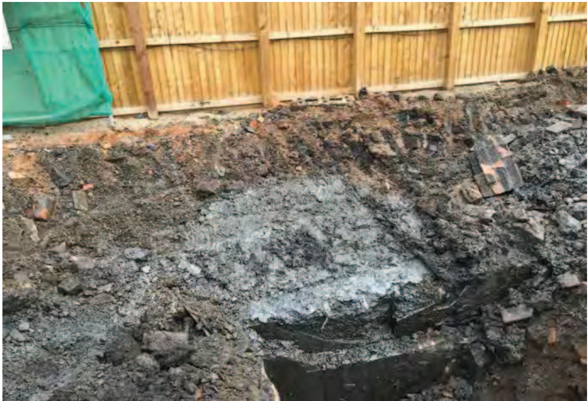
Photo (45): Northern edge of tar tank following removal of asbestos cement debris and slate
