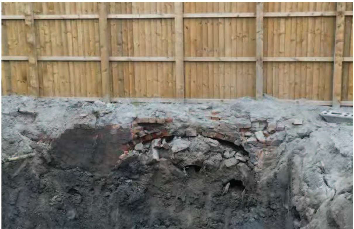
Photo (38): Brick archway extending from Excavation Area 11 off-site towards Rivulet Road
