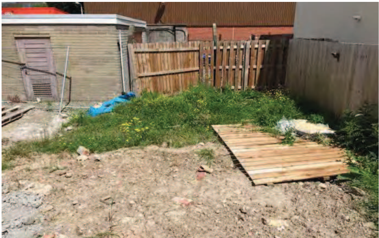
Photo (2): Site prior to start of works looking south towards electrical sub station.
