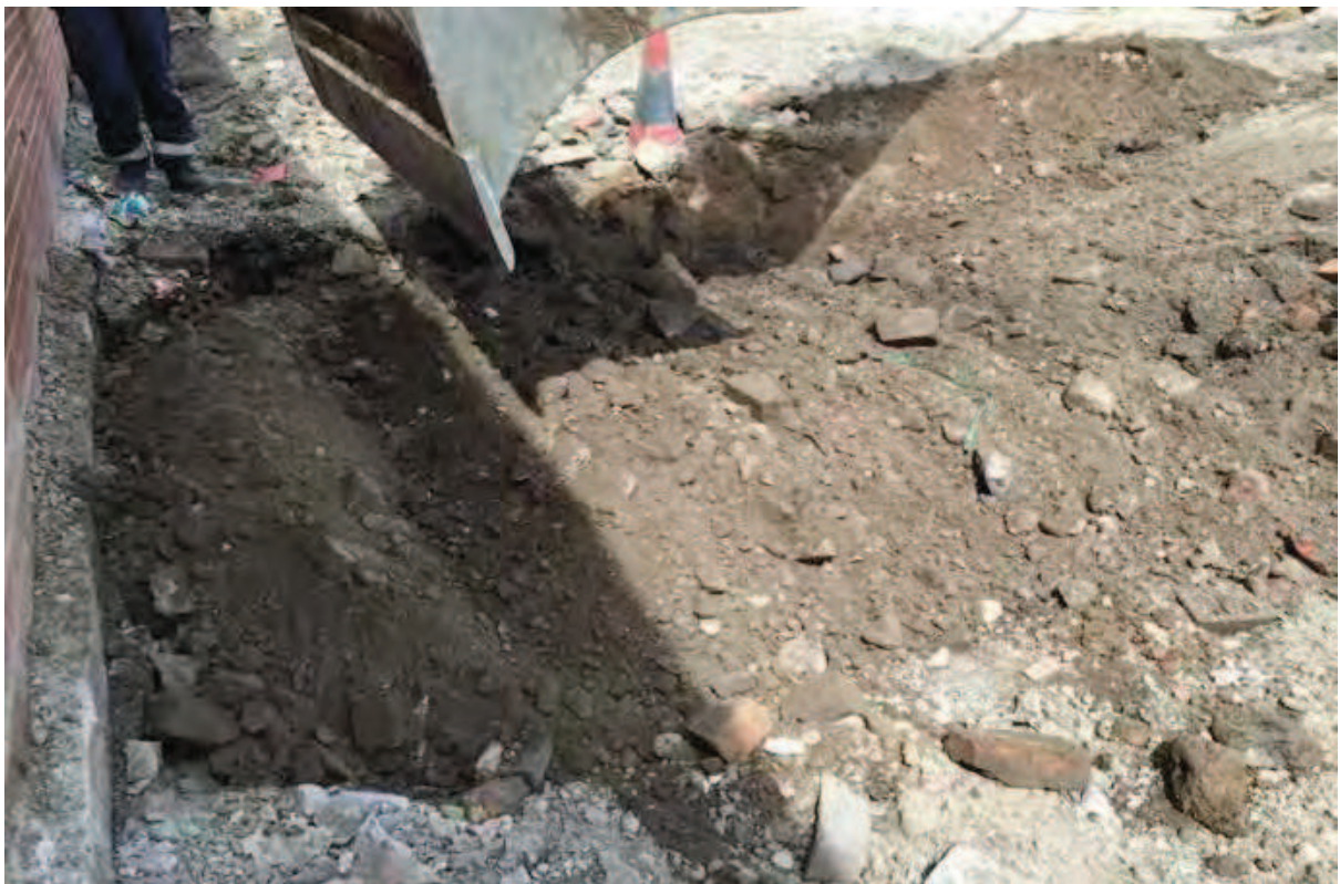
Photo (16): Backfilling of Excavation Area 5 with site-won material to 300mm below Final Finished Level
