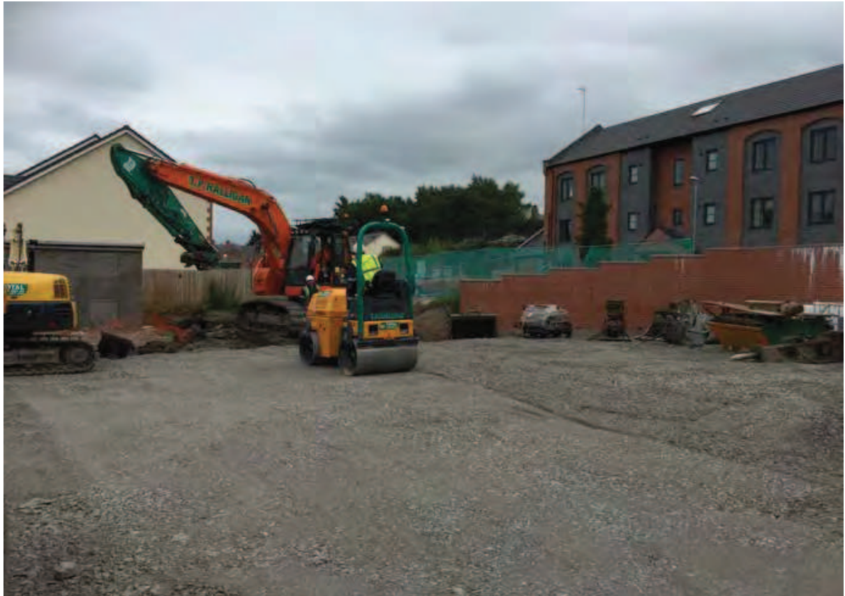
Photo (65): Compaction of 300mm Type 1 capping layer across entire site
