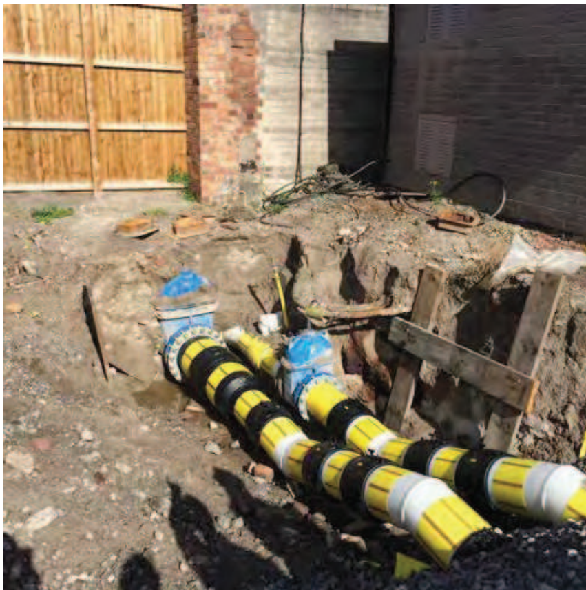
Photo (74): Newly installed WWU gas infrastructure and valves to the west of the substation
