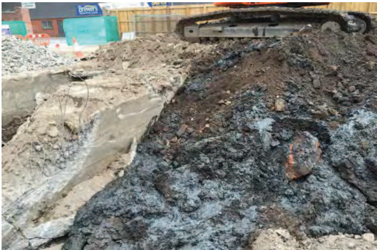
Photo (26): Material excavated from Excavation Area 9
