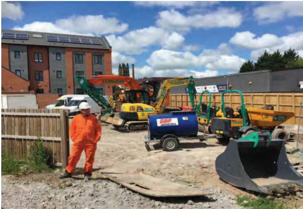
Photo (3): Site prior to starting works, looking west
