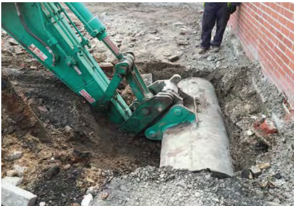
Photo (18): Excavation Area 6 adjacent to retaining wall
