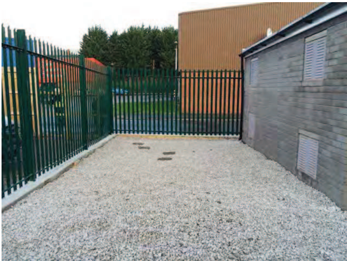
Photo (76): Completed PRI compound with fencing and capping layer in place
