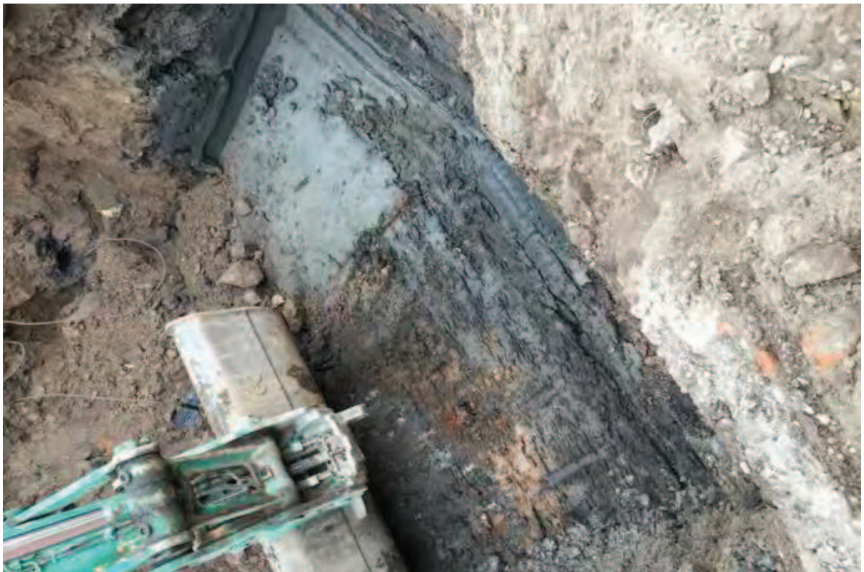
Photo (22): Base of Excavation Area 7 – visually unimpacted clay encountered at depth of 3m
