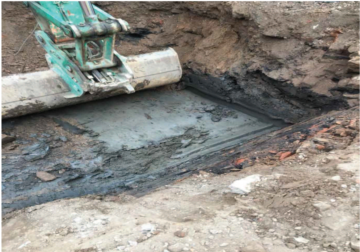
Photo (23): Base of Excavation Area 8 – visually unimpacted clay encountered at 1.5m
