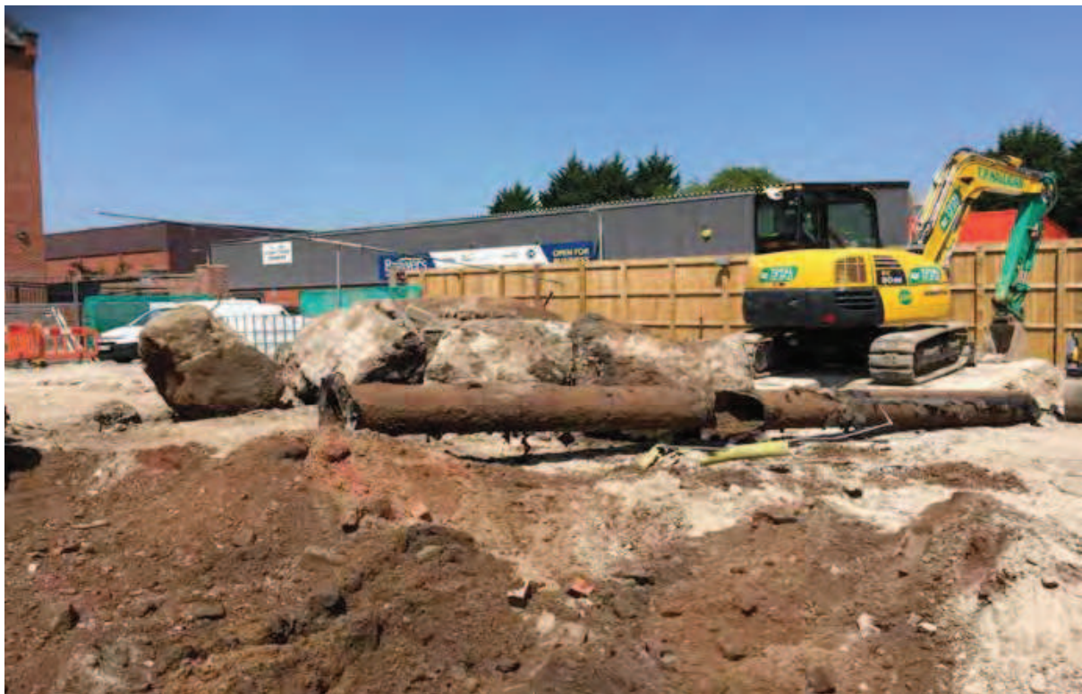
Photo (6): Removal of concrete underground structures adjacent to retaining wall to facilitate excavations
