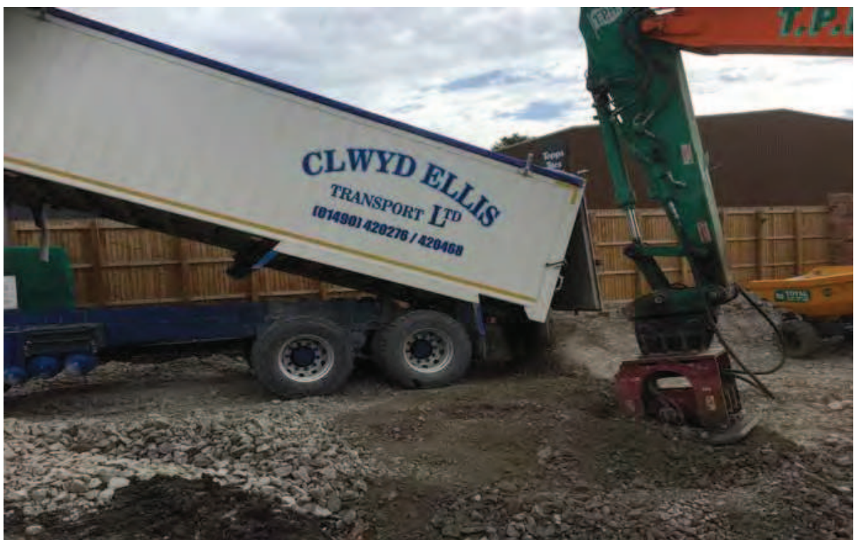
Photo (56): Import of primary 6F5 to backfill Excavation Area 12
