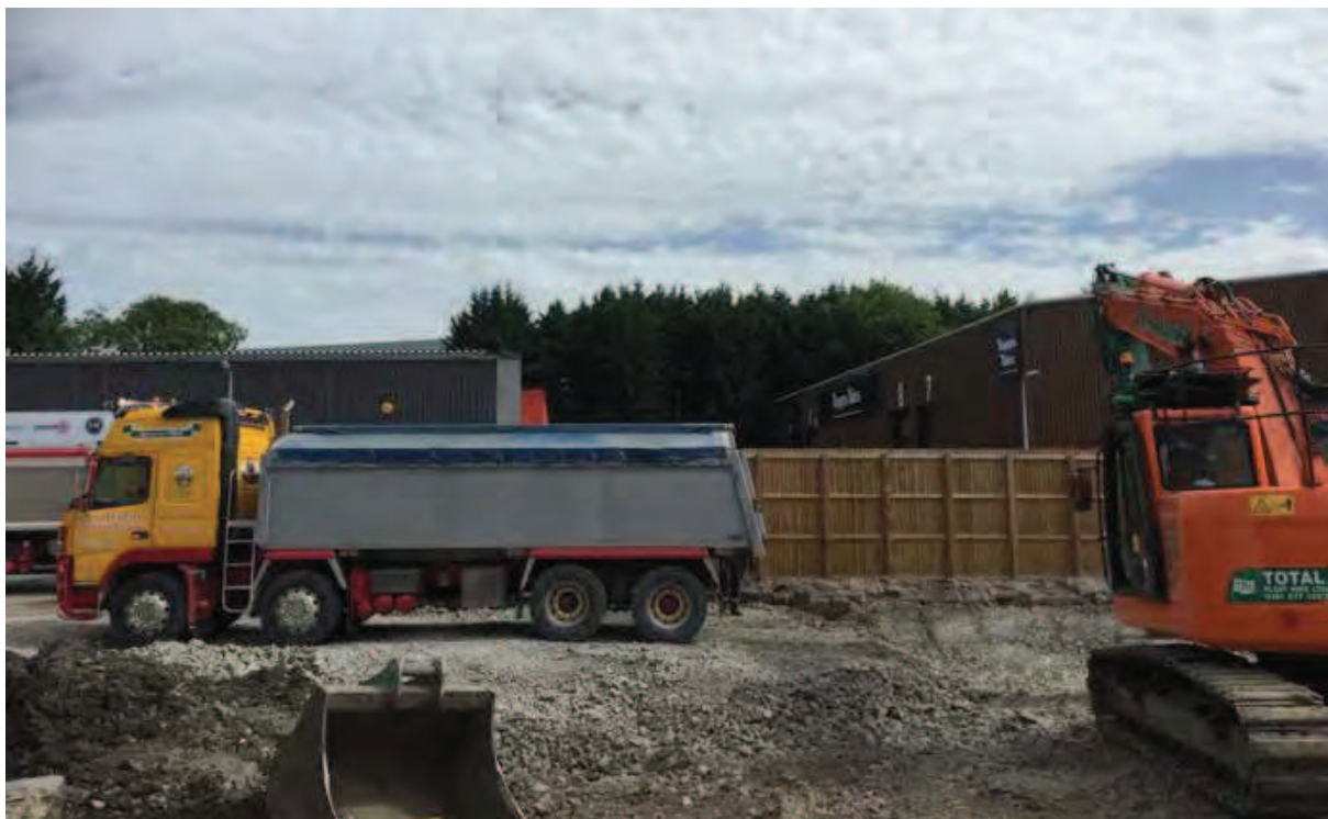
Photo (58): Import of primary 6F5 to backfill Excavation Area 12 within 300mm of Final Finished Levels
