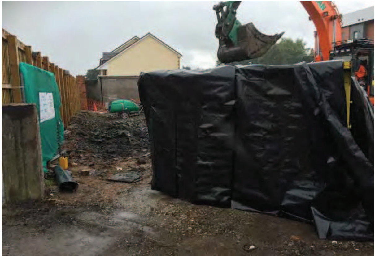
Photo (41): Excavation of tar tank under Notifiable Non Licensed Works
