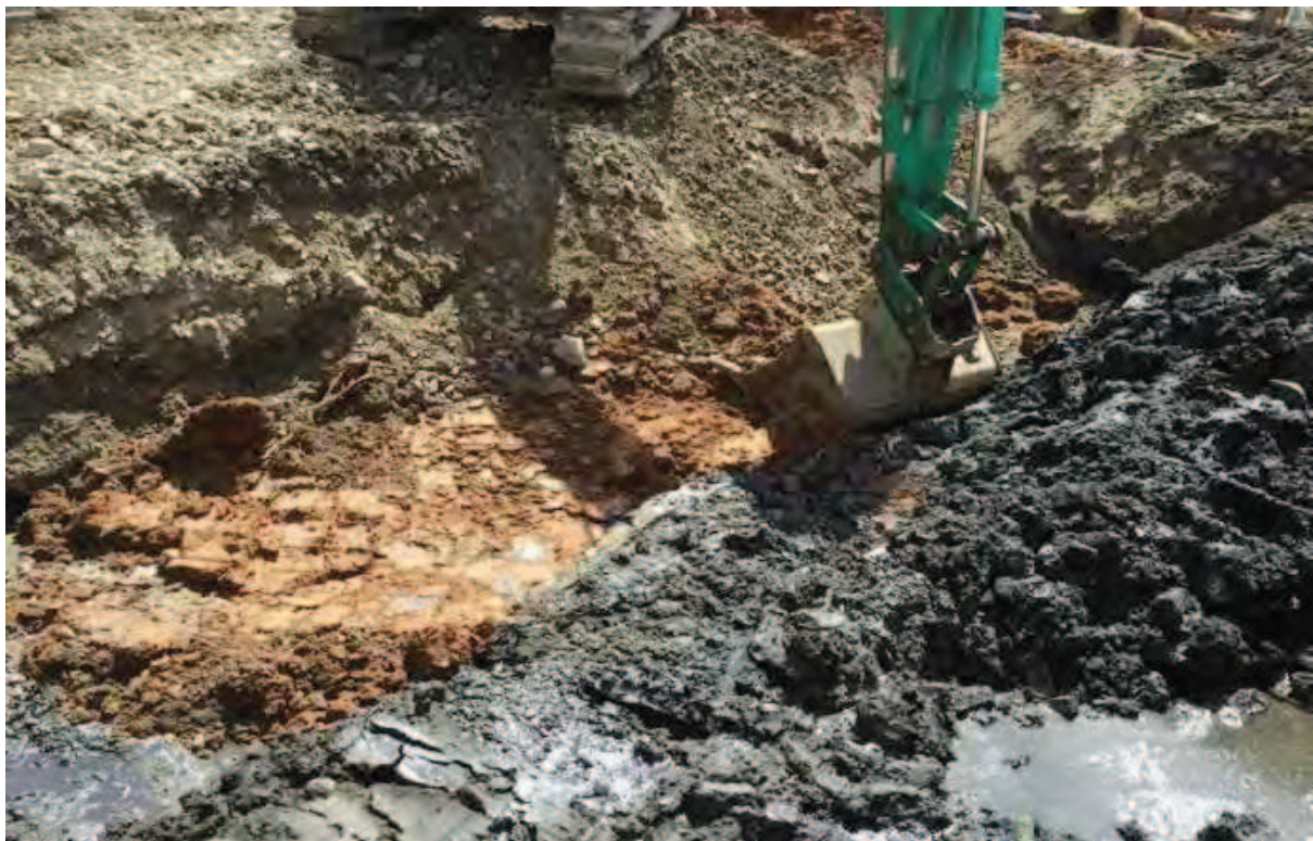
Photo (50): Imported clay being placed in base of Excavation Area 12 to act as a barrier above sands and gravels
