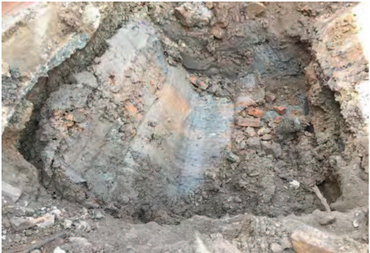
Photo (10): Excavation Area 1 – clay used to seal under retaining wall
