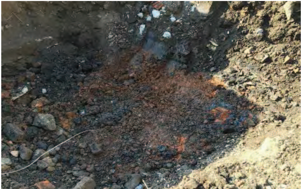
Photo (34): Base of Excavation Area 10 – visually unimpacted clay encountered at depth of 2.5m
