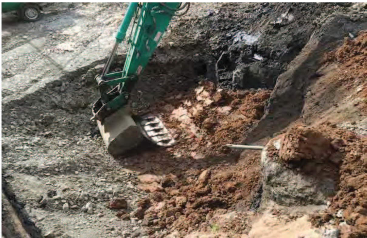
Photo (54): Imported clay being placed in base of Excavation Area 12 to act as a barrier above the sands and gravels
