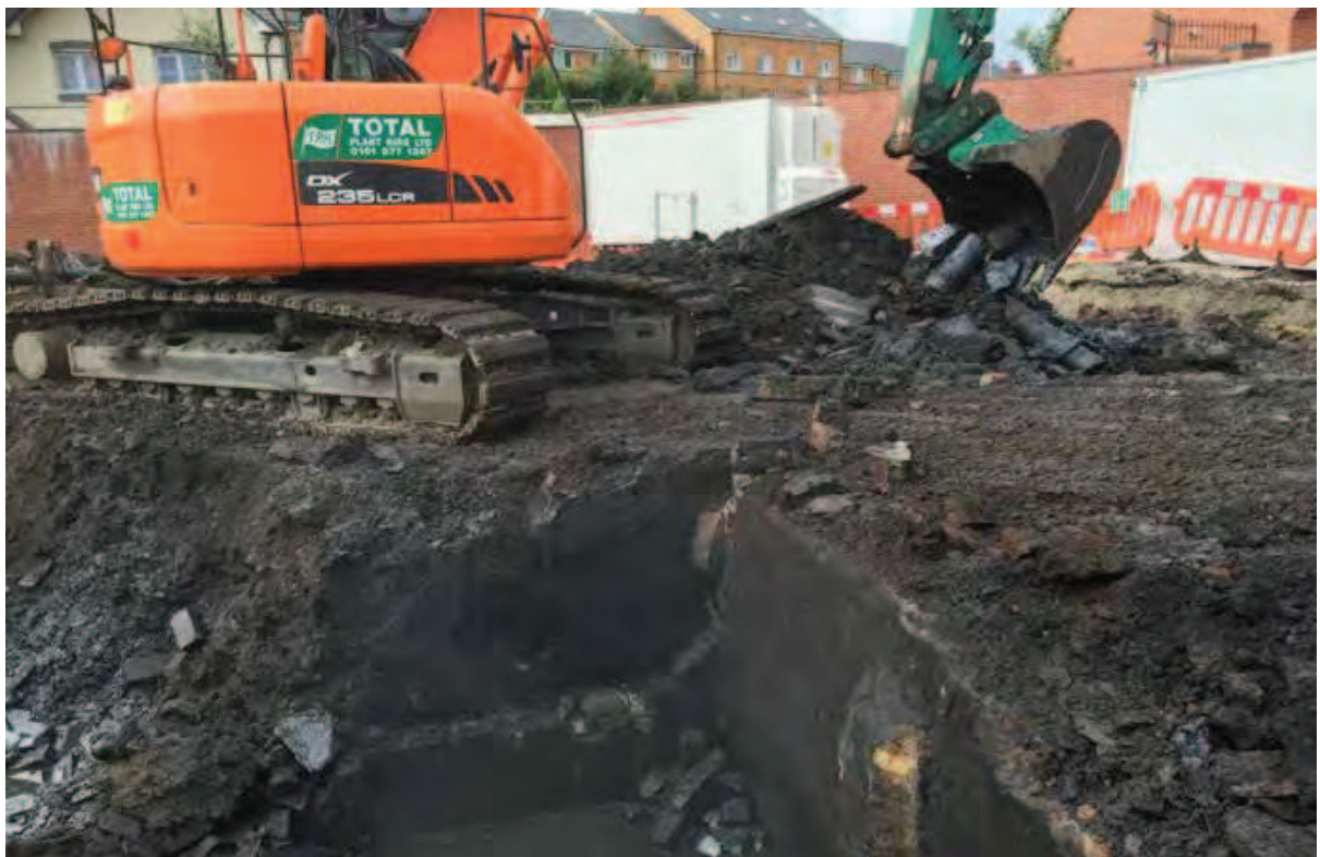
Photo (44): Southern and eastern edges of tar tank following removal of asbestos cement debris and slate
