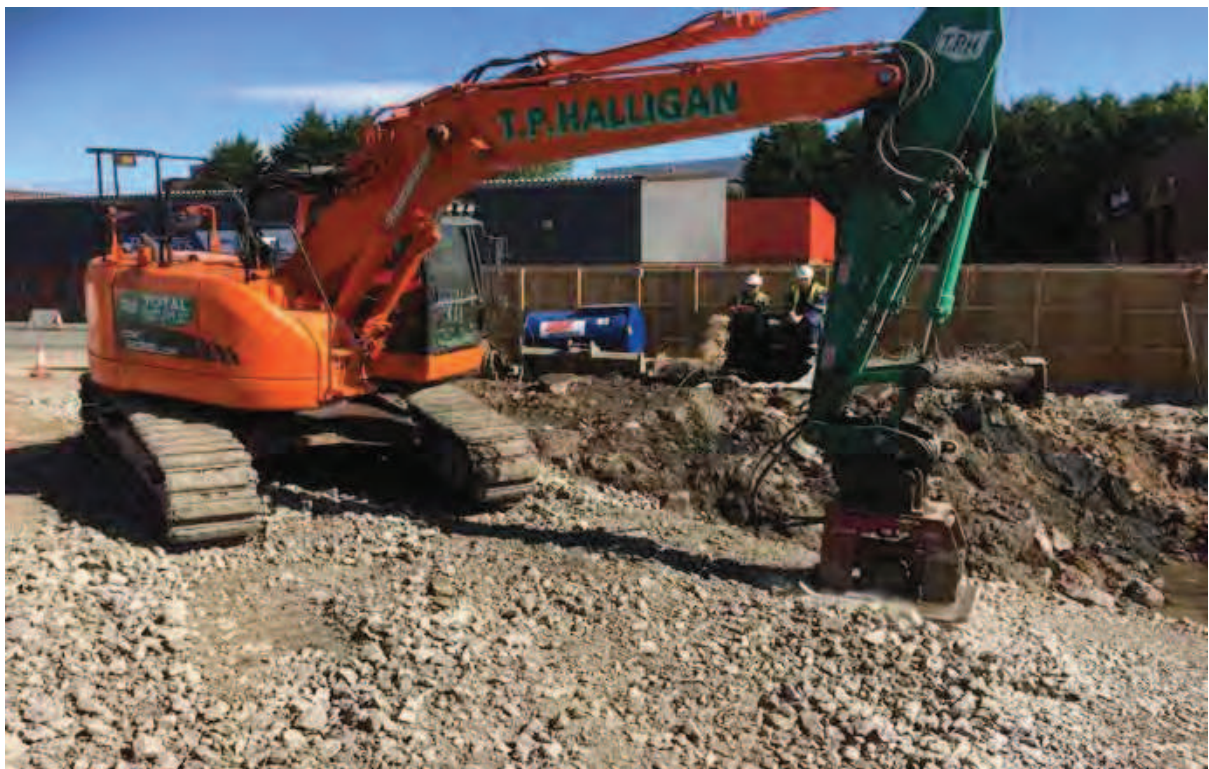
Photo (32): Compaction of imported primary 6F5 used to backfill Excavation Area 9 to 300mm of Final Finished Levels
