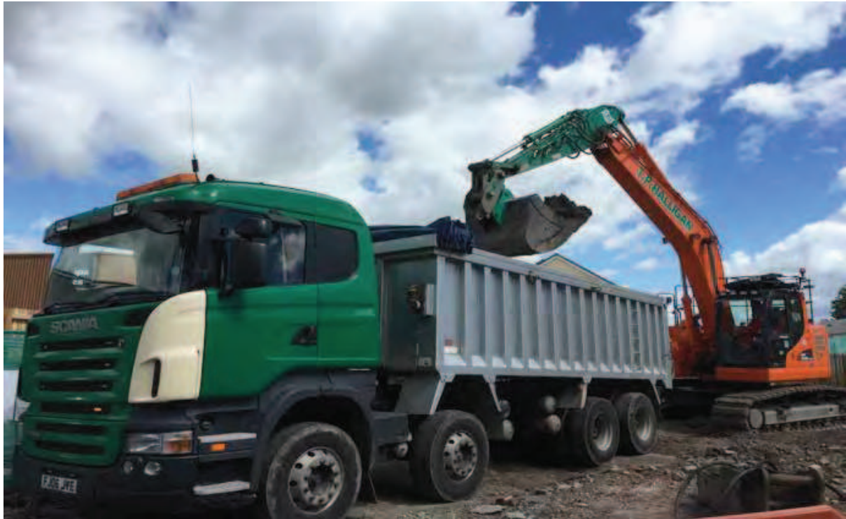
Photo (25): Loading eight wheel tipper lorry with hazardous material for offsite disposal.
