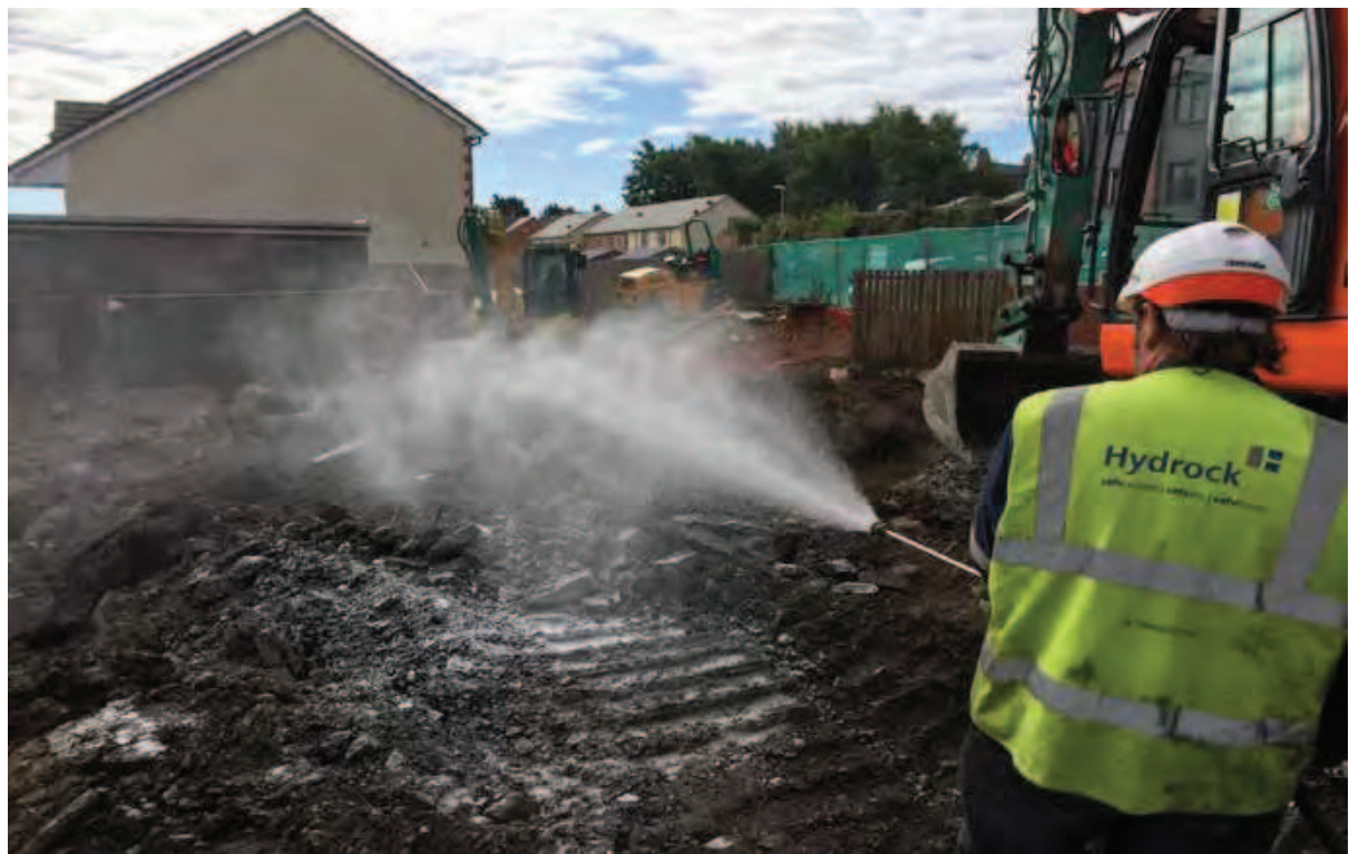
Photo (30): Spraying excavated material with odour supressing foam prior to offsite disposal
