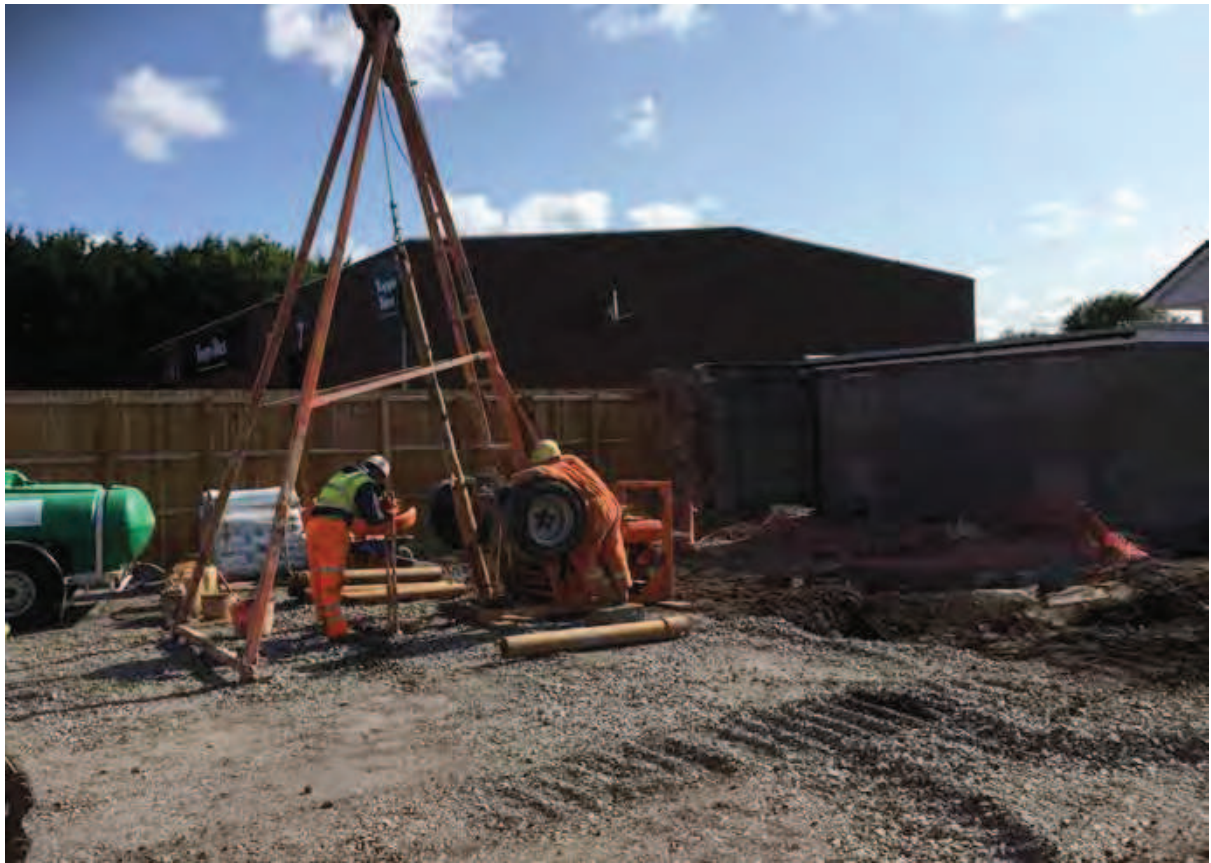
Photo (67): Drilling of groundwater extraction wells
