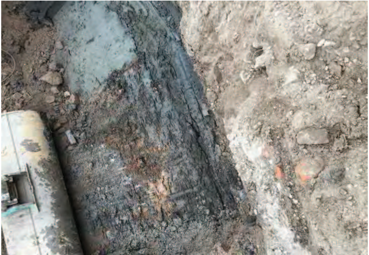
Photo (21): Base of Excavation Area 7 – visually unimpacted clay encountered at depth of 3m
