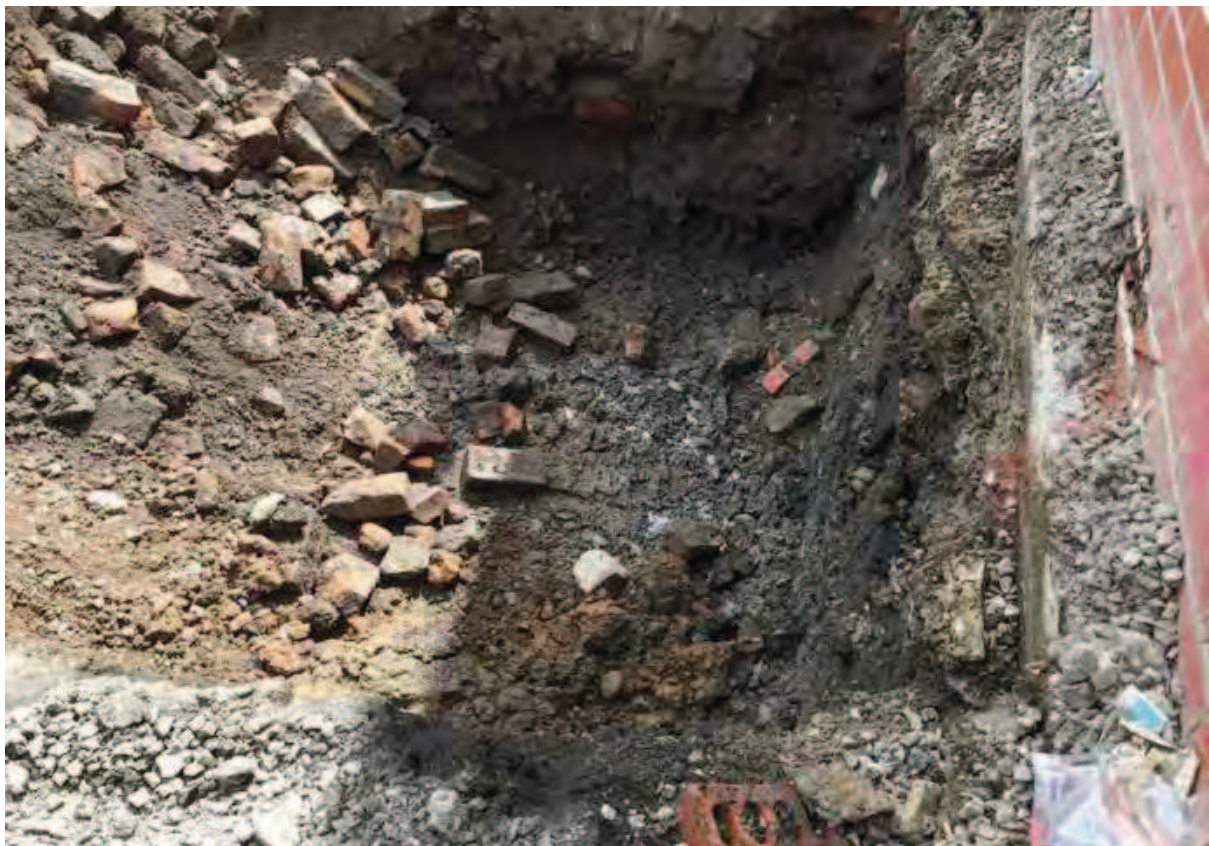
Photo (14): Base Excavation Area 4 – Visually unimpacted clay encountered at depth of 1.5m
