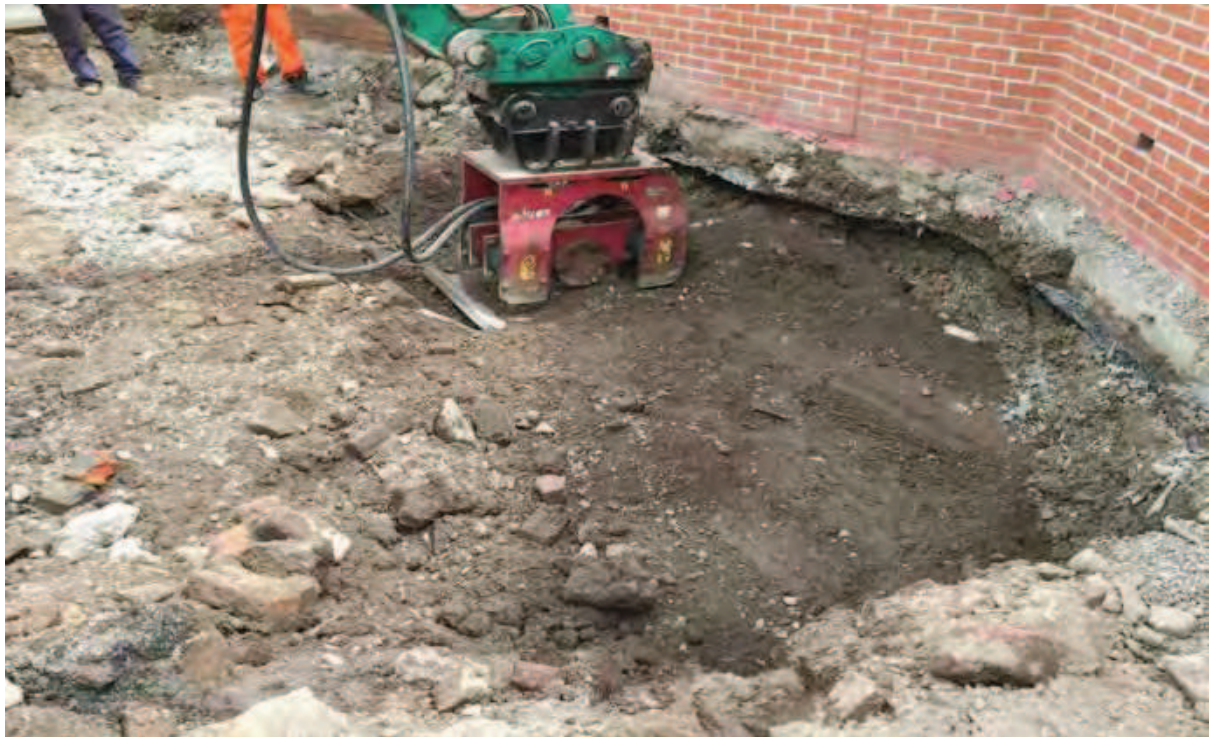
Photo (13): Backfilling of Excavation Area 3 with site-won material to 600mm below Final Finish Level
