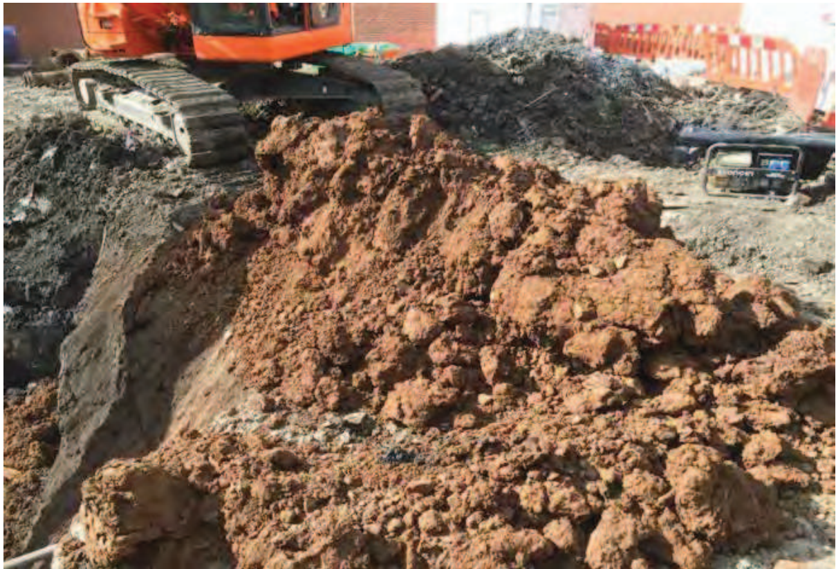
Photo (53): Imported clay being placed on the base of Excavation Area 12 to act as a barrier above the sands and gravels
