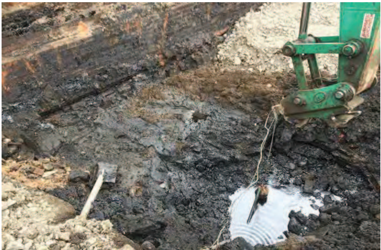
Photo (52): Dewatering of hydrocarbon impacted perched water from Excavation Area 12
