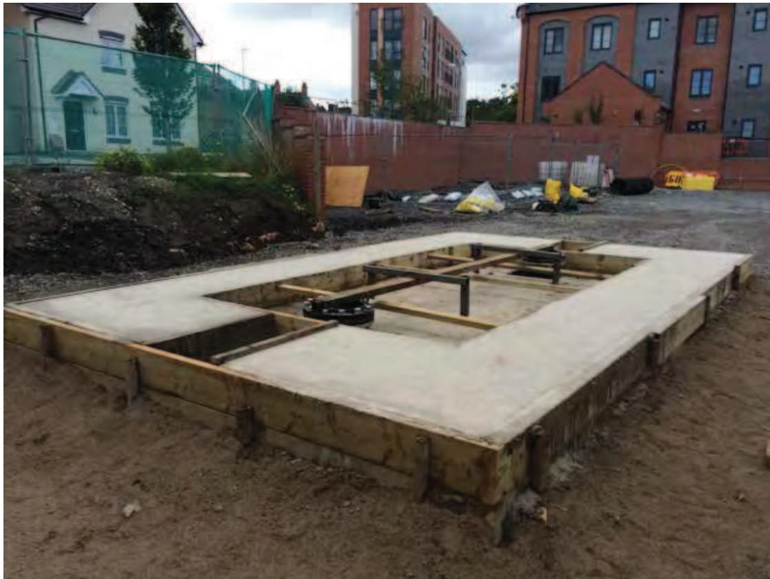
Photo (75): Works in progress to construct the WWU PRI slab
