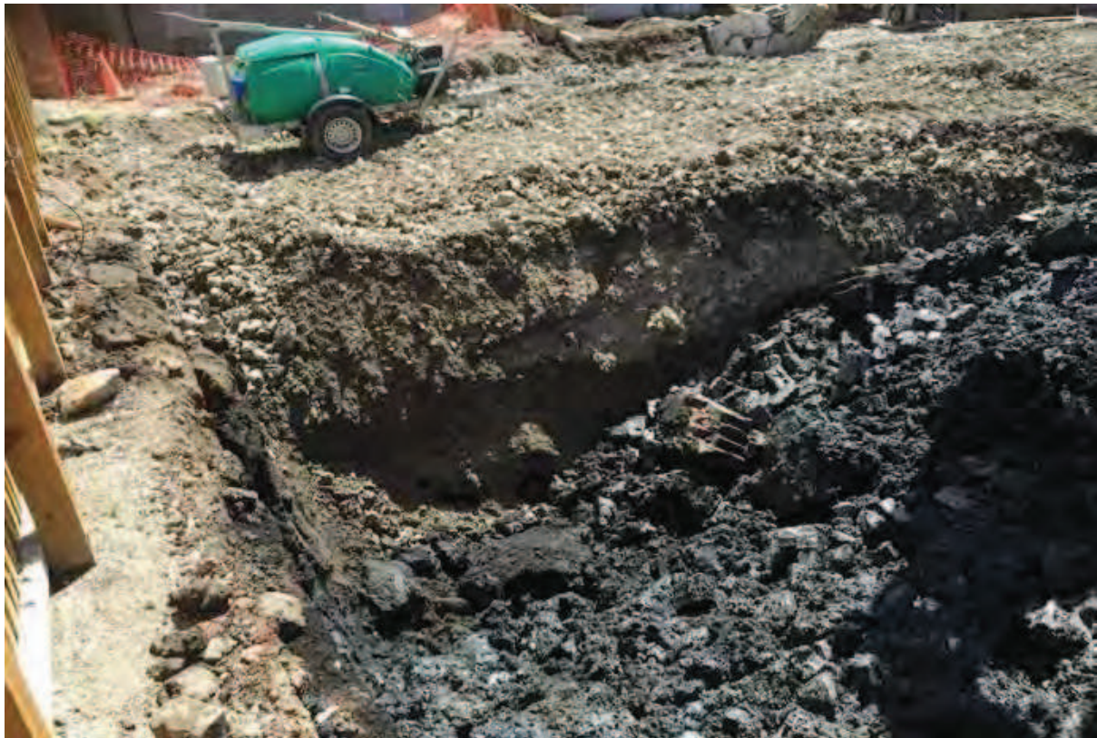
Photo (47): Excavation of Excavation Area 12 surrounding tar tank
