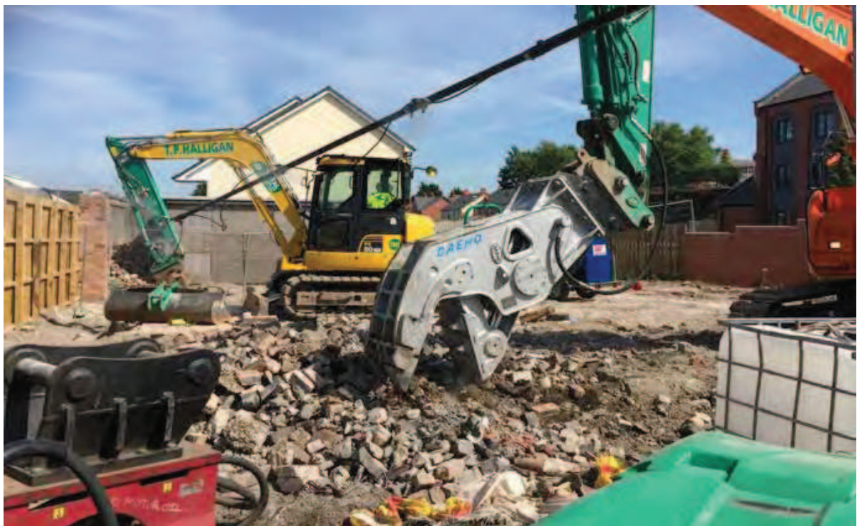
Photo (4): Crushing of site-won bricks to produce reusable aggregate for backfill.
