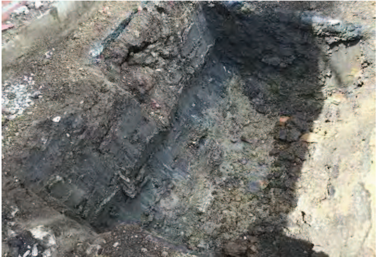
Photo (19): Base of Excavation Area 6 – visually unimpacted clay encountered at depth of 1.5m
