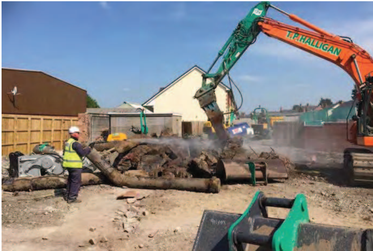
Photo (7): Breaking concrete underground structures with pneumatic breaker.
