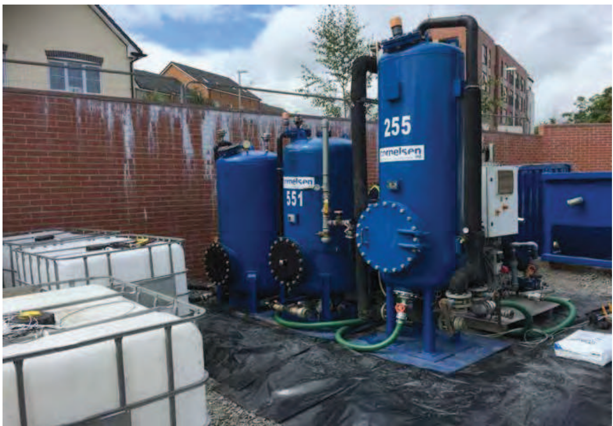
Photo (70): Installation of ground water treatment plant
