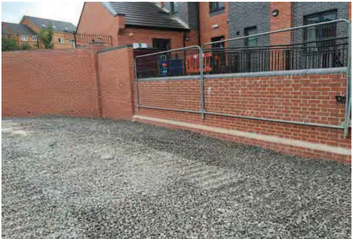
Photo (72): Site following completion of works looking west
