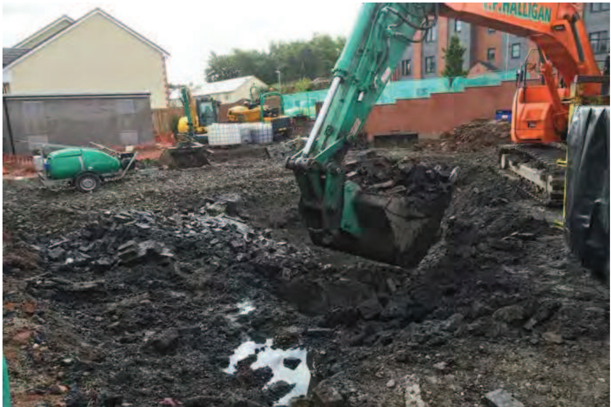
Photo (42): Excavation of tar tank under Notifiable Non Licensed Works
