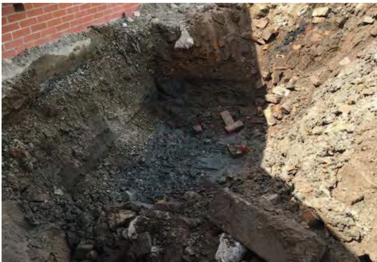
Photo (11): Base Excavation Area 2 – Visually unimpacted clay encountered at depth of 1.5m
