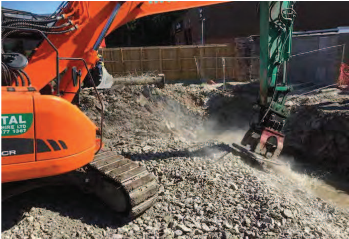
Photo (31): Compaction of imported primary 6F5 used to backfill Excavation Area 9 to 300mm of Final Finished Levels
