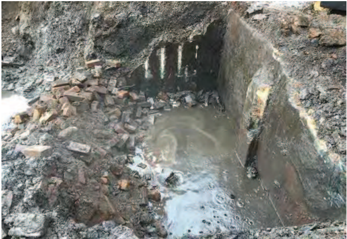
Photo (43): Western edge of tar tank following removal of asbestos cement debris and slate
