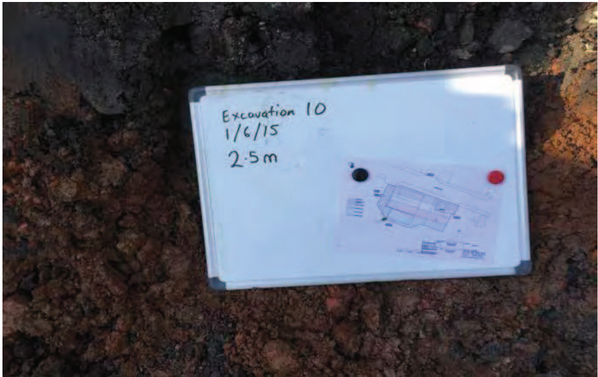
Photo (33): Base of Excavation Area 10 – visually unimpacted clay encountered at depth of 2.5m
