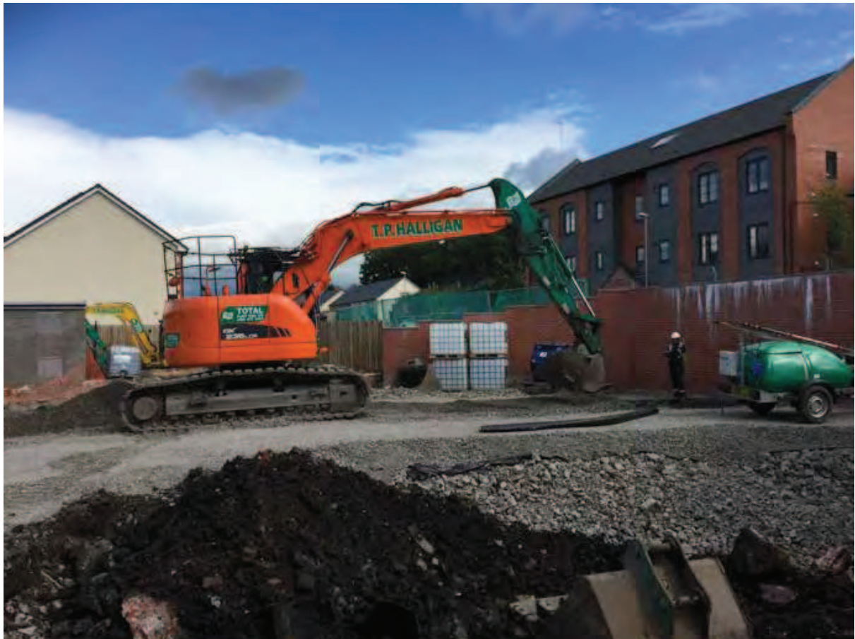
Photo (63): Placement of Terram and 300mm Type 1 capping layer across entire site
