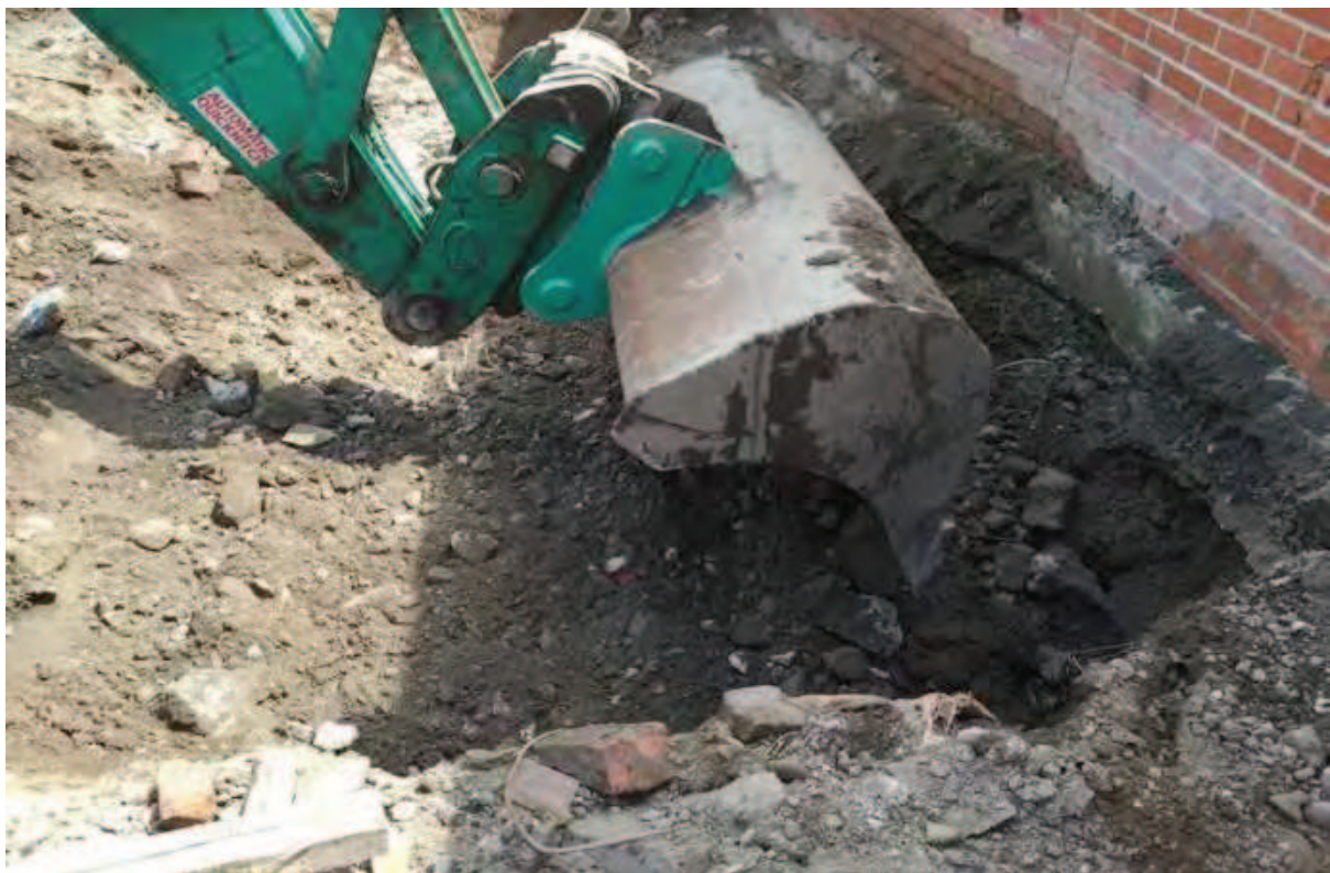
Photo (8): Excavation Area 1 adjacent to retaining wall
