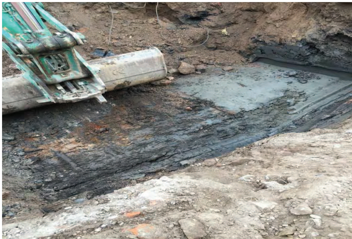
Photo (24): Base of Excavation Area 8 – visually unimpacted clay encountered at depth of 1.5m
