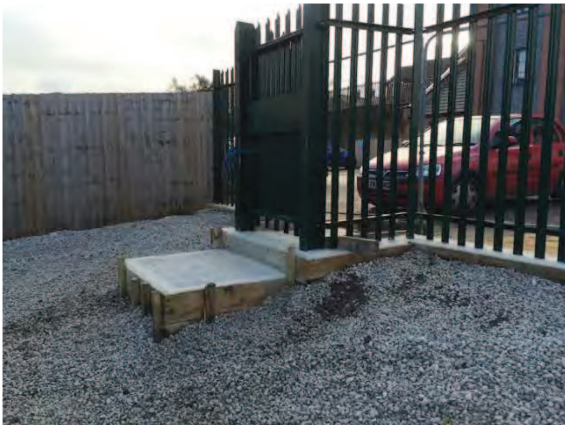
Photo (78): PRI compound pedestrian panic gate and access steps under construction
