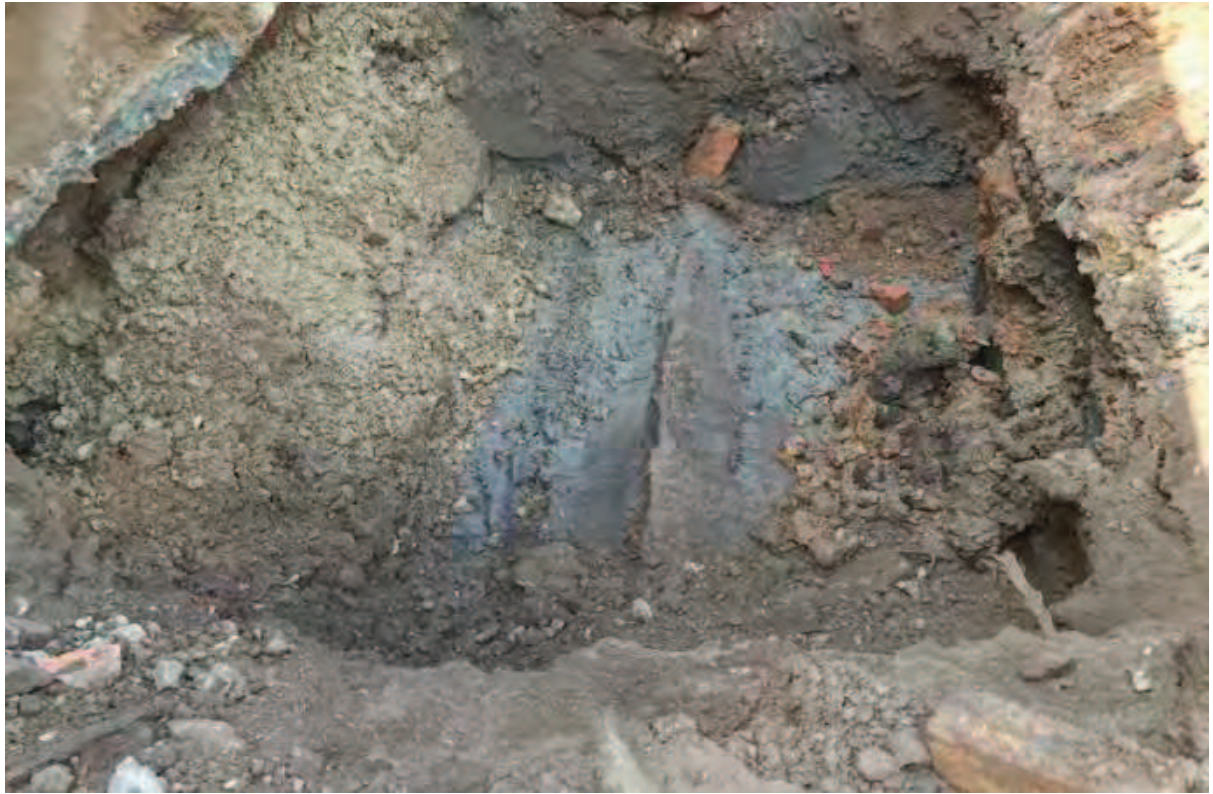
Photo (9): Base of Excavation Area 1 – Visually unimpacted clay encountered at depth of 1.5m
