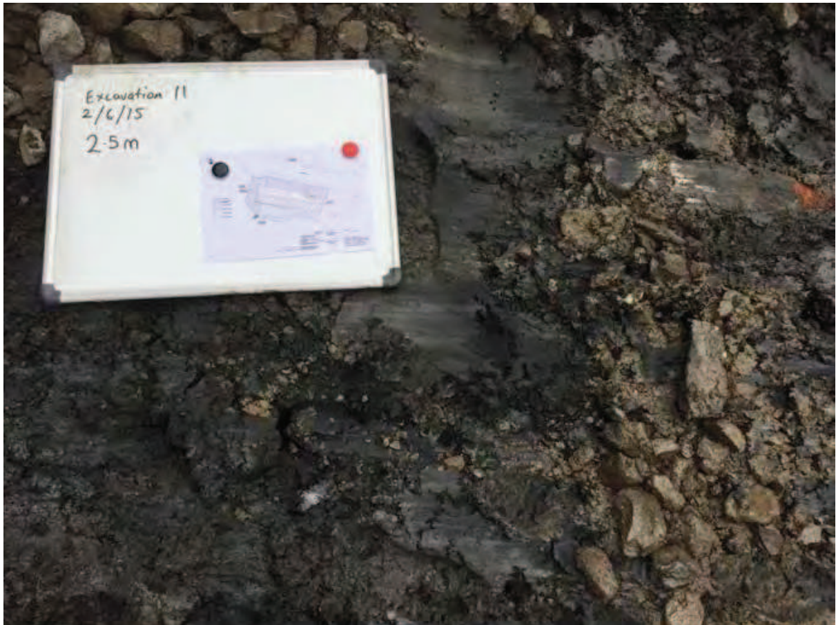
Photo (37): Base of Excavation Area 11 – visually unimpacted clay encountered at depth 2.5m
