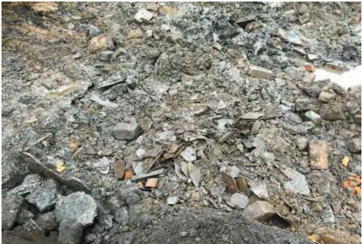
Photo (40): Tar tank backfilled with slate and asbestos cement debris
