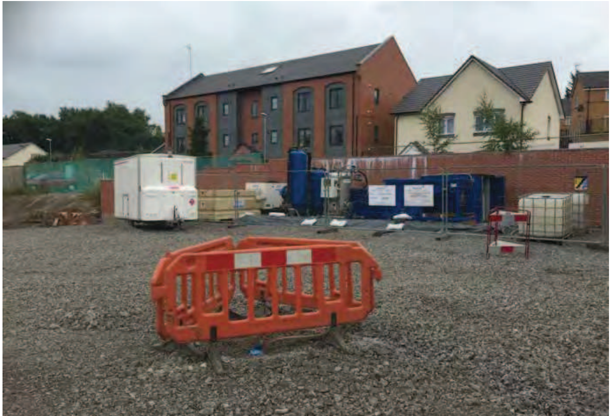
Photo (73): Site following completion of main site works looking south
