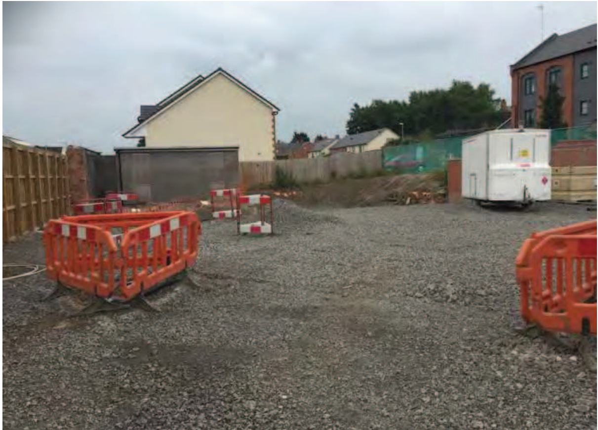
Photo (71): Site following completion of main site area works looking east
