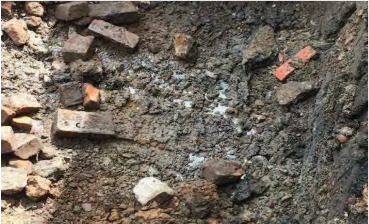
Photo (15): Base Excavation Area 5 – Visually unimpacted clay encountered at depth of 1.5m
