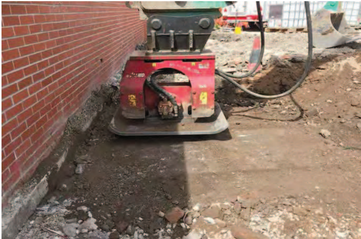
Photo (17): Compaction of backfill to Excavation Area 5
