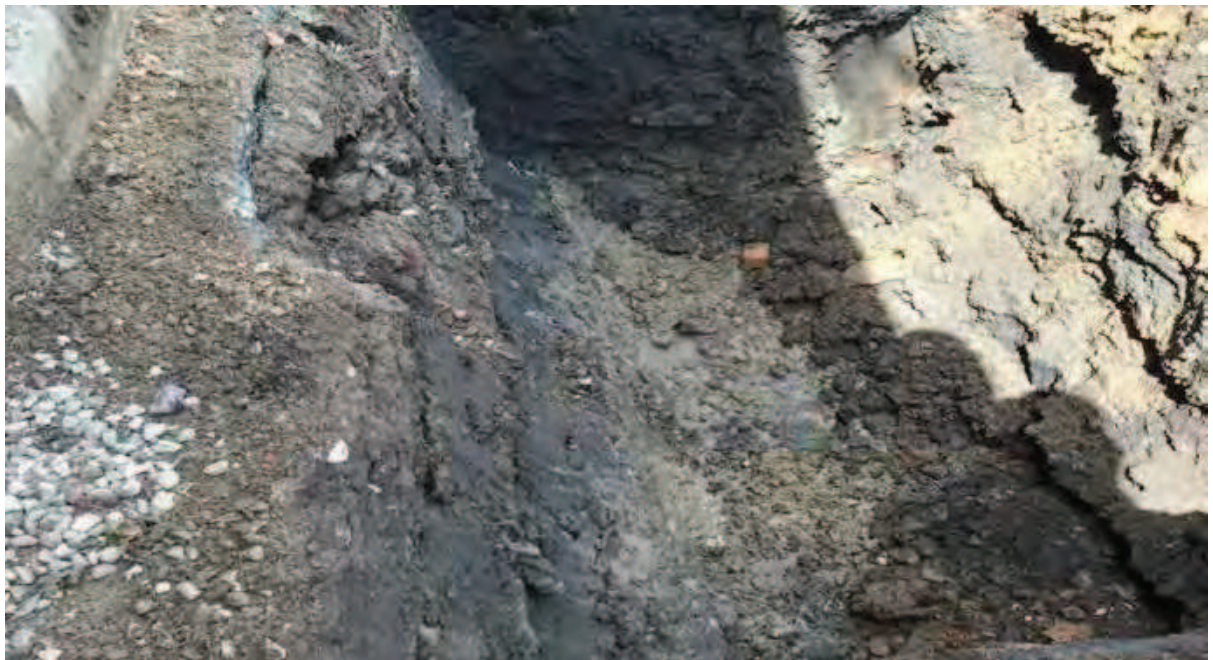
Photo (20): Base of Excavation Area 6 – visually unimpacted clay encountered at 1.5m
