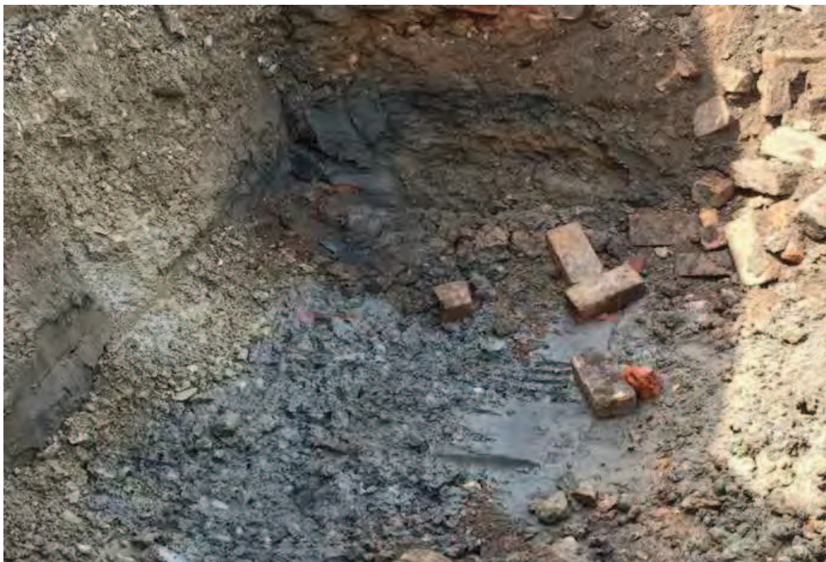
Photo (12): Base Excavation Area 3 – Visually unimpacted clay encountered at depth of 1.75m
