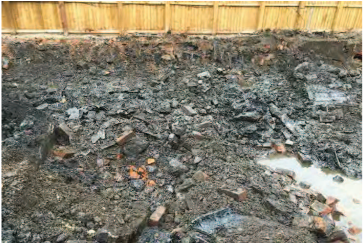
Photo (39): Excavation of Excavation Area 12 to expose tar tank
