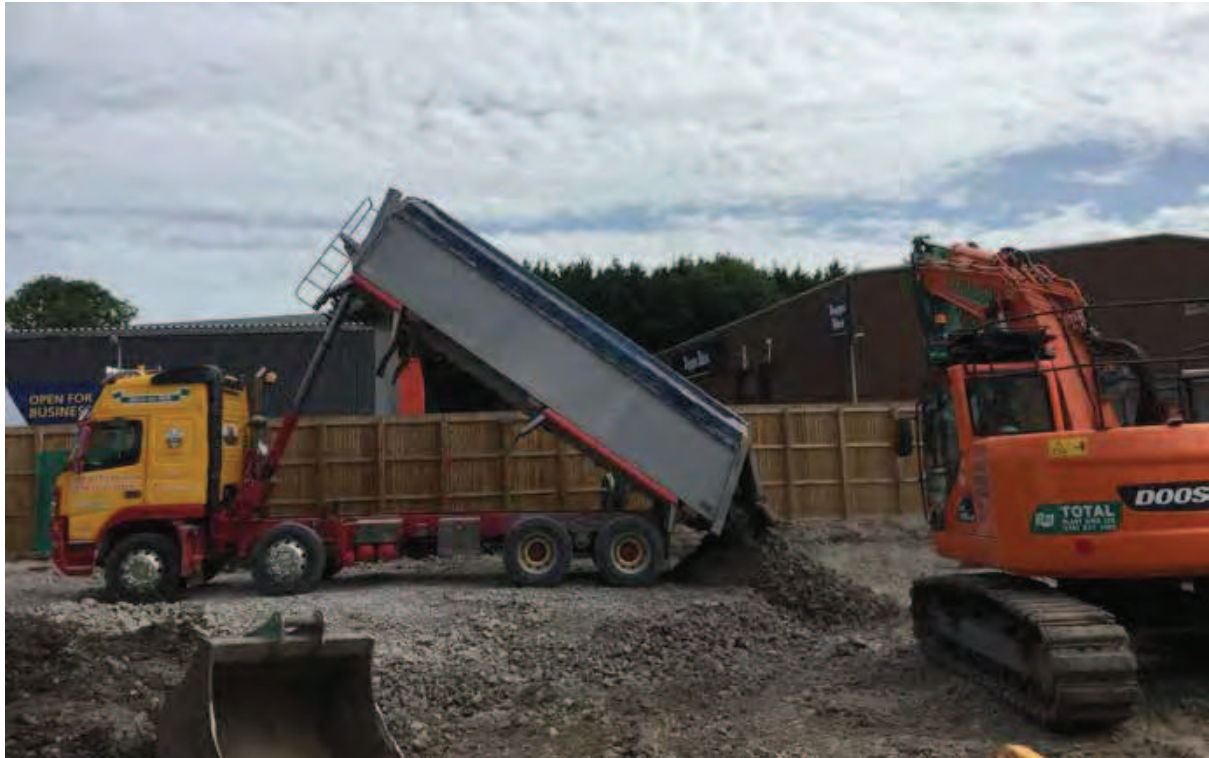
Photo (59): Import of primary 6F5 to backfill Excavation Area 12 within 300mm of Final Finished Levels
