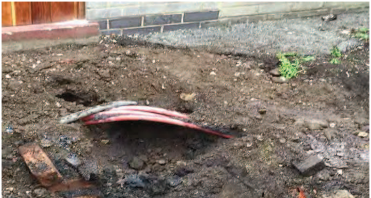
Photo (62): High Voltage cables following removal of tar impacted redundant gas pipe within excavation Area 14, by hand.
