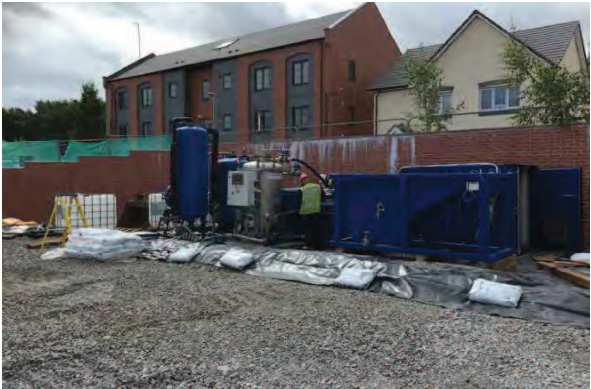
Photo (69): Installation of ground water treatment plant
