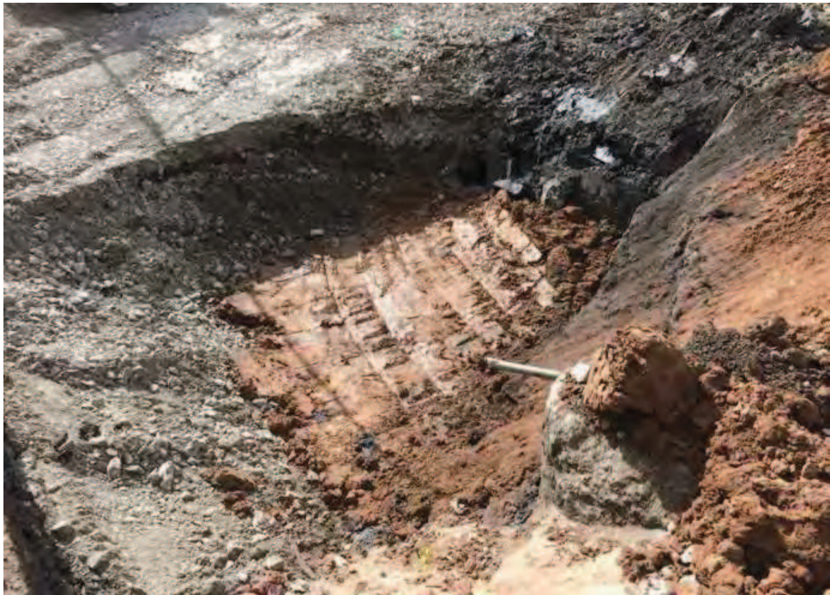
Photo (55): Imported clay being placed in base of Excavation Area 12 to act as a barrier above the sands and gravels
