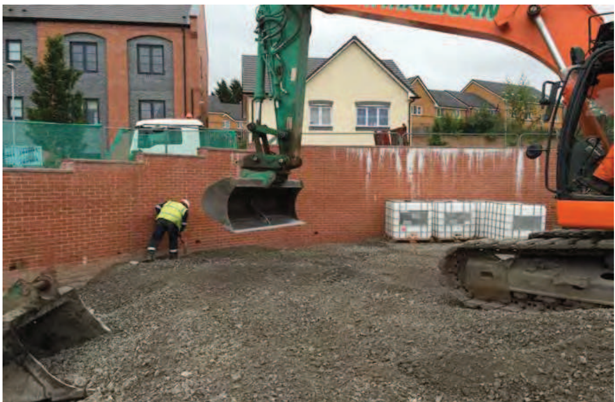
Photo (64): Placement of Terram and 300mm Type 1 capping layer across entire site
