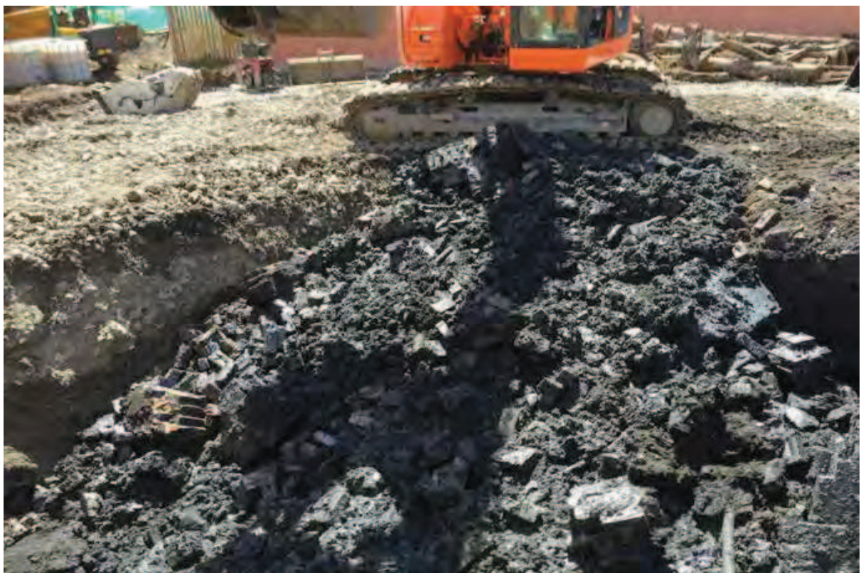
Photo (46): Material excavated from Excavation Area 12 surrounding tar tank
