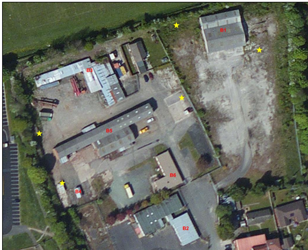
Photograph 1 showing buildings and approximate positions of surveyors (yellow stars) during emergence survey
