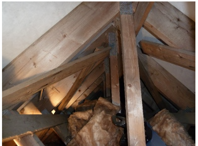
P6: Building 1 roof space.
