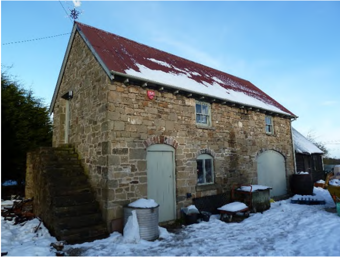
P1: Building 1 (southwest and southeast elevations).
