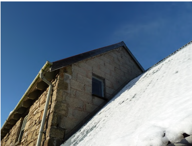
P3: Building 1 (southeast and northeast elevations).
