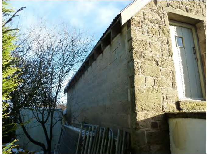
P2: Building 1 (northwest and southwest elevations).
