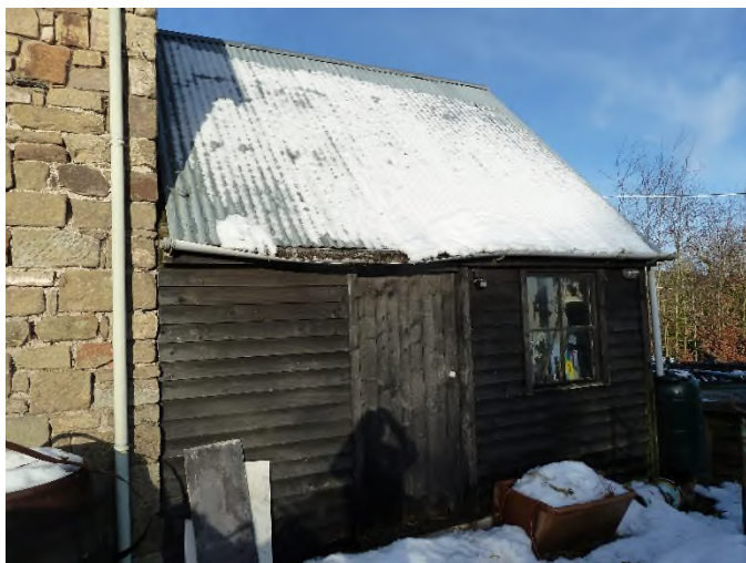
P7: Building 2 (southeast elevation).
