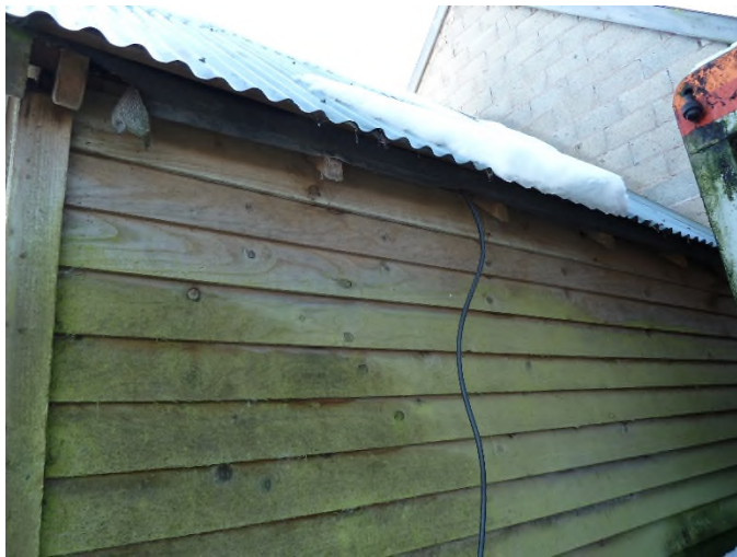
P9: Building 2 (northwest elevation).
