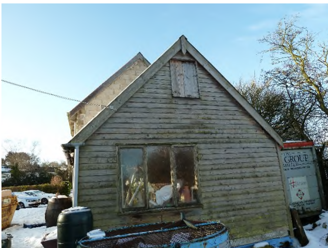
P8: Building 2 (northeast elevation).
