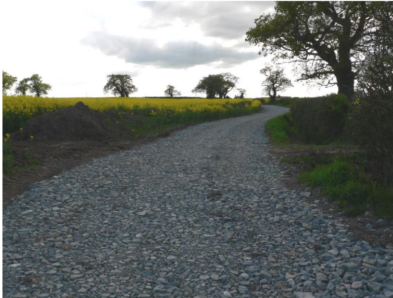
Photograph 9: Upgraded access track alongside hedge and ditch, April 2017
