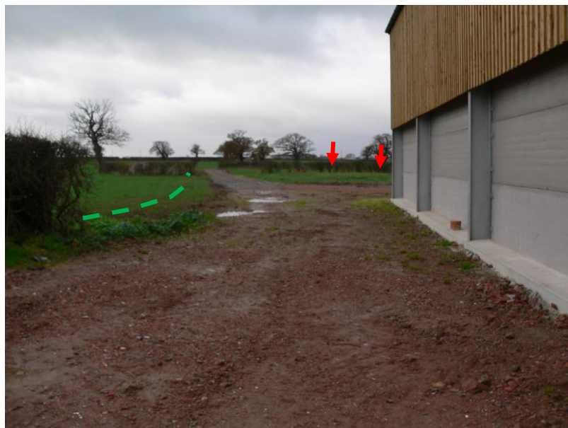
Photograph 8: access approaching new shed, December 2017. Red arrows = west field boundary. Green dashes = proposed new hedgerow
