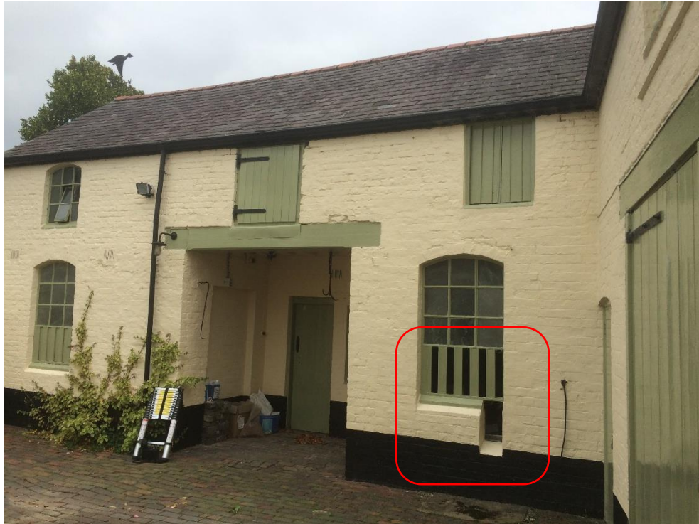
Photograph 7- External view of building 4 and Bat Access Point 2 (circled)
