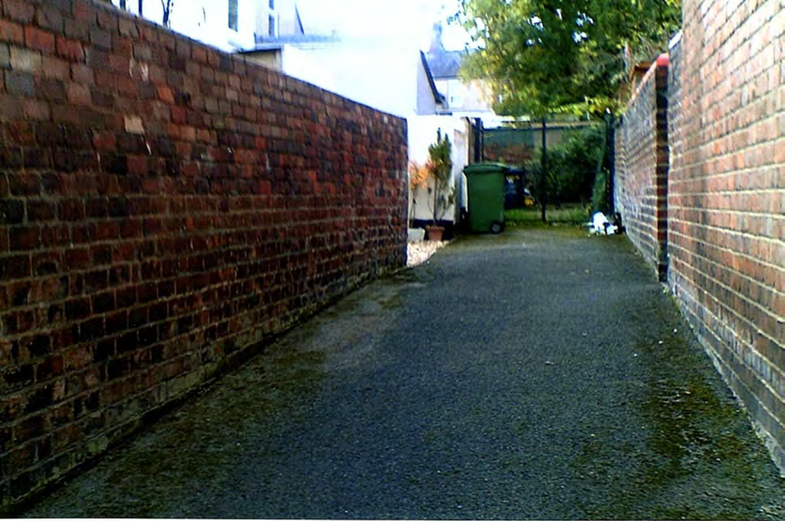
14/10/2017 Rear Access to No's 10-9-8 Albert Street & No.2 Greenbank Street
