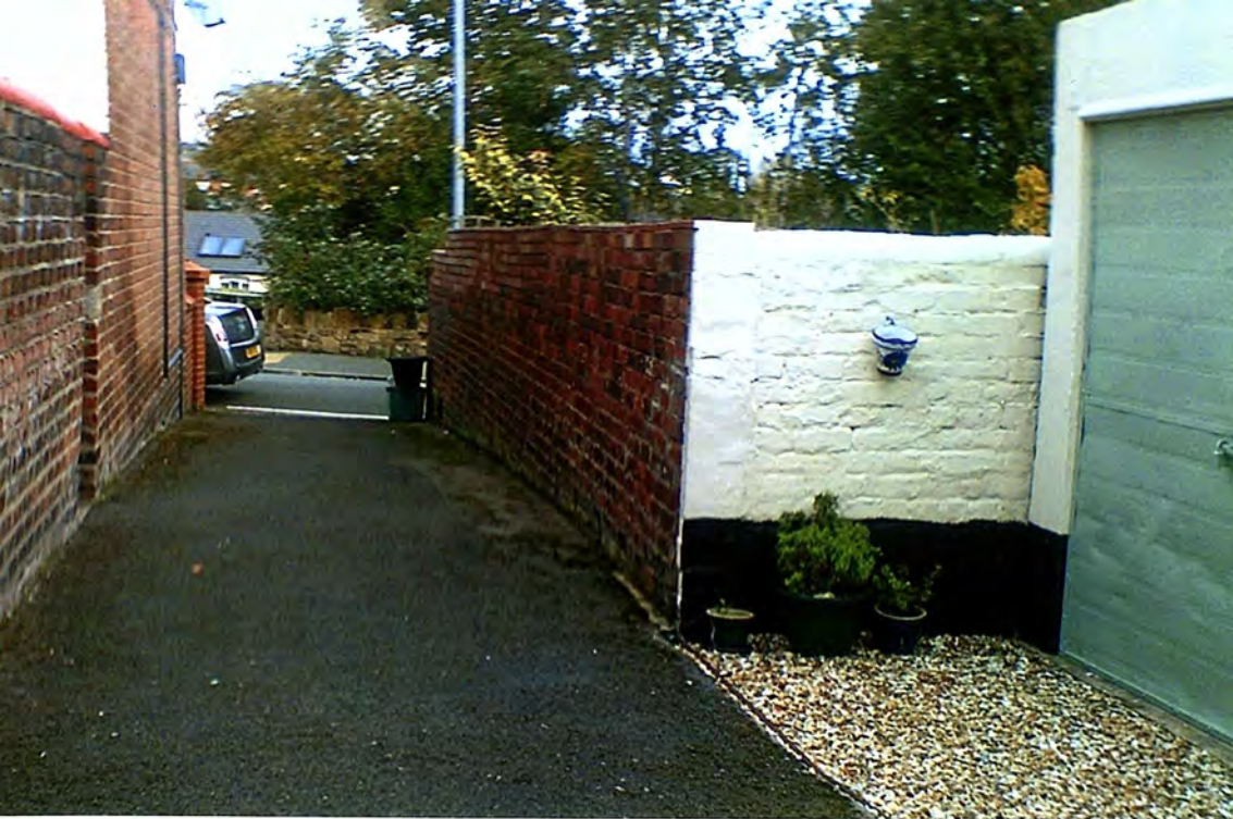
14/10/2017 Rear Access to No.10-No.9-No.8 Albert Street + No.2 Greenbank St.
