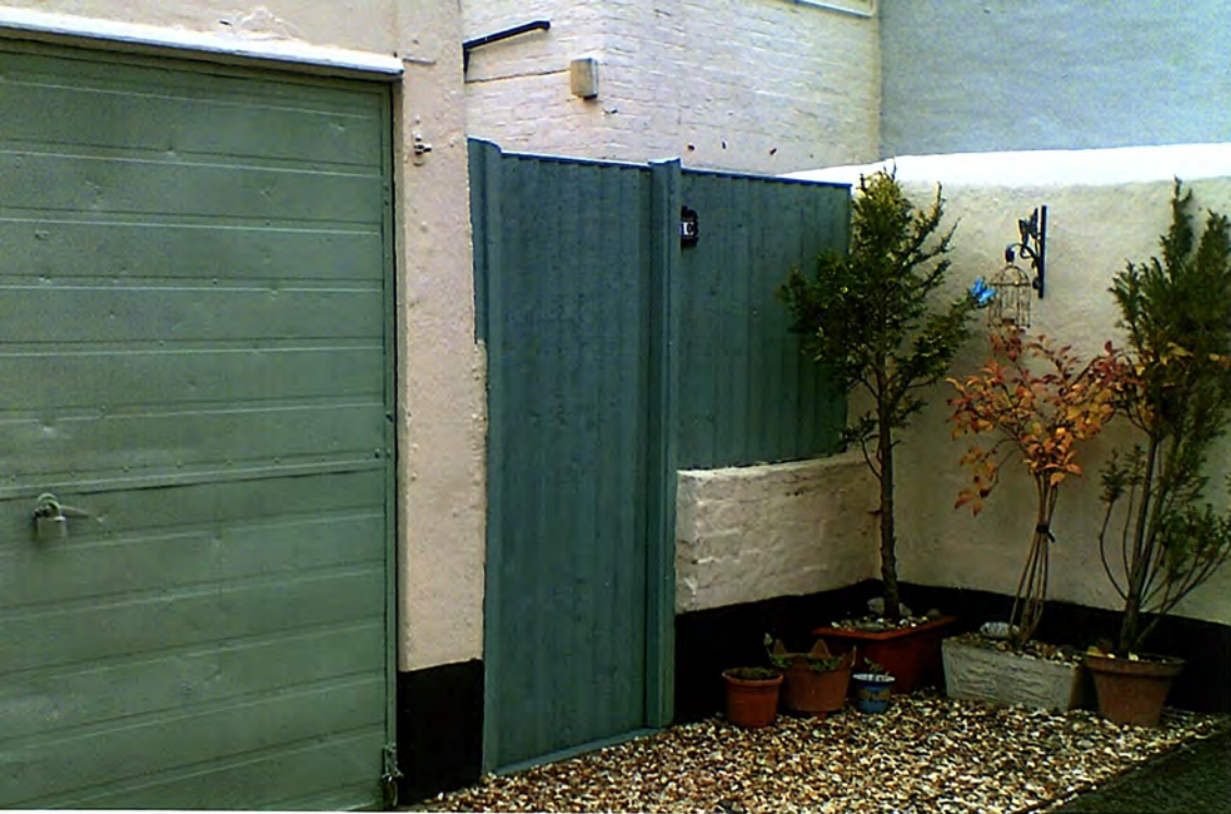
14/10/2017 - No.10 Albert Street (Rear)
