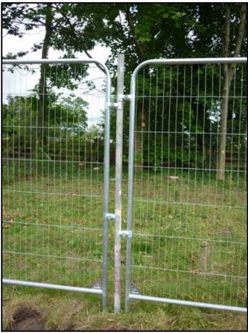
Tree Protective Fencing Specification
