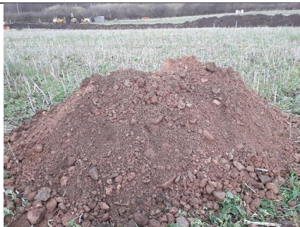
Soakaway Pit 02: Excavation spoil.
