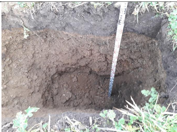
Soakaway Pit 01: Internal view of excavation.
