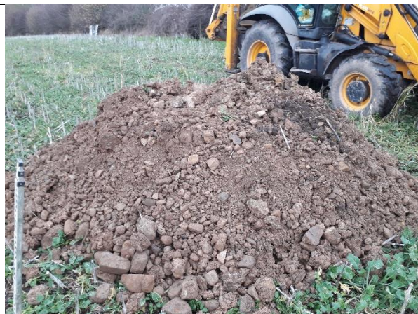
Soakaway Pit 01: Excavation spoil.
