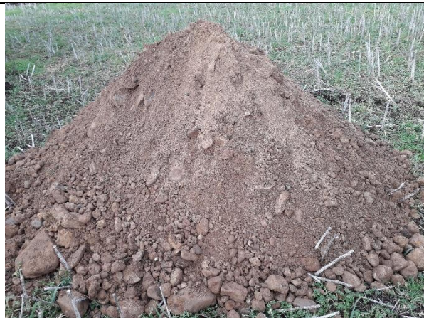
Soakaway Pit 03: Excavation spoil.
