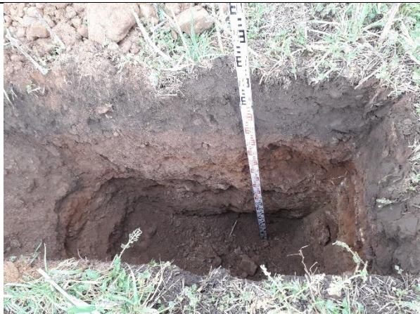
Soakaway Pit 03: Internal view of excavation.
