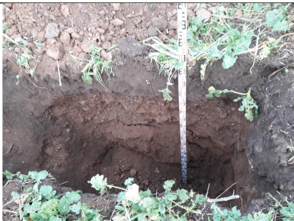
Soakaway Pit 02: Internal view of excavation.
