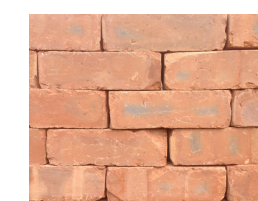
Scotch Common Brickwork
