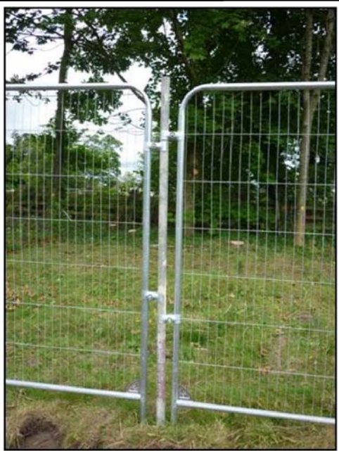
Tree Protective Fencing Specification
