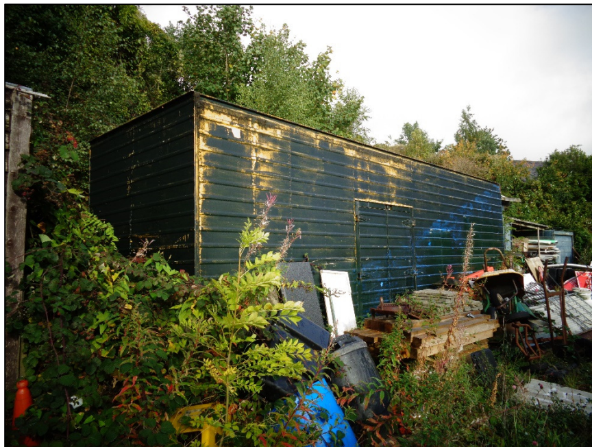
A1.10 Plate 10 – Building/structure 2 (B2)
