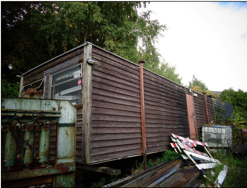
A1.11 Plate 11 – Building/structure 3 (B3)
