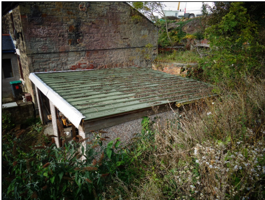
A1.12 Plate 12 – Building/structure 4 (B4)
