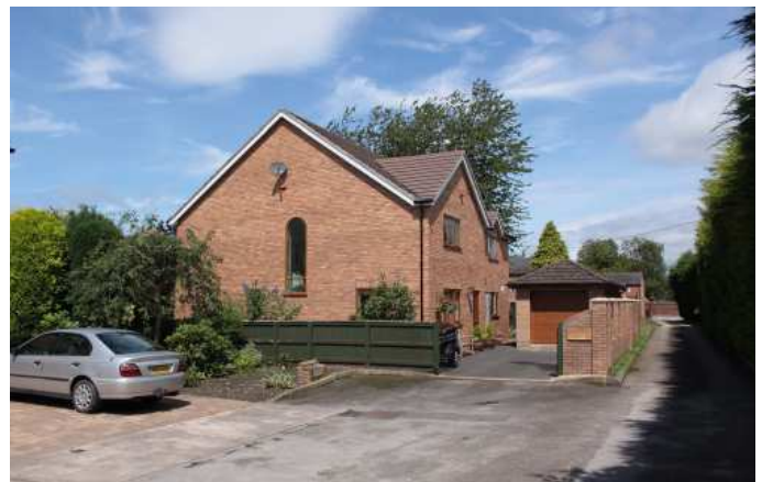
Fig 2.7 - View back along towards the high street. (prior to construction starting)
