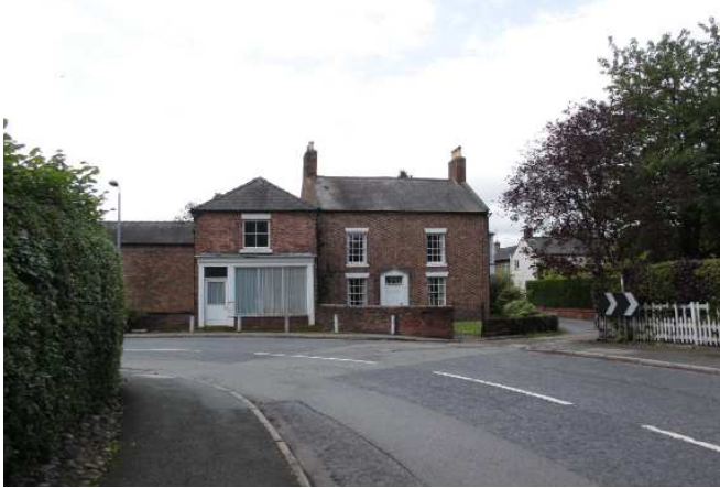
Fig 2.2 - View of Pen Y Llan house from the High Street
