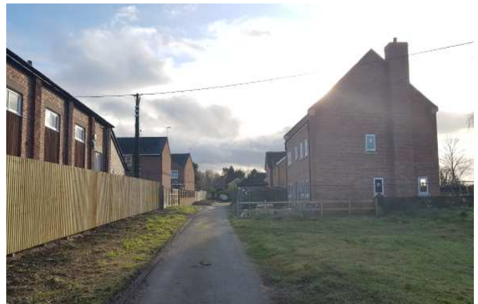
Fig 2.5 - View along existing private road and the Orchards under construction with Library to the left.
