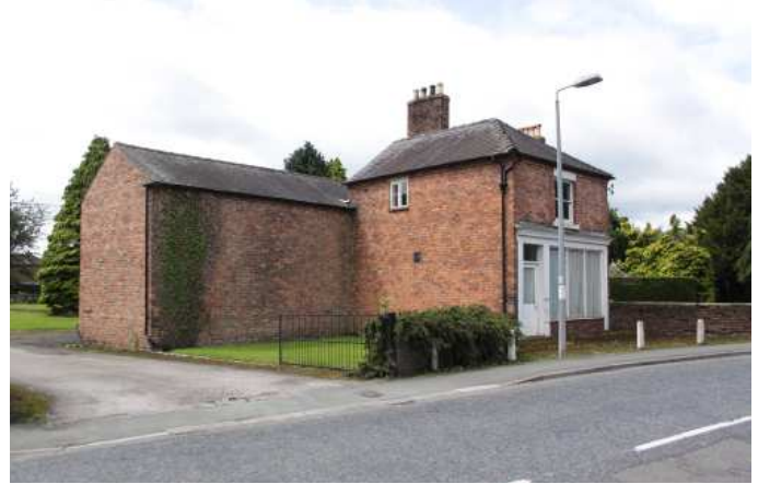
Fig 2.3 - View of Pen Y Llan house and the private road access
