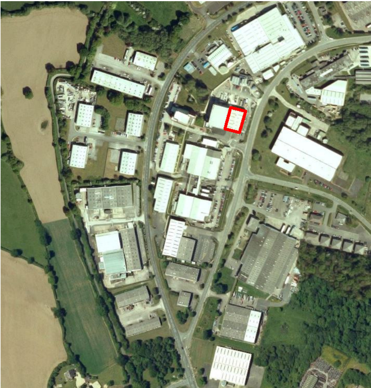
Figure 2 - Aerial view of site – New building outlined in Red
