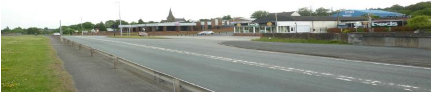
04 View to south of mould road junction
