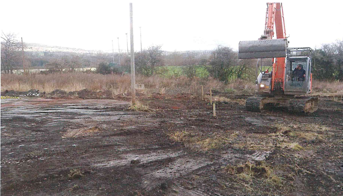
Photograph 9 Overhead and line of gas main
