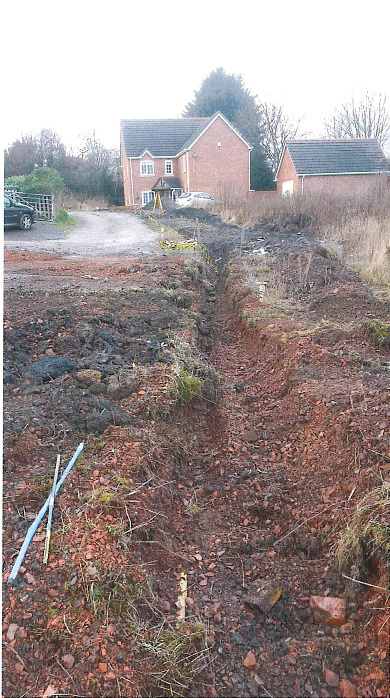
Photograph 11 Line of gas main
