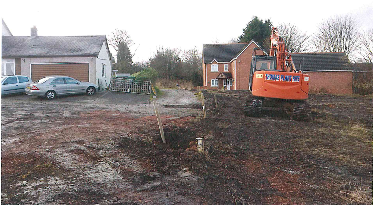
Photograph 5 Line of gas and water main looking west (posts)
