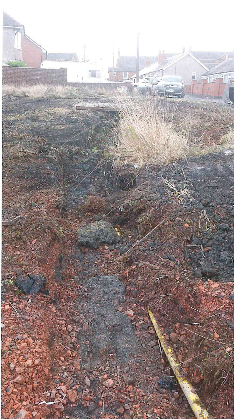
Photograph 12 Line of gas main
