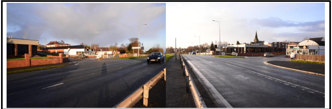
Approach from south and north of the site access.
